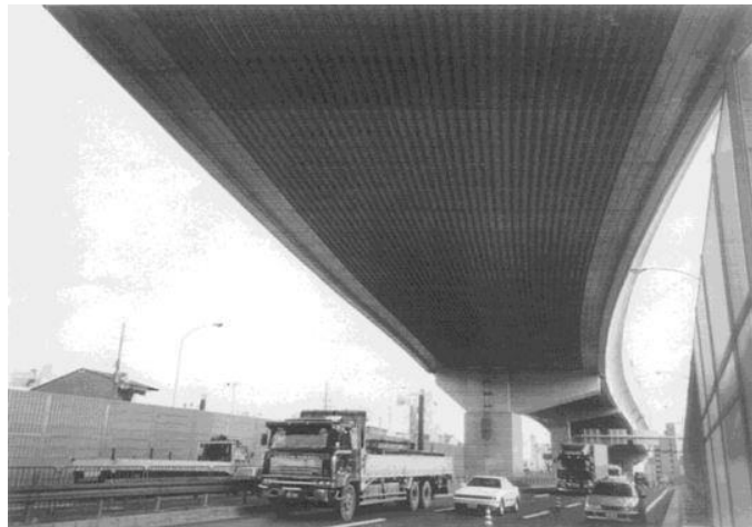
Figure 3. Alporas (Shrinko Wire, Japan) foam being used as a sound management solution on the underside of an elevated motorway. Image sourced from [35].
