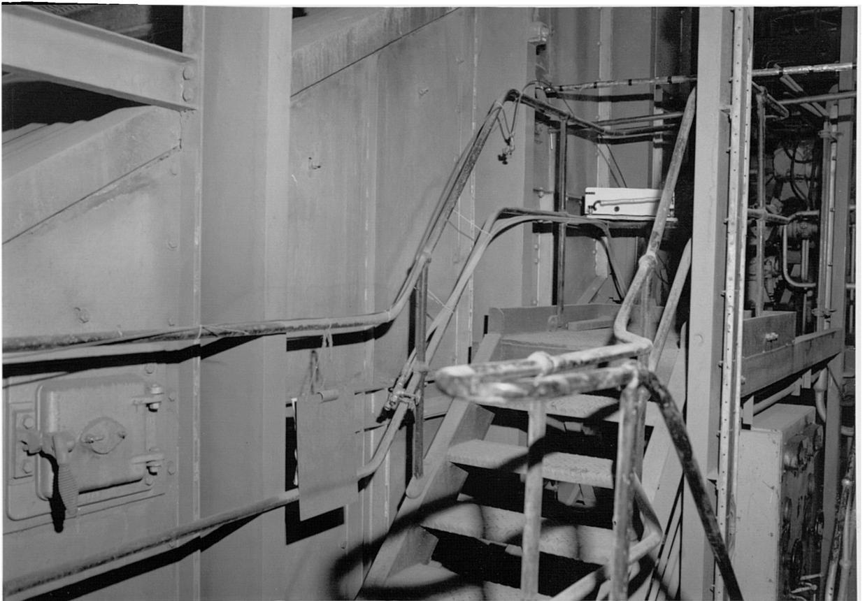
**PLATE 9 - Inside view of the furnace showing location of secondary air openings on the roof arch of the furnace. As shown, most of the openings are blocked.**
