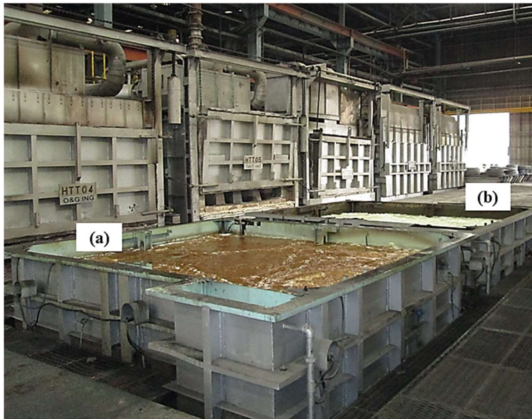
Figure 3-9: Image of the industrial quenching tanks at FRISA: (a) polymer quenching tank and (b) water quenching tank (company archive).
