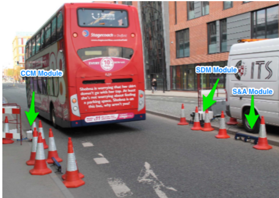
Figure 3.7: Eyre Street installation
