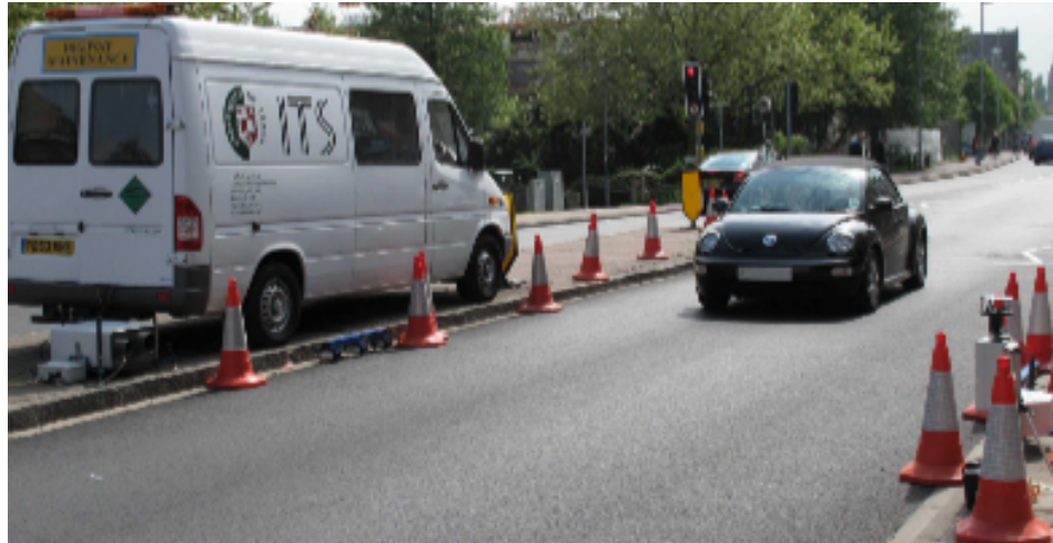
Figure 3.10: East Road installation
