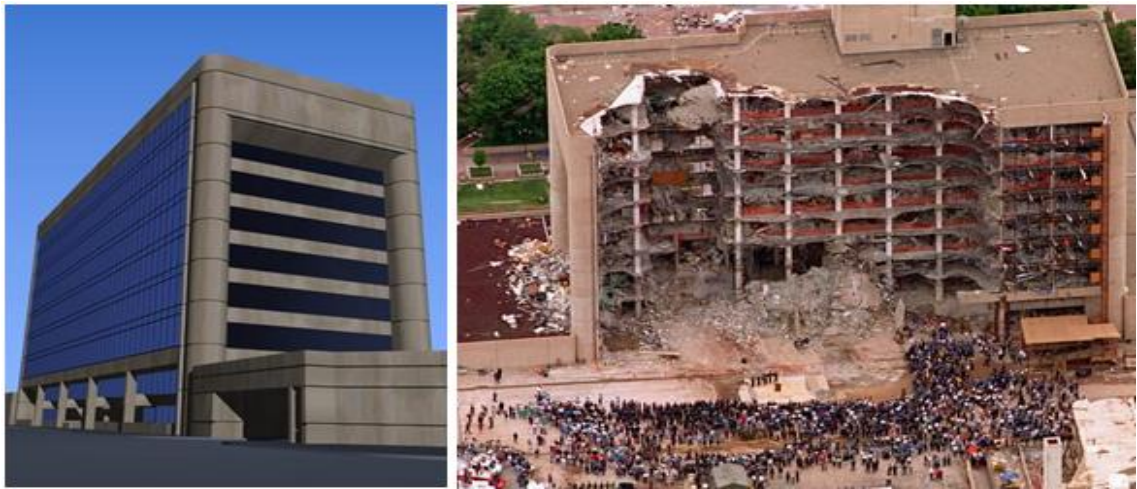
Figure 2-3 Collapse of Alfred Murray Building in United States
