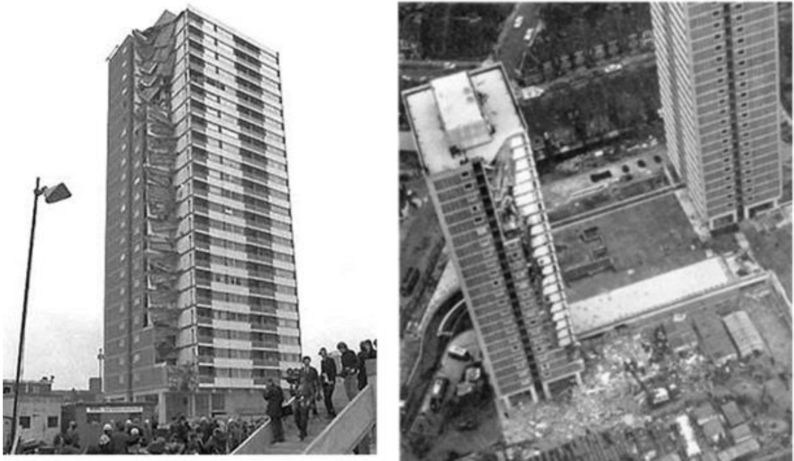
Figure 2-2 Partial collapse of Ronan Point Building (Nair 2006)
