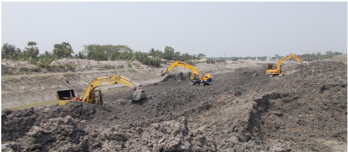
Figure 6: Excavation of Kobadak River in Tala
