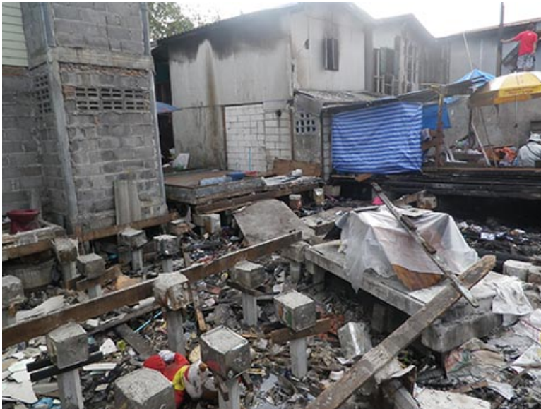
Figure 7.5: Support beam construction methods
