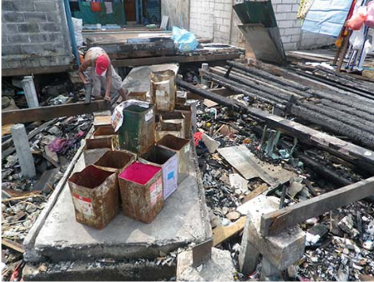
Figure 7.4: Petrol cans waiting to be filled with concrete
