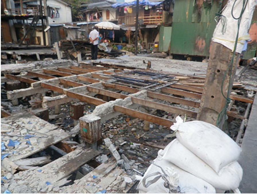
Figure 7.8: Timber support beams to base of dwelling
