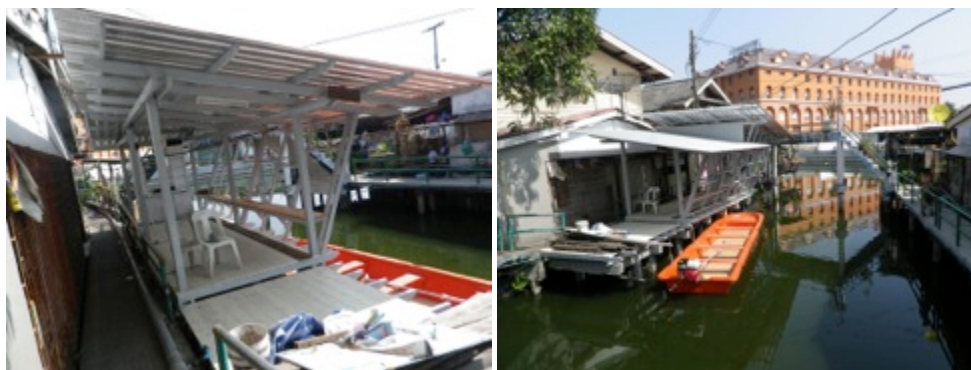
Figures 3.3 and 3.4: Pier intervention in an informal settlement, Bangkok.
