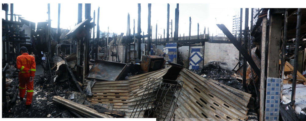
Figure 3.18: Devastation two days after the fire, Rom Klao
