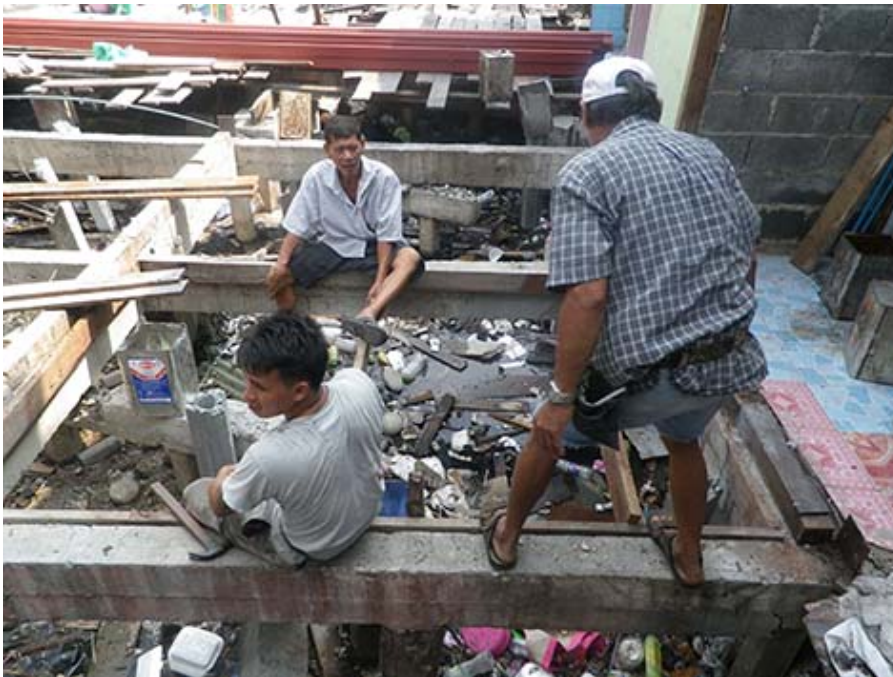
Figure 7.6-7.7: Support beam construction methods
