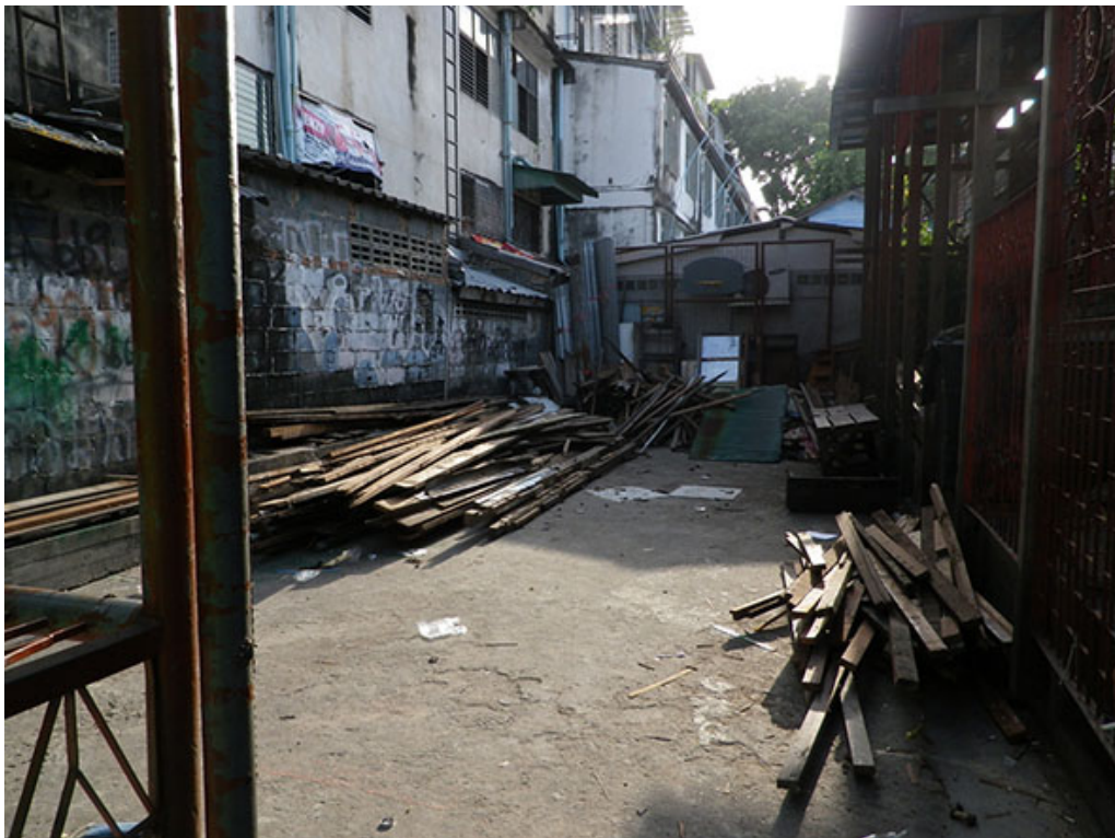
Figure 6.11: Timber being stored in Community Lantern, Lok 1-2-3
