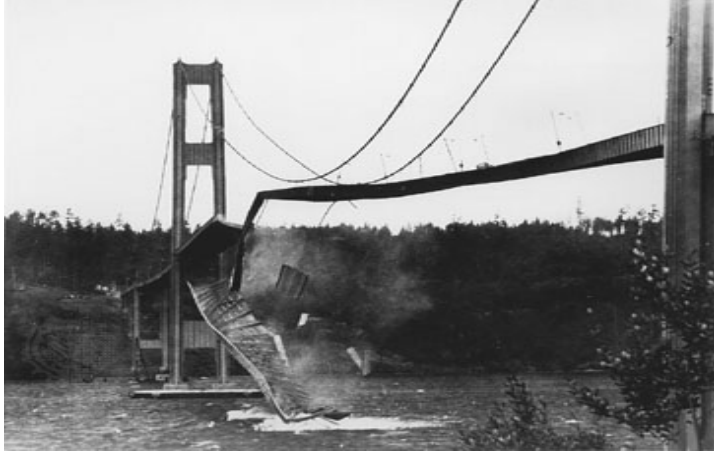
Fig. 1.1 Tacoma narrows suspension bridge 1
