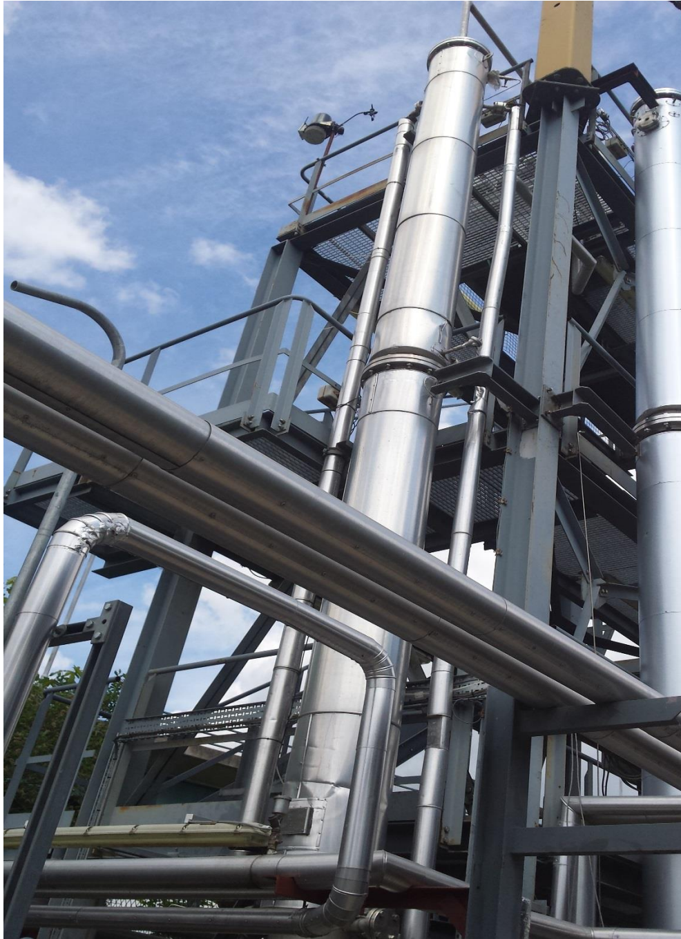
(a): The wind sensors clamped on a mast at the PACT site, Beighton.
