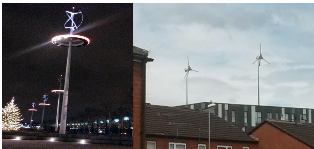
Figure 2. 8: An example of VAWT and HAWT applications within a built environment in UK.
