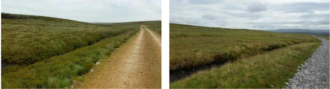
**Figure 4.9** Stone tracks with drainage channels running parallel to the track on the upslope side.
