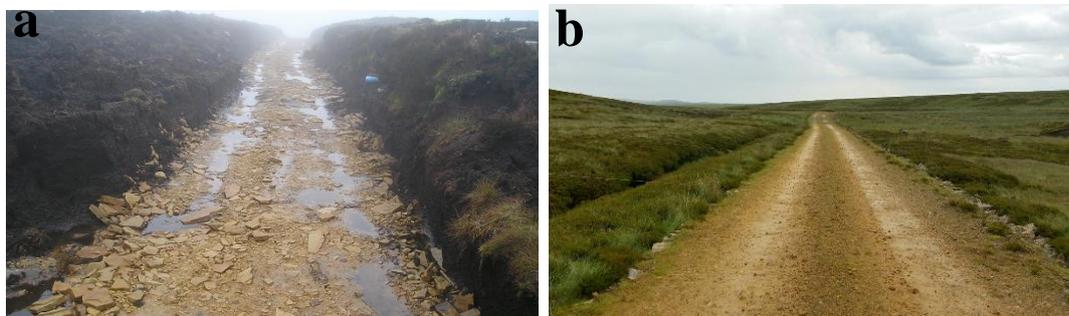
**Figure 2.3 a-b** a) Example of a ‘cut and fill’ road where the peat has been excavated and aggregate placed along the base of the trench to form the travelling surface. Photo Courtesy of North Pennines AONB. b) Example of floating road on blanket peat where the aggregate is placed on top of the peat surface.
