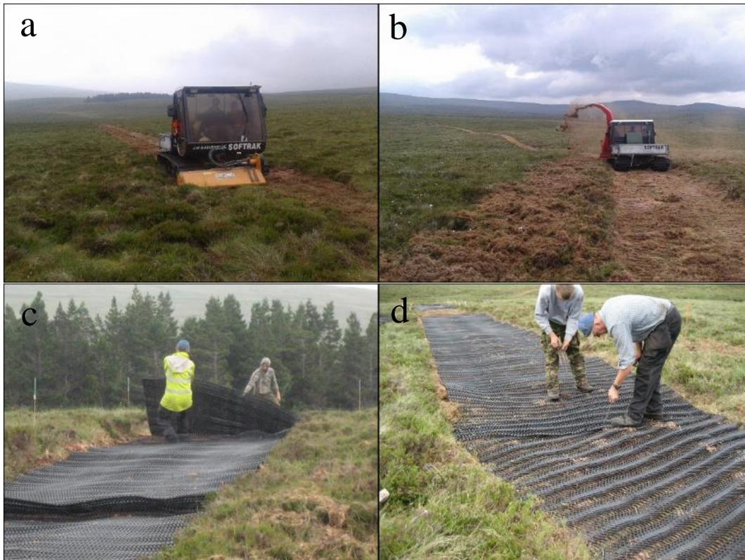
**Figure 3.8 a-d** a) Cutting of track route using a SOFTRAK with mower attachments, b) Removal of excess cut vegetation along track route using the SOFTRAK with forager attachment, c) Positioning of plastic mesh along route, and d) pinning of track route into place. Photos a) and b) courtesy of Alistair Lockett (North Pennines AONB Partnership).
