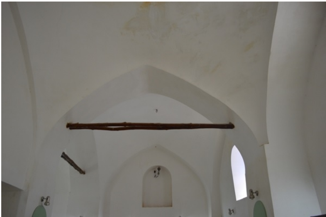
Figure 6.25 Wooden trusses at Khan Al-Shiln .
