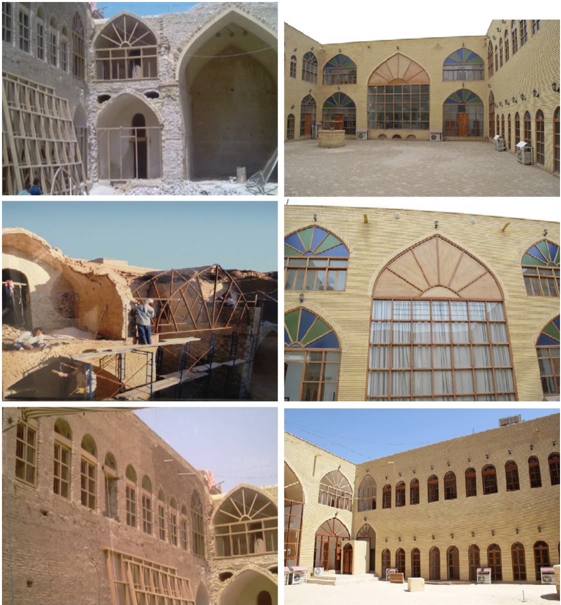
Figure 6.31 Rehabilitation work on Khan Al-Shilan ; (source: The Khan Al-Shilan museum).
