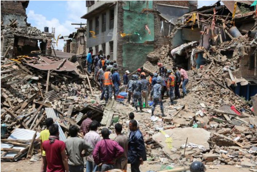
Figure 2.1: Partially and fully collapsed sections of buildings after the 2015 Nepal earthquake. Fully collapsed areas are very difficult to explore and partially collapsed areas can be structurally unstable and thus unsafe (image reproduced from [49] under the Creative Commons license).
