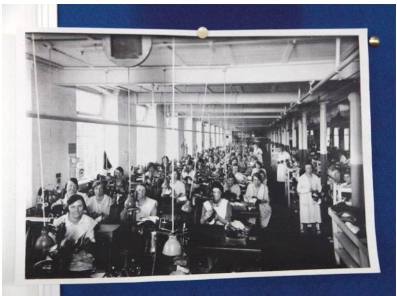
Fig. 6.5: A photograph of the same office when it was a factory. Date unknown.
