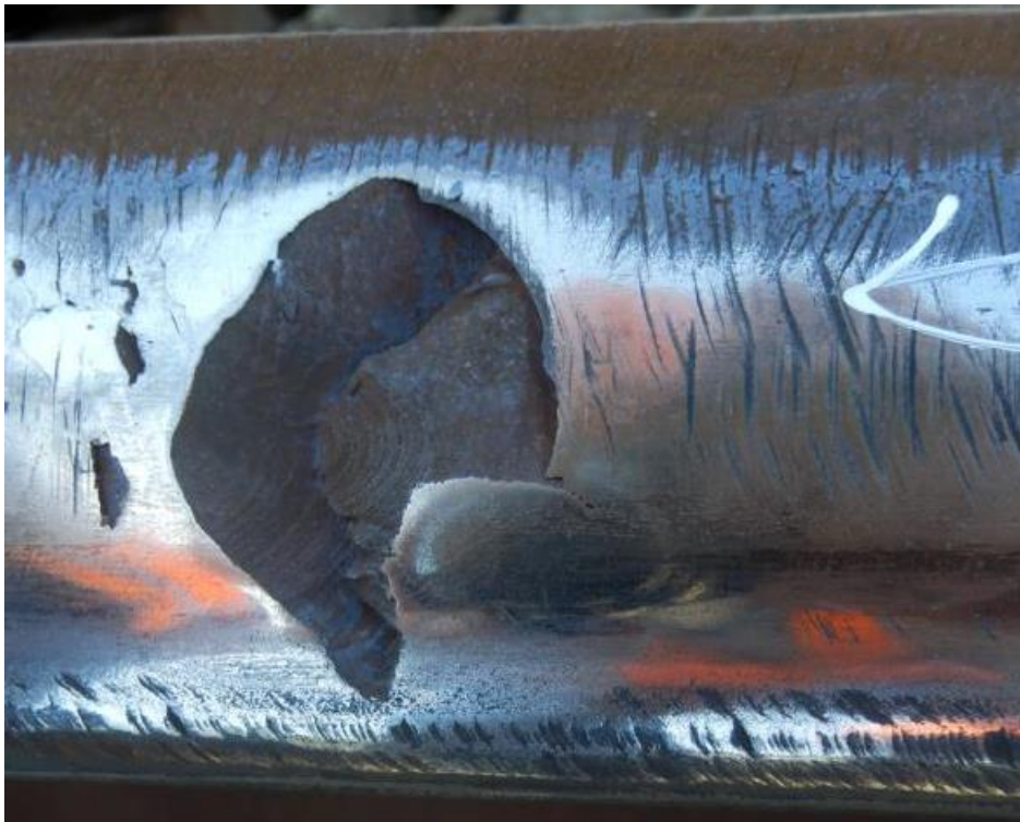
Figure 3-21 Squat type defect that has spalled out (delamination of rail surface) [4].
