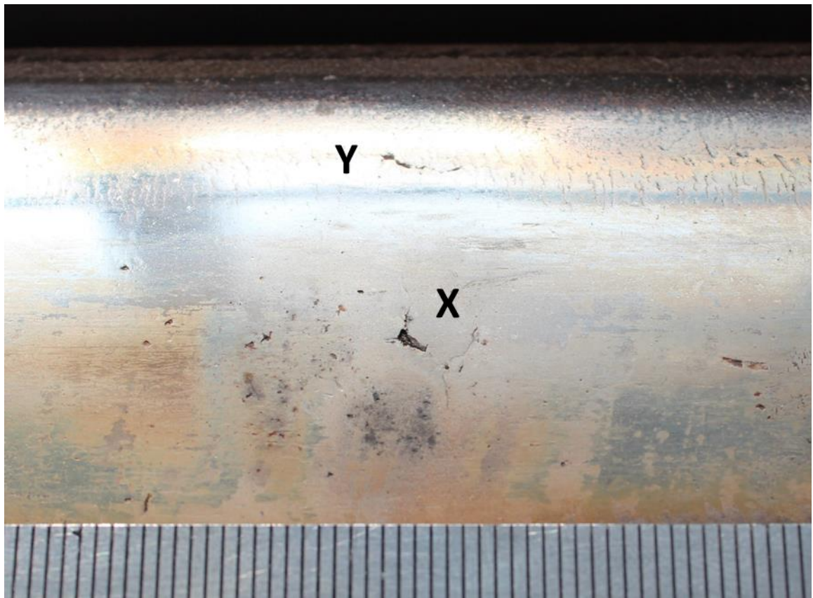
Figure 3-2 Detail observation of defect A. X and Y denotes crack mouth
