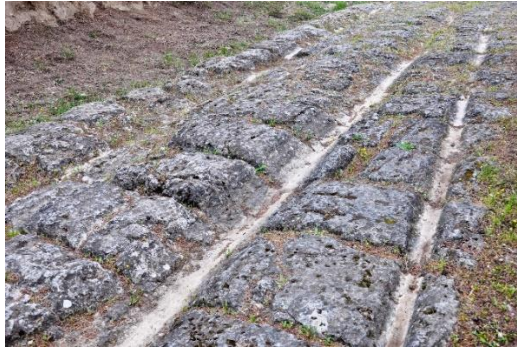
Figure 2-1 Paved track/ruts that guide the wheel so that the vehicle will remain on the track near Corinth, Greece [123].
