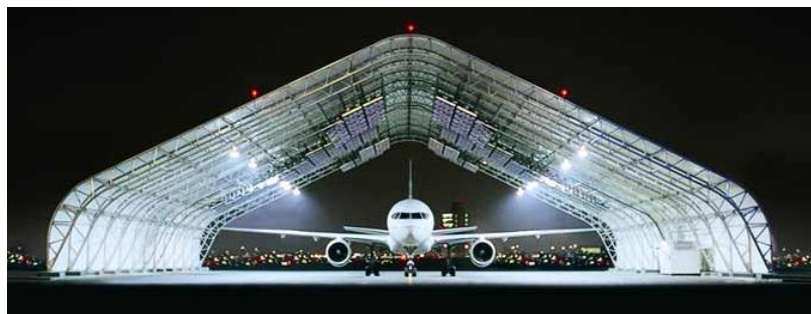
Figure 1.10 Infrared hangar structure for de-icing
