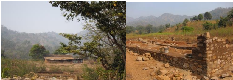
Figure 8 Traditional 'kachcha' homes in Amba, built from forest materials and mud The commencement of the building of a 'pukka' home in Amba, under a social welfare scheme.
