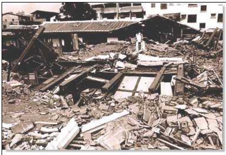
Fig. 5.8 The Lin Family mansion and garden in Wufen township after the earthquake in 1999. (Source: National United University, no date; Accessed Oct. 1, 2016, < http://web.nuu.edu.tw/~flhuang/921/a065.html >)
