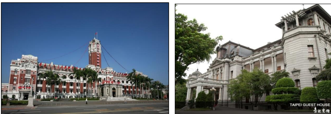
Fig. 3.14 Official buildings - legacies of the Japanese colonial period. (Source: Office of the President, no date; Accessed Oct. 1, 2016 < http://www.president.gov.tw/Default.aspx?tabid=1202 >; Taipei Guest House, no date, 2012; Accessed Oct. 1, 2016 < http://www.mofa.gov.tw/tgh/cp.aspx?n=4F8ED5441E33EA7B >)
