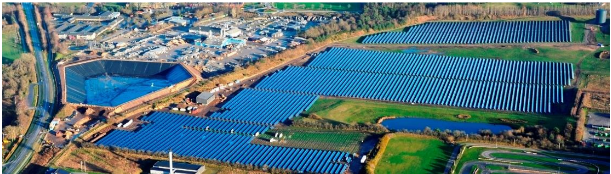
Figure 2-36: Vojens 70,000m 2 solar thermal array and 200,000m 3 pit thermal store. Source : State of Green (2016).
