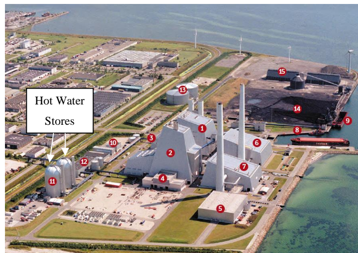
Figure 1-3: Two 22,000m 3 hot water stores at a CHP plant linked to district heating in Copenhagen. Source: DONG Energy (n.d.).
