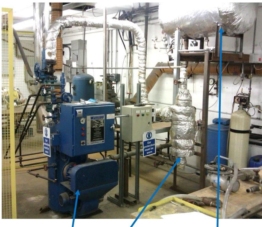
Figure 5-3: *Wanson Vaporax II* steam generator, with steam separator and feed water tank
