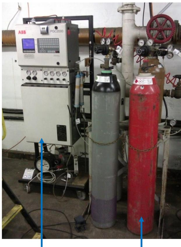
Figure 5-20: The ABB PGC2000 gas chromatograph and carrier gas cylinders
