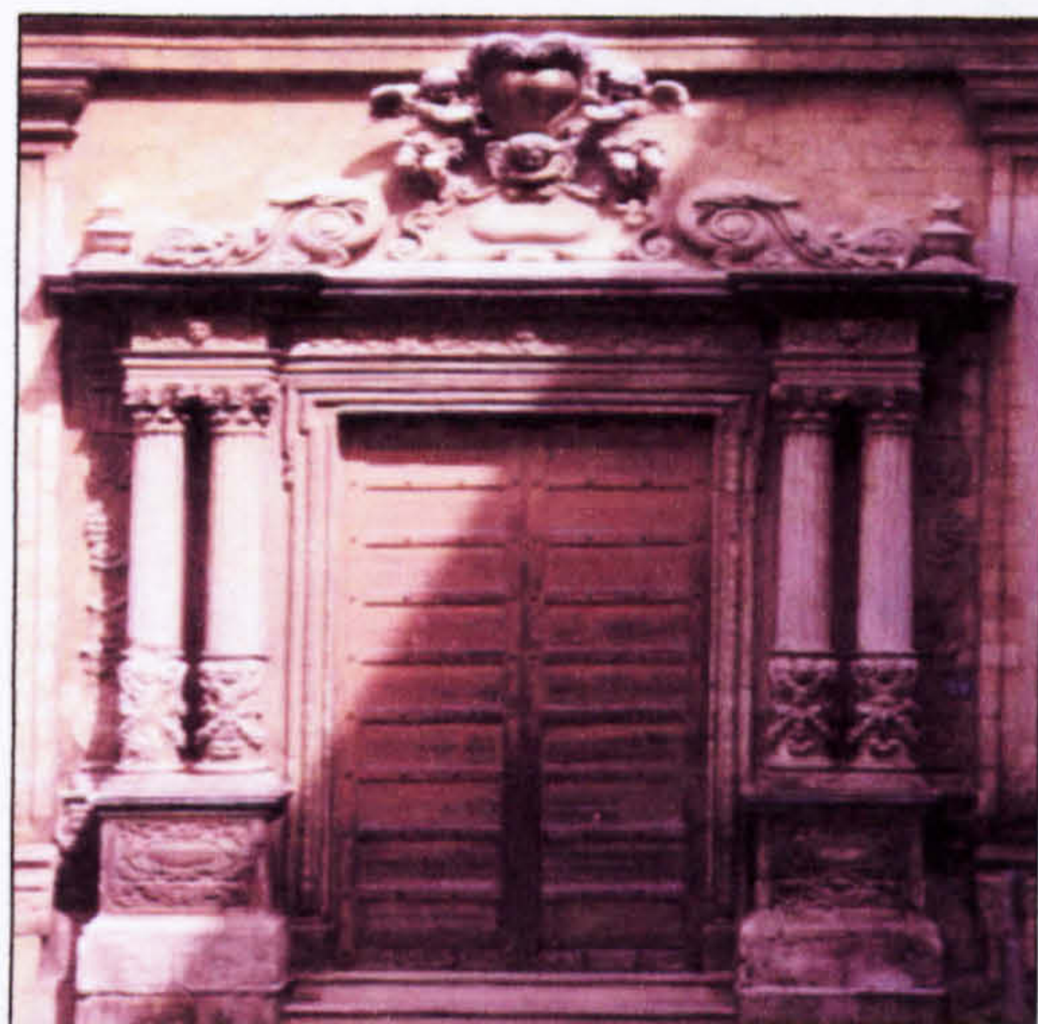
Figure 5.108: Entrance to the church of Chiesa del Gesu, Palermon, Sicilly (photo by S. Di Maria)
