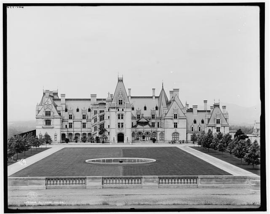
Fig. 13. William Henry Jackson, Biltmore House , c. 1902. Photograph. Library of Congress Prints and Photographs Division, Washington D.C.
