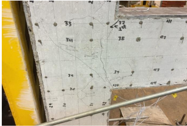
Photo 4-21: Crack formation in the SCS under cyclic load
