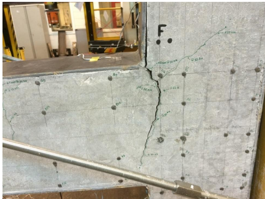
Photo 5-12: Cracking in the DSC with HSC – test
