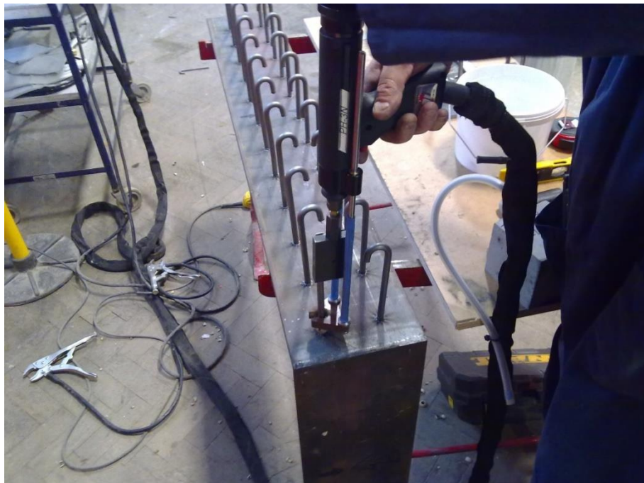
Photo 3-3: J-hooked connector welding
