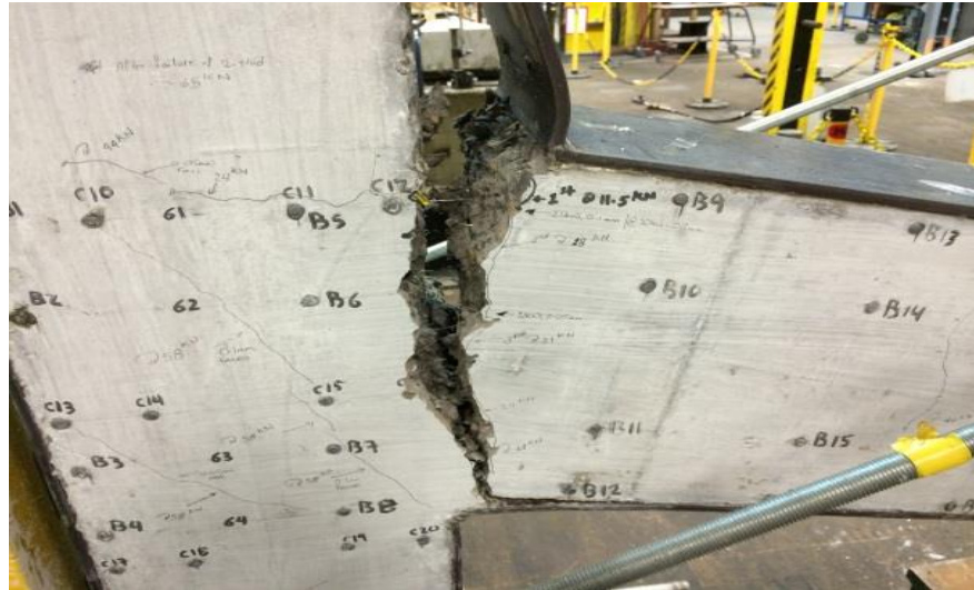
Photo 4-15: Failure of the SCS joint with SF 0.25%
