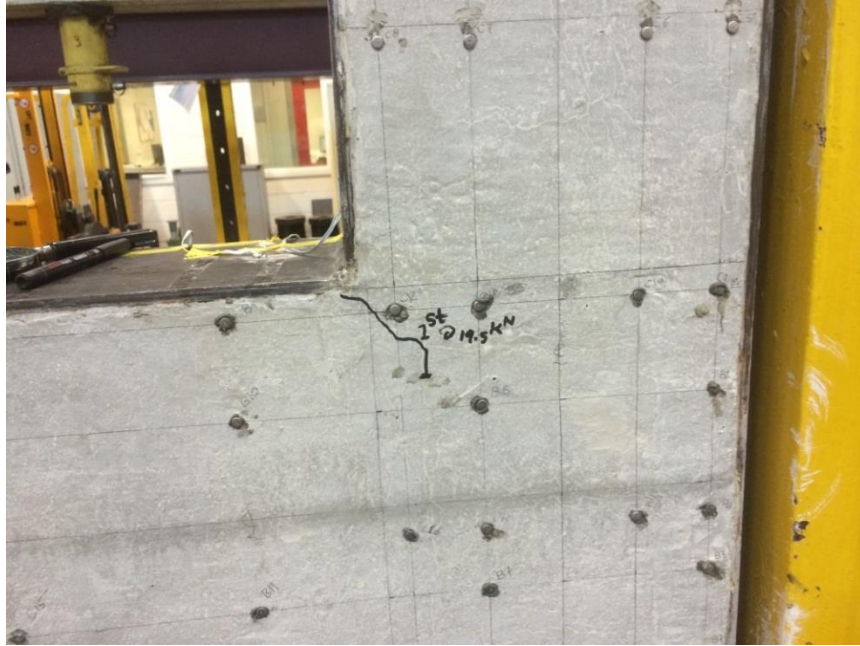
Photo 4-16: First crack formation in the SCS joint with SF
