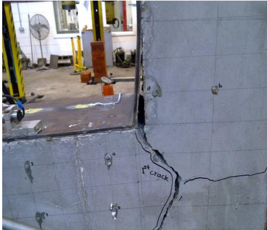
Photo 4-3: Final failure in the SCS joint – basic design
