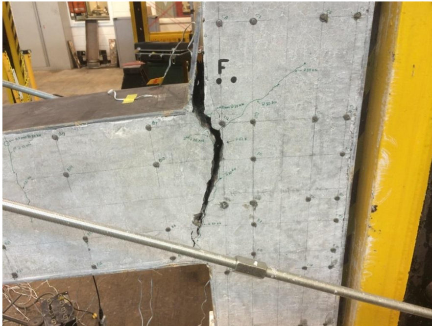
Photo 4-13: Failure of the SCS joint with HSC
