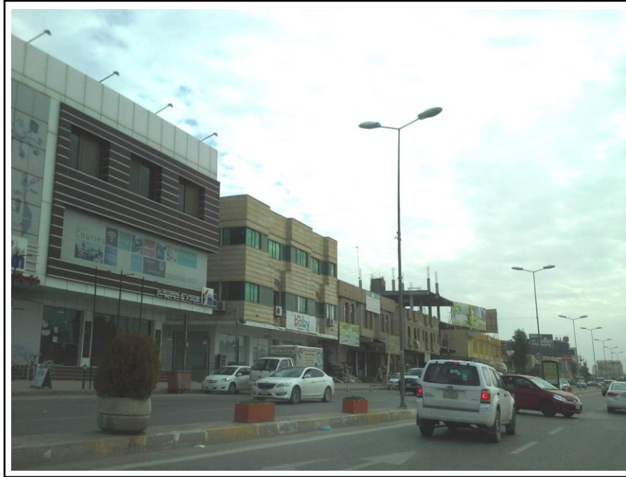
Figure 4.119: Demolition the old houses located on the radial road (Runaky Road) and replacing them by multistorey commercial buildings. (Source: Researcher)
