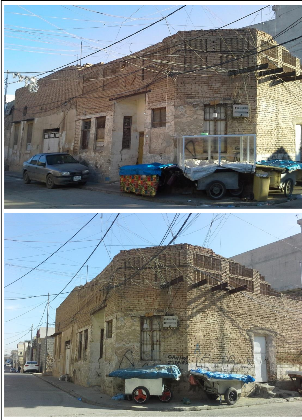
Figure 4.43: ‘I–section steel joists’ used for windows and doors lintels and roofing in an early single-family house in the area of ‘Sample 2’. It superseded the use of timber which was in use prior to 1920. (Source: Researcher)
