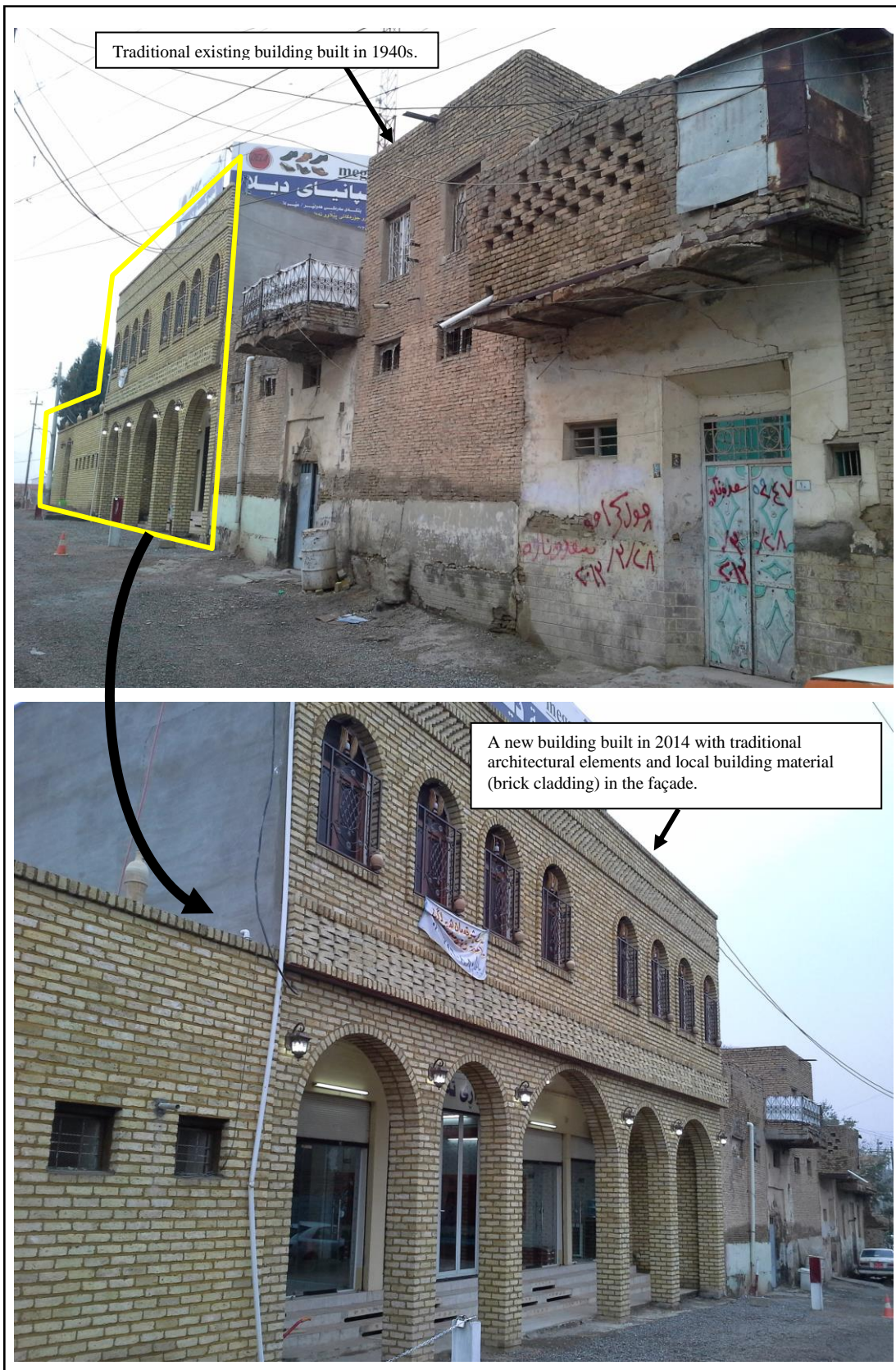
Figure 4.28: The influence of the proposed urban design guidelines for the ‘buffer zone A’ of the citadel. A new building in the area built adjacent to a traditional building according to the regulations that achieve harmonizing the facades. (Source: Researcher)
