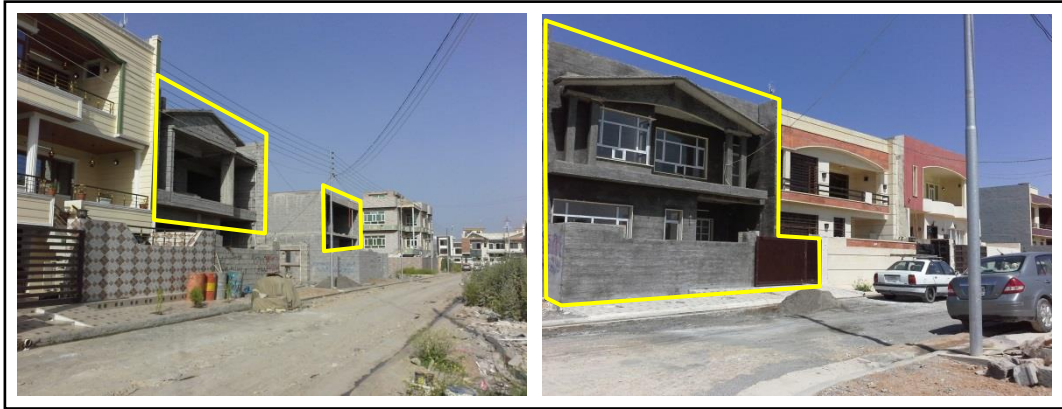
Figure 4.197: Incomplete houses beside completed houses. (Source: Researcher)
