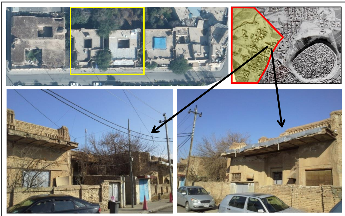
Figure 4.75: Early courtyard houses in the northeast part of the ‘Minara’ quarter built in the late of the second period (1937-1940). (Source: Researcher)
