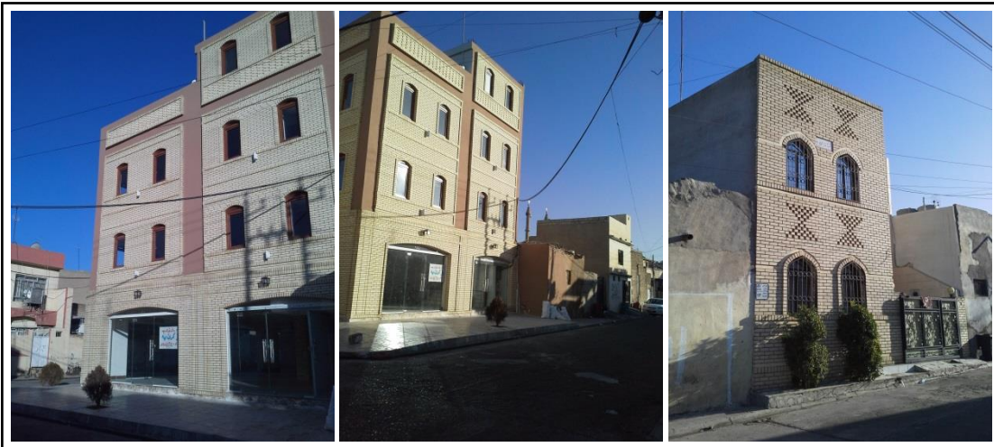
Figure 4.60: New buildings in the area built according to the 'Citadel Buffer Zone Guidelines of 2011'. The maximum height allowed is 4 floors. Setback distance from the streets is applied on some zones in the area basing on their previous regulations. The facades are flat with decorated brick cladding and windows with flat and pointed arches to reflect the heritage and vernacular elements. However, the attached type has been maintained. (Source: Researcher)
