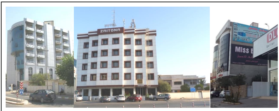
Figure 3.11: Single-family houses adjacent to multi-storey buildings. (Source: Photographs by the researcher, 2011)
