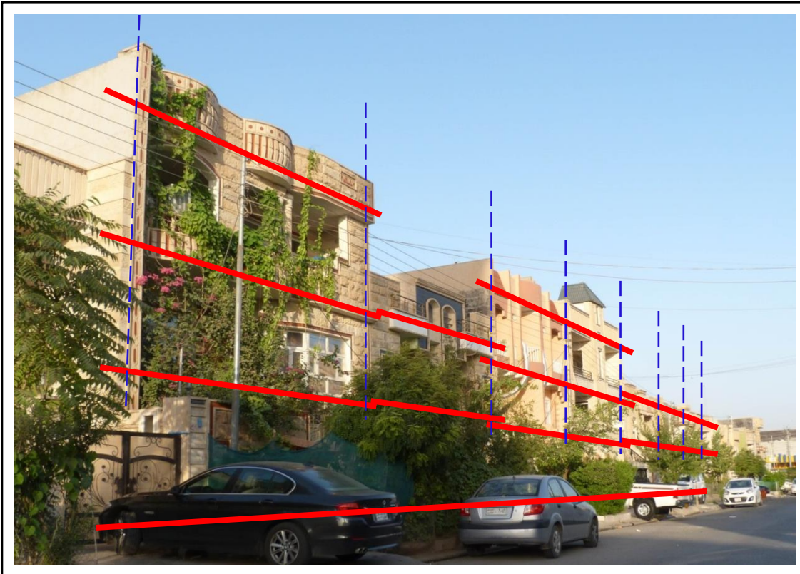
Figure 3.17: Attached houses with two and three floors in one block. (Source: Researcher)
