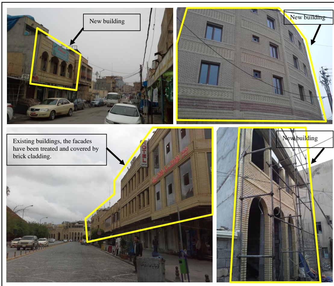
Figure 4.32: New and existing buildings that have façade treatment with brick as a local and vernacular building material. (Source: Researcher)
