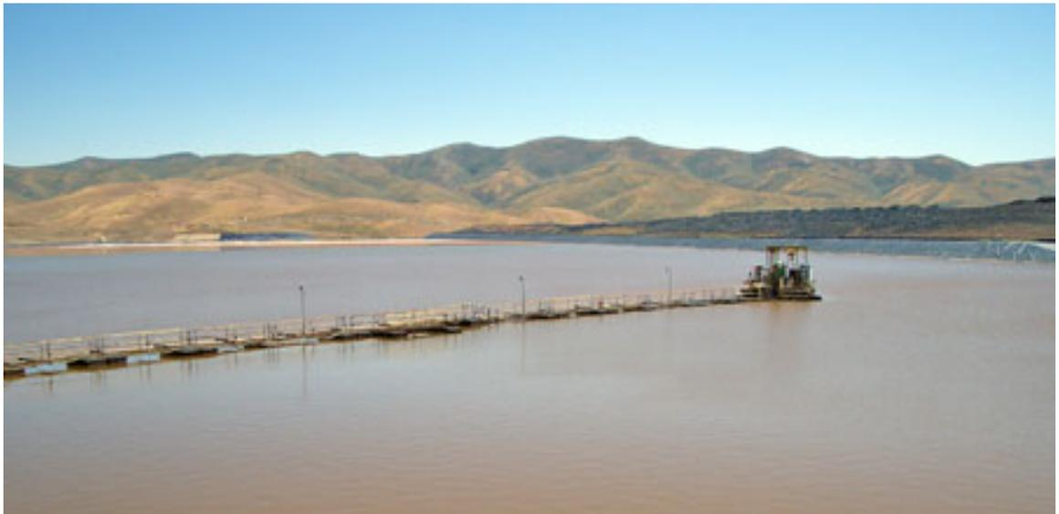
**Figure 1.4:** Example of a conventional impoundment technique to store mine waste in mining areas. Picture reproduced from Engels [18].
