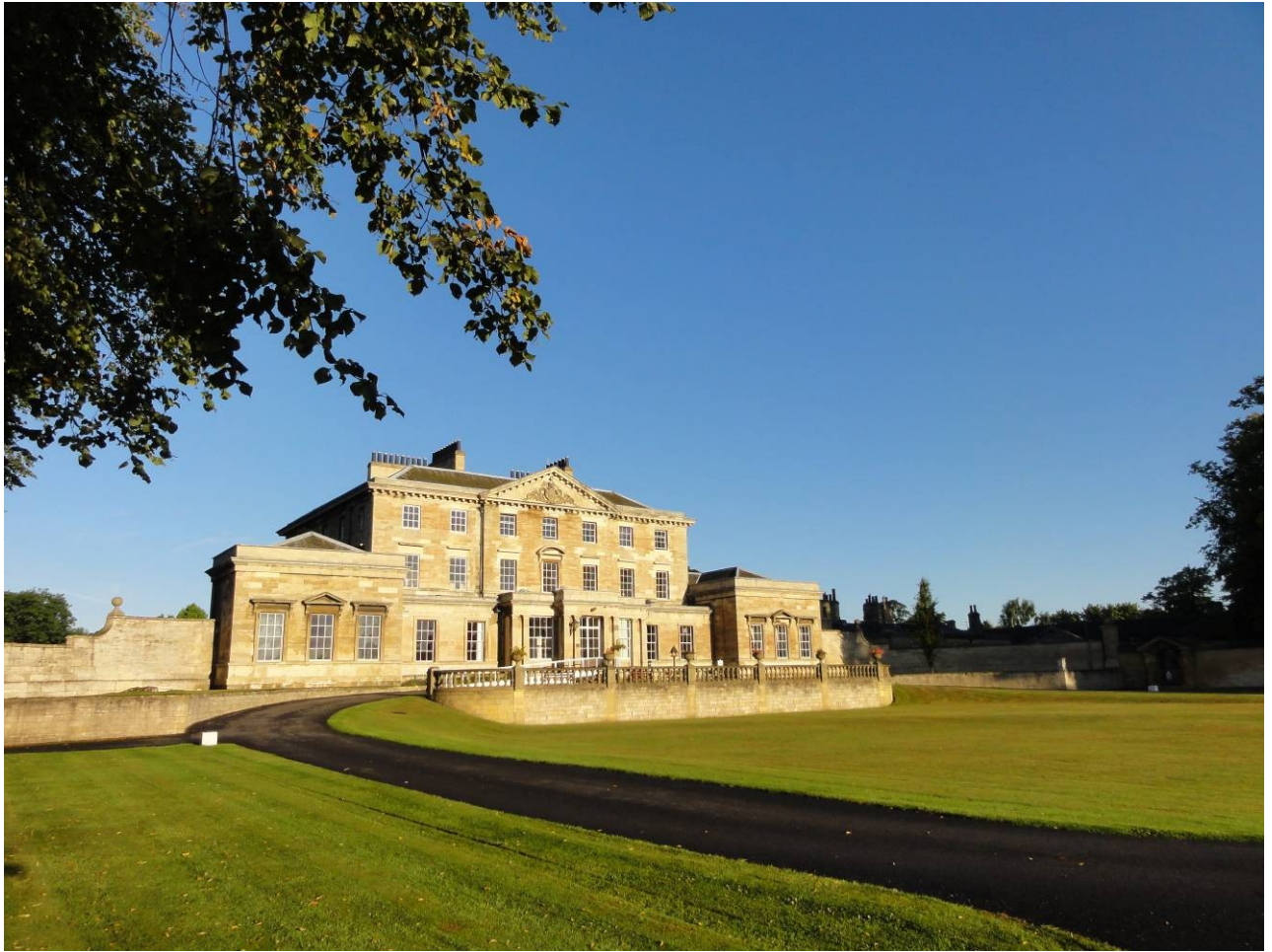
Figure 4.18: The imposing east facing Palladian style facade of Hickleton Hall. Source: author
