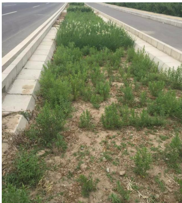
Fig. 2.30. Planting failure caused by inappropriate plant selection in a series of highway rain gardens. The failed vegetated zone was occupied with native weeds. Xi'an China. Photo was taken by the author in June 2014.
