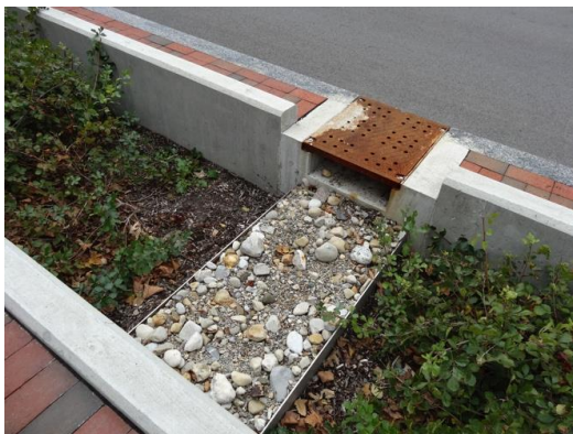
Fig. 2.33. Poorly managed vegetation in a street rain garden, Columbus, USA. Photo was taken by the author in October 2012.
