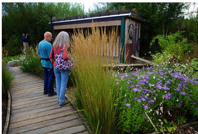
Fig. 2.4 Typical rain garden systems used to treat runoff diverted from a building roof and surrounding surfaces in London Wetland Centre, London, UK. Photo was taken by the author in
