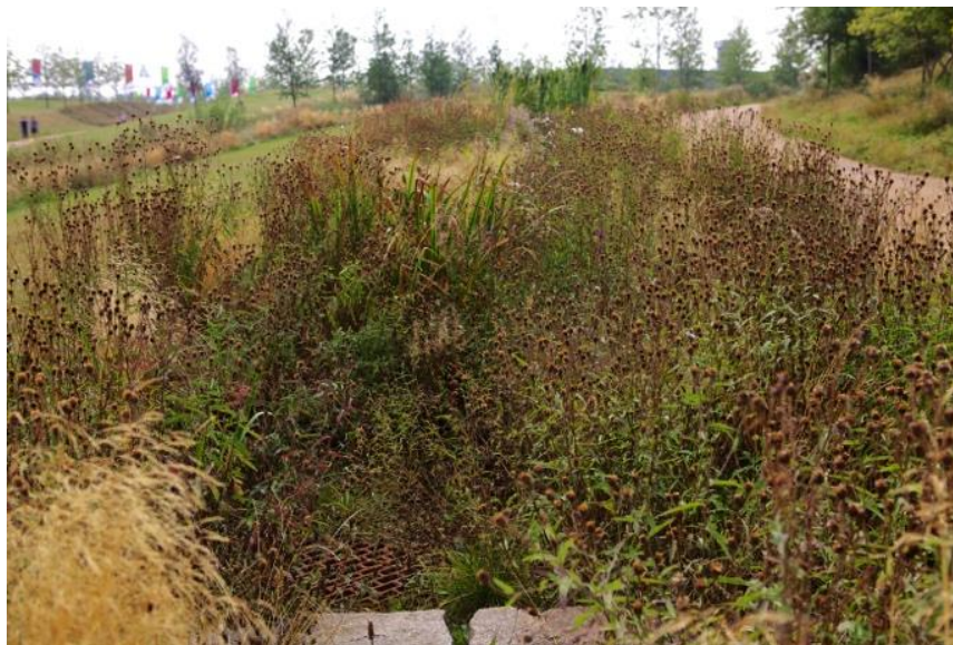
Fig. 2.19. Public drain inlet placed on the marginal area of rain garden to quickly drain the excess surface runoff, London 2012 Olympic Park, London, UK. Photo was taken by the author in August 2013.
