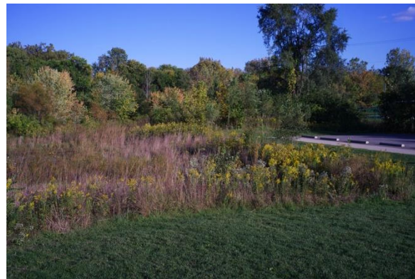
Fig. 2.12. Typical filter basin with dense planting, Olentangy River Wetland Research Park, Columbus, USA. Photo was taken by the author in September 2012.
