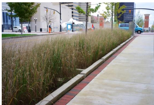
Fig. 5.2. Rain gardens installed alongside city road, which featured monoculture of native grasses, Columbus, USA. Photo was taken by the author in October 2012.
