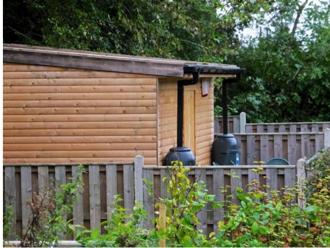
Fig. 2.14. Runoff harvesting barrels fitted with roof gutter in Manor community, Sheffield, UK.
