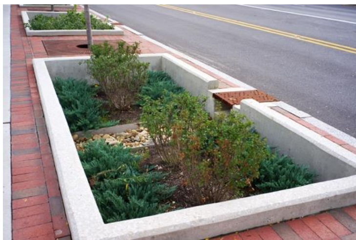
Fig. 2.18. Rain garden used to infiltrate highway runoff, Columbus, USA. Photo was taken by the author in October 2012.
