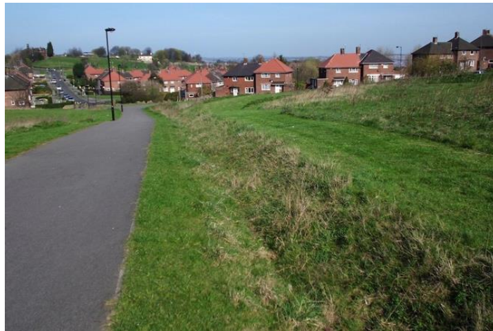
Fig. 2.32. Bioswale featuring sown turf mixes with low plant diversity and poor aesthetics, Sheffield, UK. Photo was taken by the author in May 2012.
