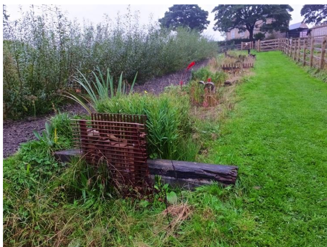
Fig. 2.10. Bio-swale conveying and infiltrating runoff from an upland allotment to downstream watershed, Sheffield, UK. Photo was taken by the author in October 2013)
