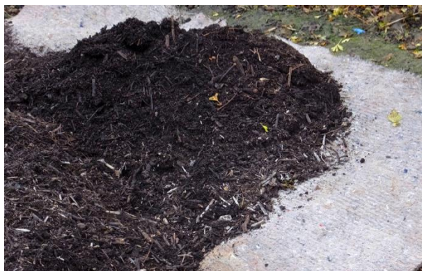
Fig. 5.28. Spreading green waste compost on the top of the felt mat laid on the existing soil. Photo was taken by the author in December 2013.
