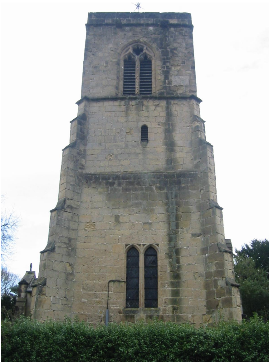
Fig. 64. St Mary, Little Driffield from the west.
