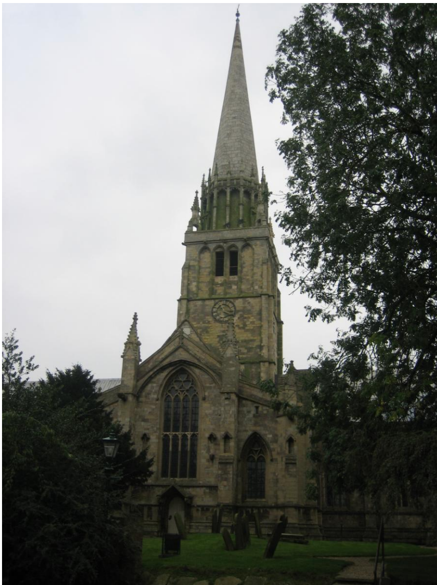
Fig. 192. St Patrick, Patrington from the north.
