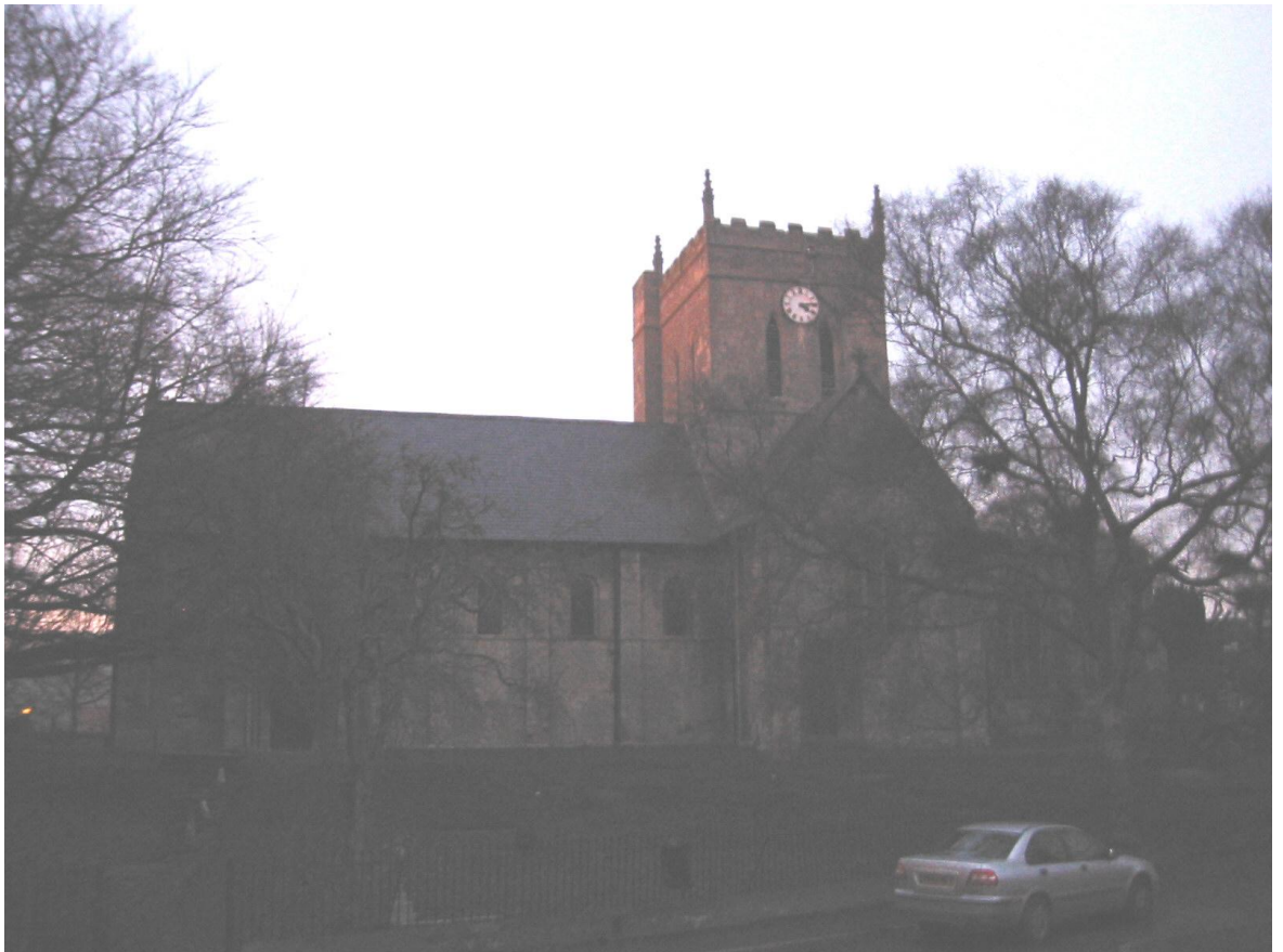
Fig. 48. The Church of St Nicholas, North Newbald from the south-west.
