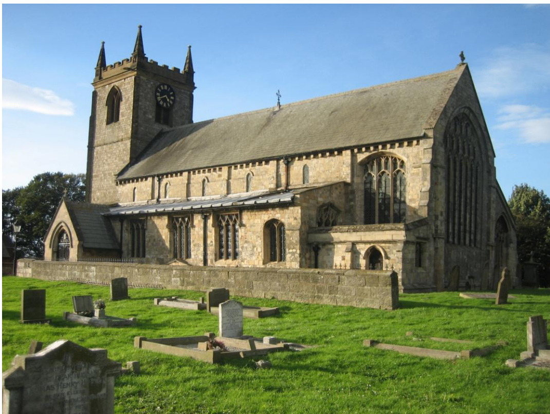
Fig. 111. St Mary, Swine from the south-east.
