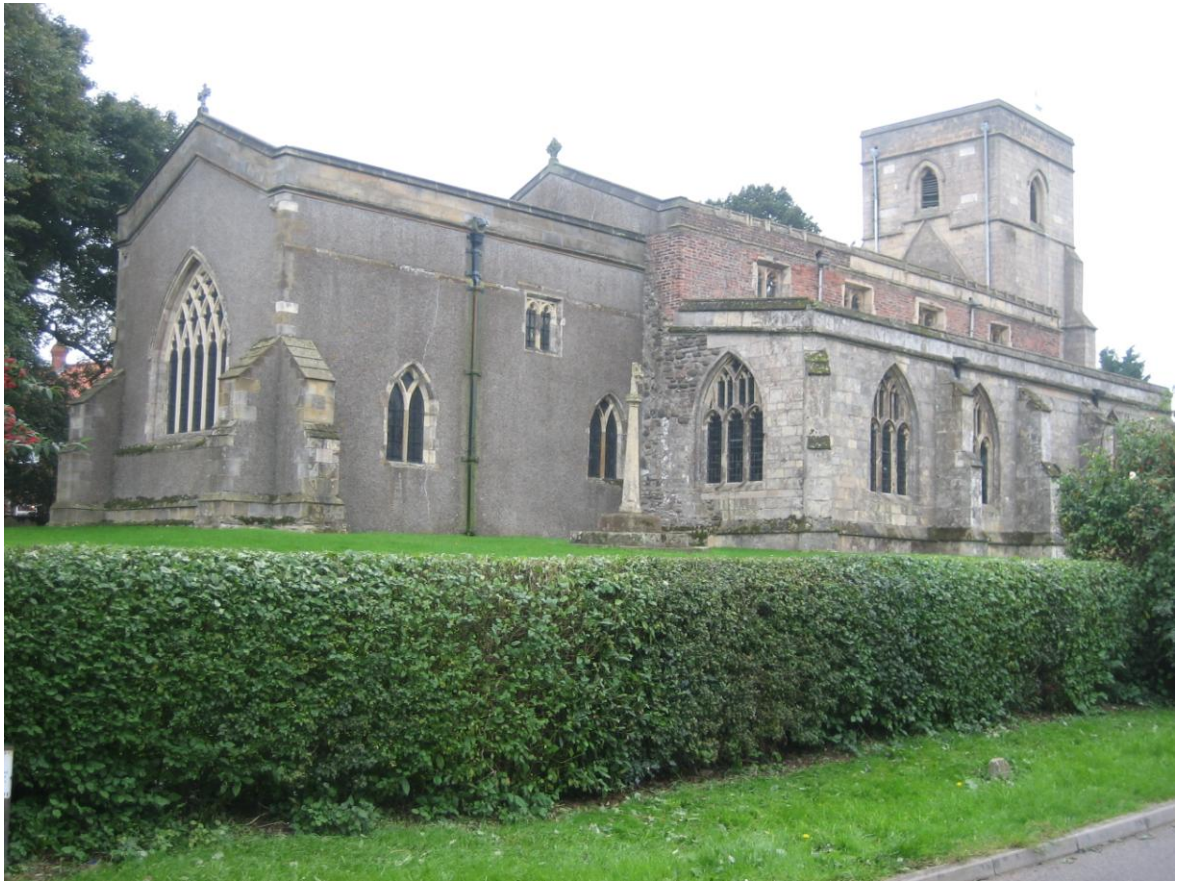
Fig. 184. St Nicholas, Keyingham from the north-east.
