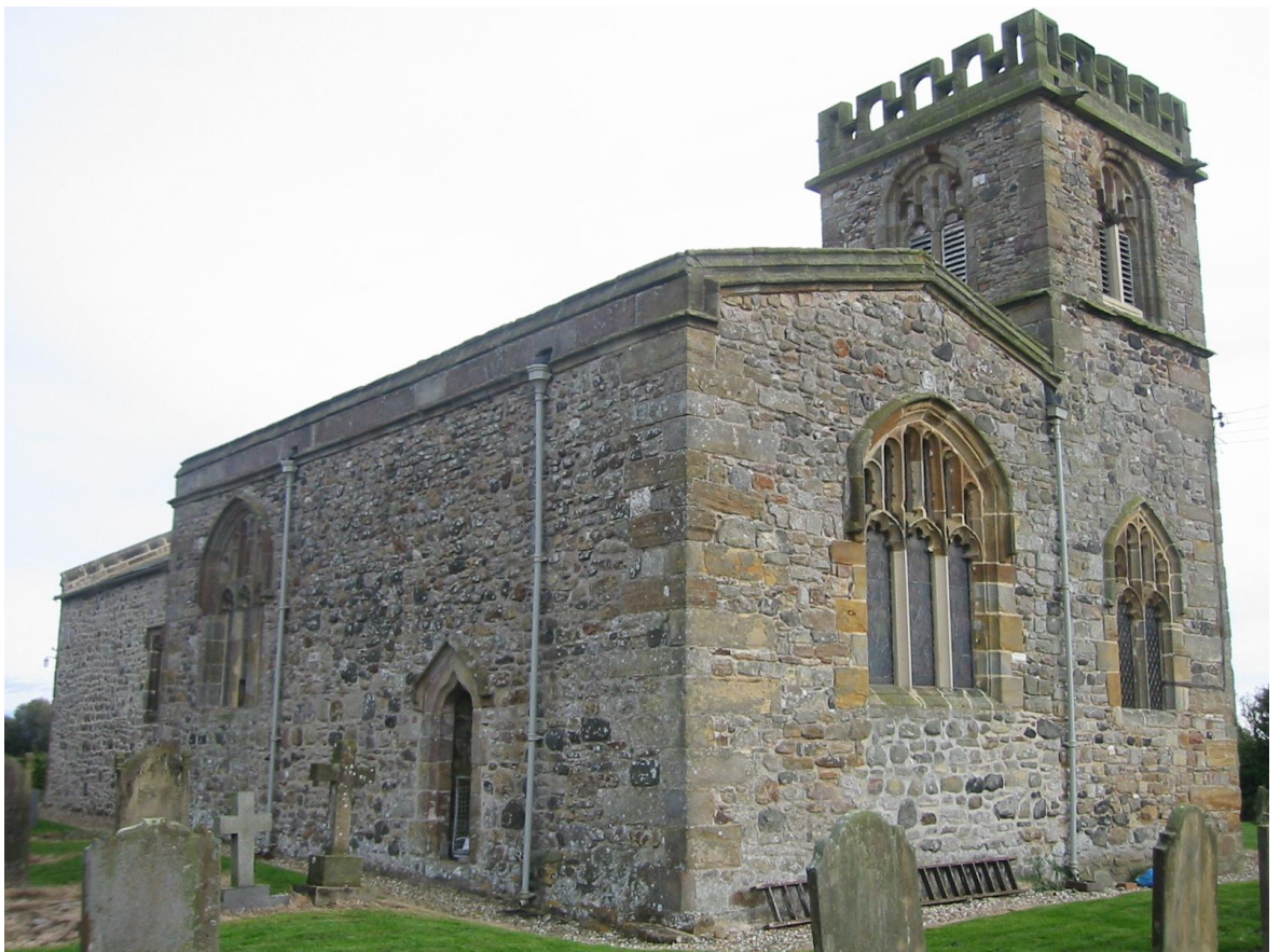
Fig. 115. St Leonard, Barmston from the north-west.
