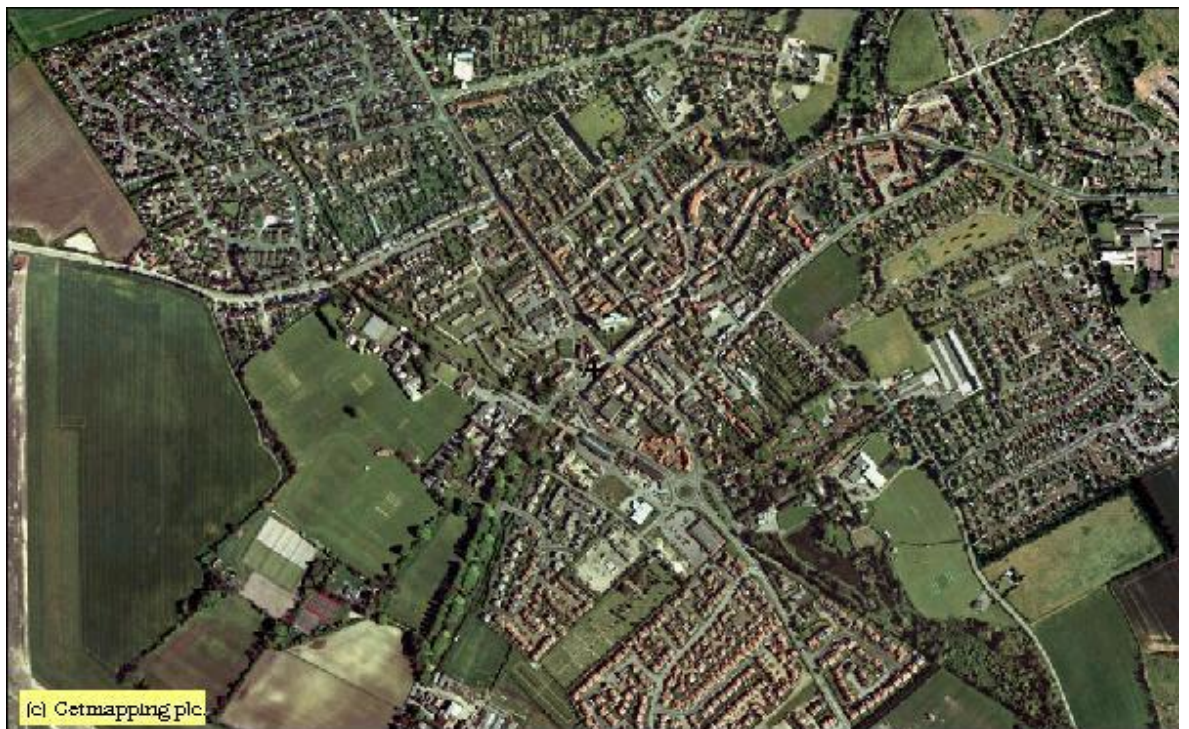
Fig. 154. Aerial view of Pocklington.
