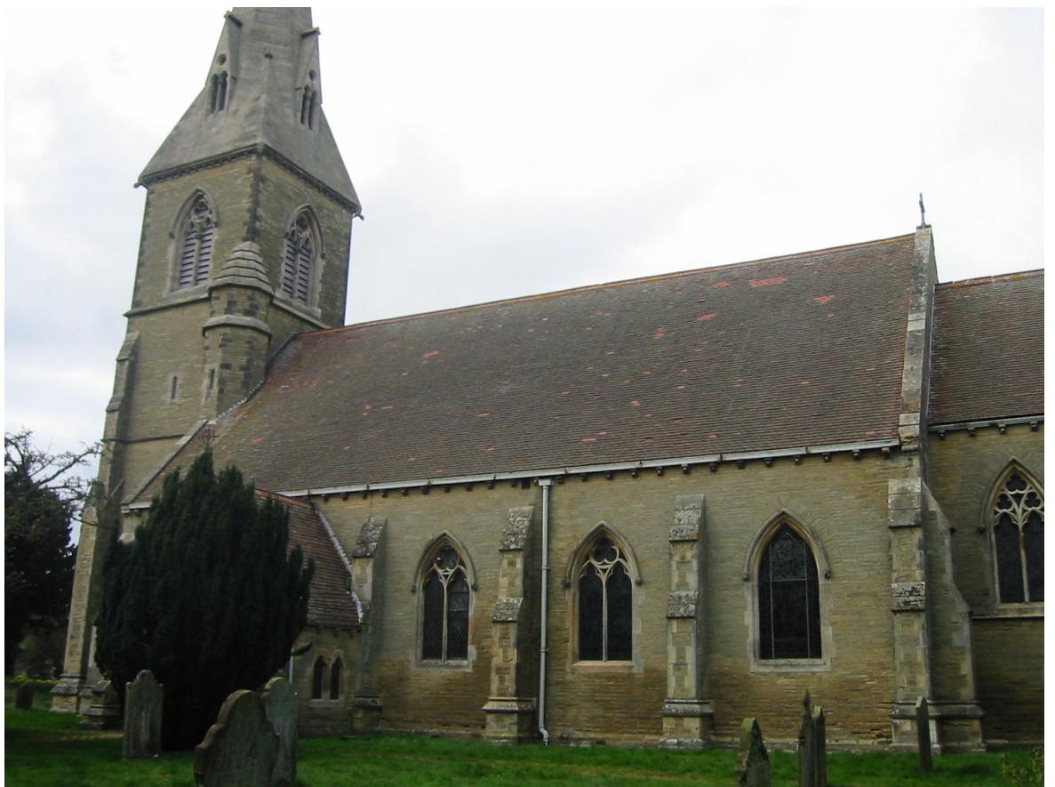
Fig. 244. St James, Warter from the south.
