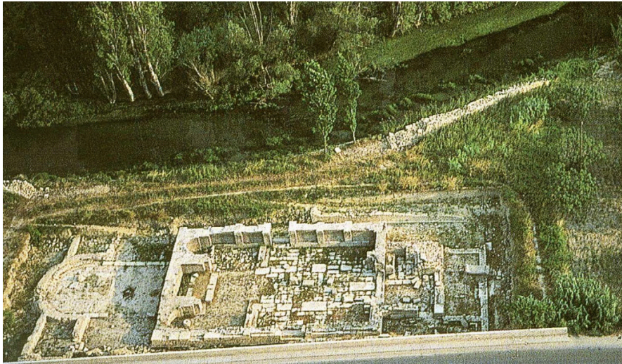
Fig. 151. SS Peter and Moses , Solin: foundations, eleventh century.
