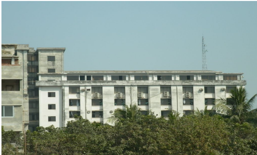
Figure 4.3: Trendmaker Factory Building
