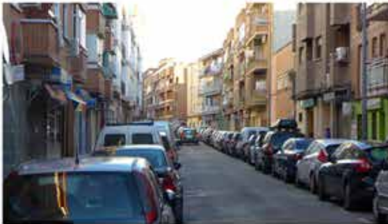
Stage 14- 1980's private residential 4 storey block, in normal side street with shops at ground level
