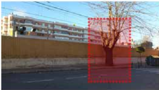
Stage 11- Security Brick wall device in the street. The interface area shows how the device stops permeability between the street and the public station.
