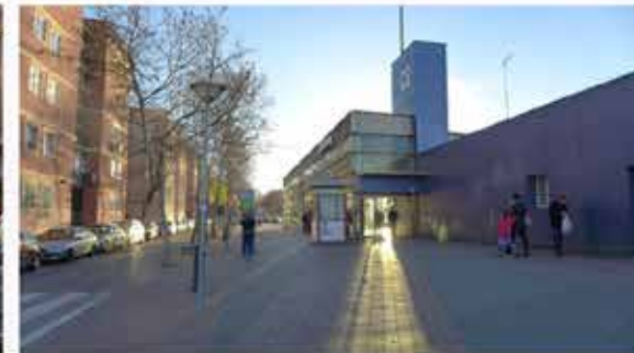
Stage 19- 1970's private residential 4 storey block and New Leganes Train Station
