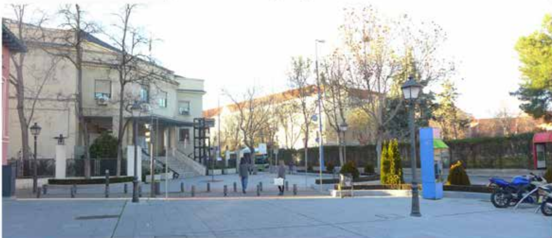
Stage 4- Environment designed to new spatial order: bollards to stop cars entering pedestrian space
