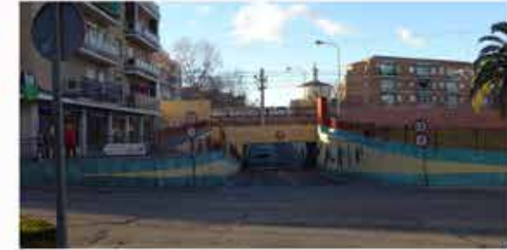
Stage 9- Edge between the town and the motorway with an underpass for cars
