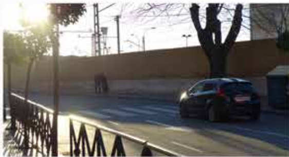
Stage 12- Edge between street and train station: brick wall
