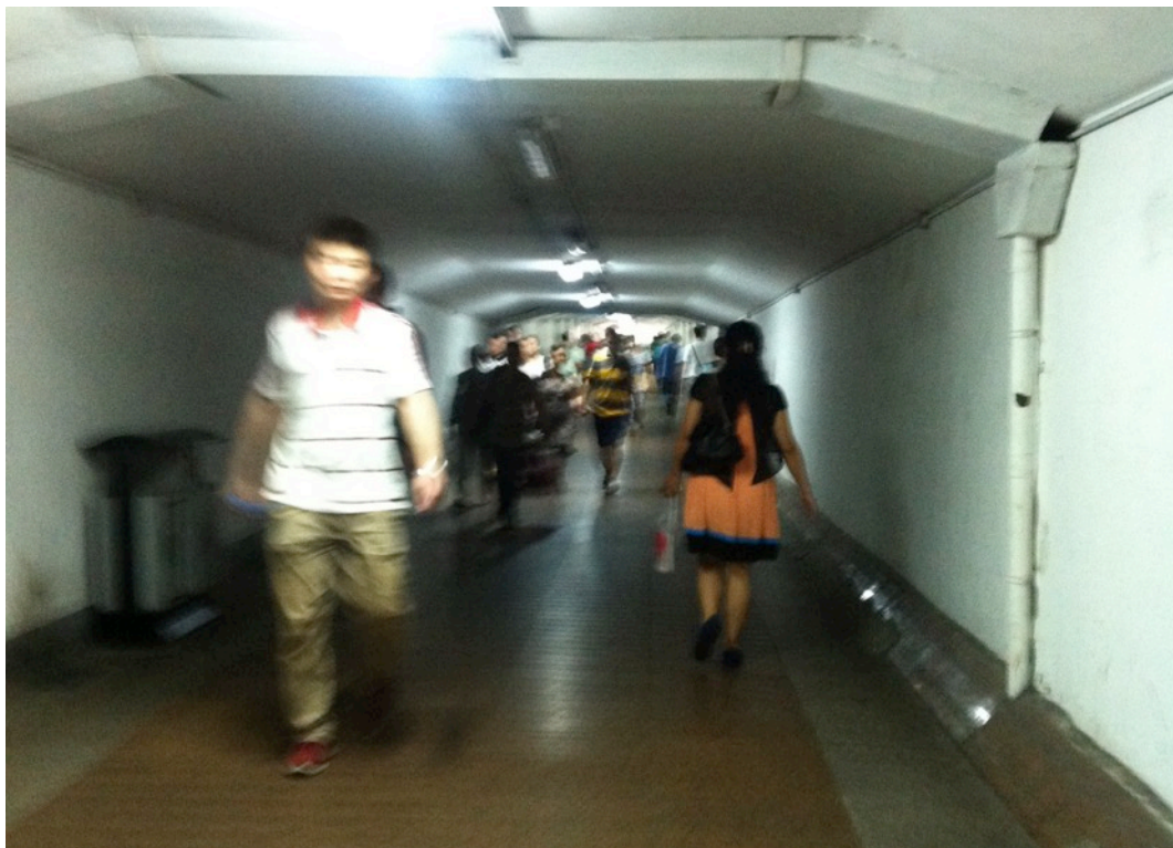
Figure 5.10 Internal view of the Connection Tunnel at the lower ground level of Wuchang Railway Transit Centre
