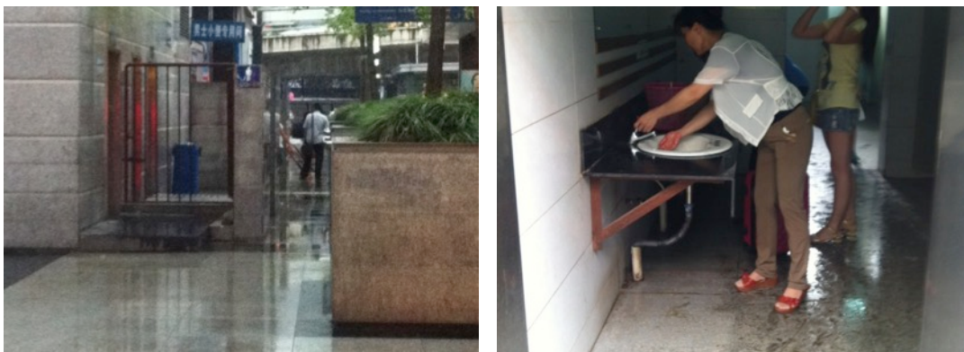
Figure 7.11 Exposed materials inside (left) and outside (outside) public toilets in Wuchang Railway Transit Centre
