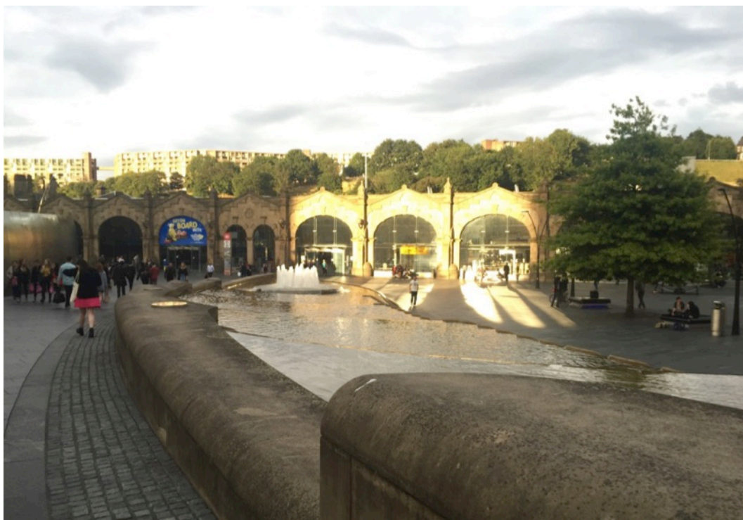
Figure 4.3 A view of Sheffield Railway Station from Sheaf Square
