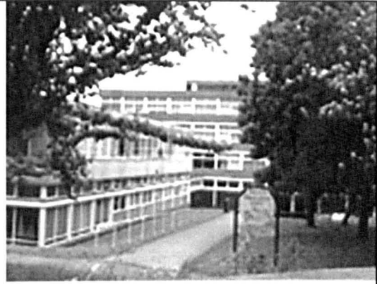
b) School gate for pedestrians
