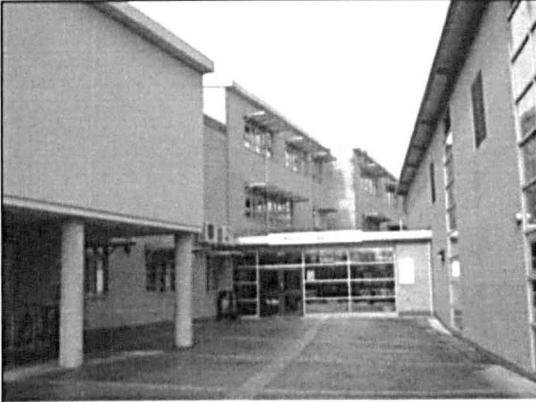
a) Entrance area
