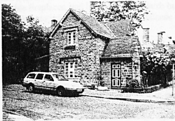
Figure 8.7: Gate-keeper's lodge, Broomhall
