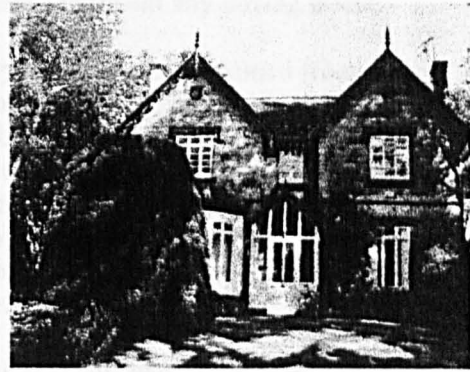
Figure 7.8: No. 9 Broomfield Road
