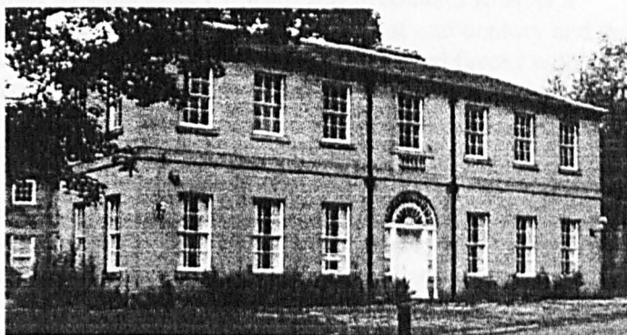
Figure 8.2: Broom Hall - East Wing
