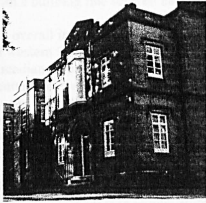
Figure 7.7: Corner of Broomfield Road and Newbould Lane
