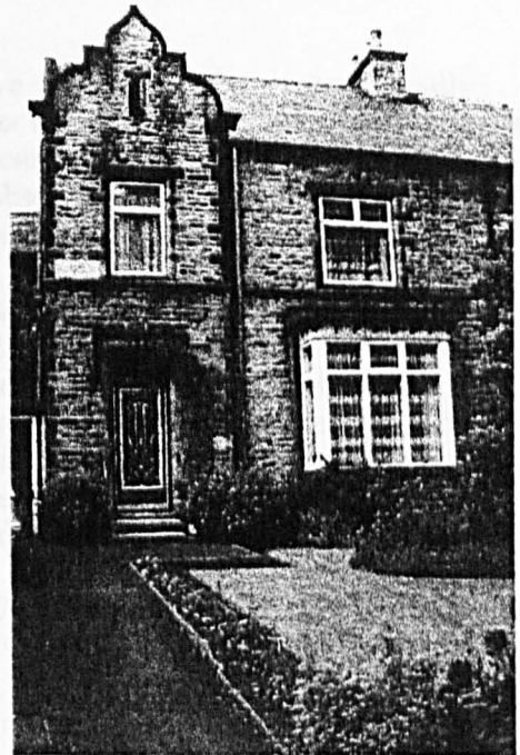
Figure 8.6: Semi-detached house, Broomhall
