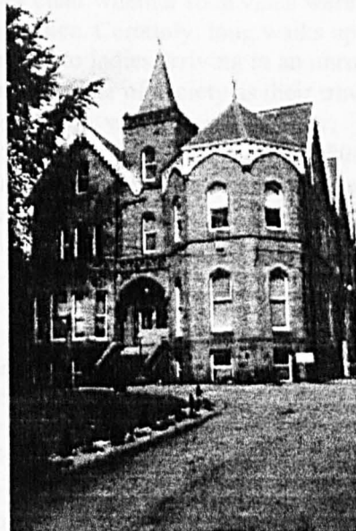
Figure 7.10: No. 11 Broomfield Road
