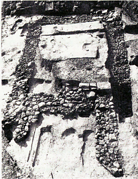
Figure 3.5. A stone building at Pontefract (Note the larger cell post-dates the phases of activity considered in the present study) (photo courtesy of WYAS).
