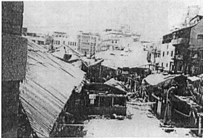
Figure 5.5 The condition of the fabric is very poor. Photo taken in Aug. 2000
