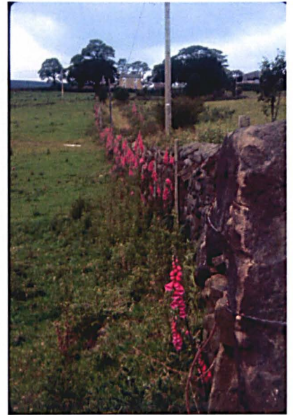
Dry stone walls need maintenance.
