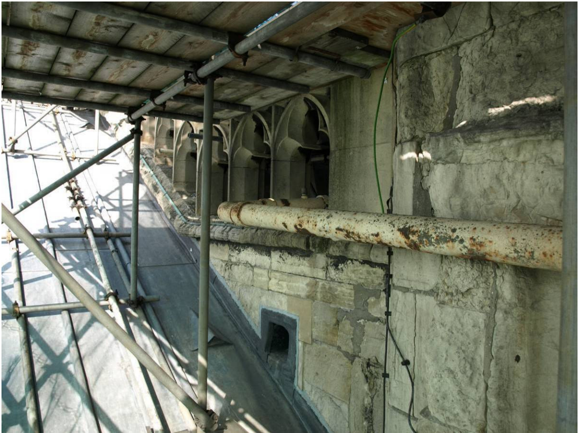
Figure 274: East Front, west face at main parapet level, south side
