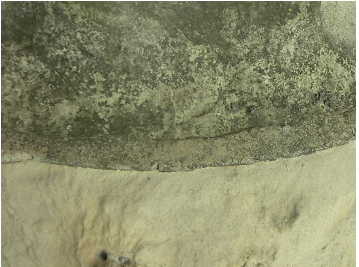
Figure 378: Seated figure, cement/New Ketton pointing between torso and head section
