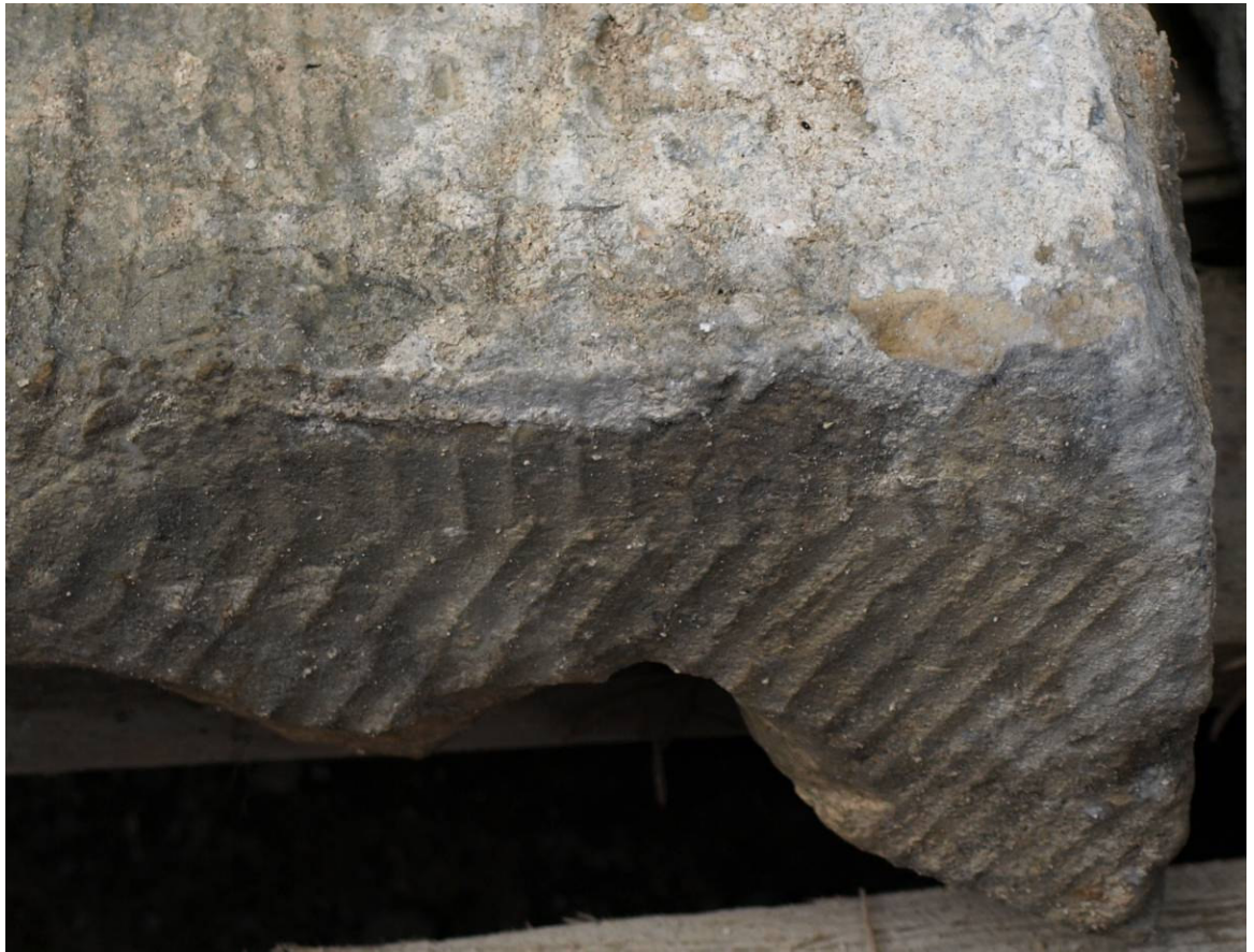
Figure 132: Plain bolster or boaster tooling, eighteenth century
