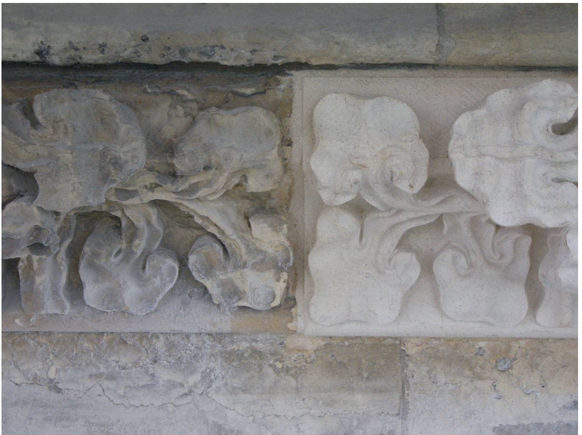
Figure 463: North-clerestory cornice bay 1 after renewal, comparison of existing and new work
