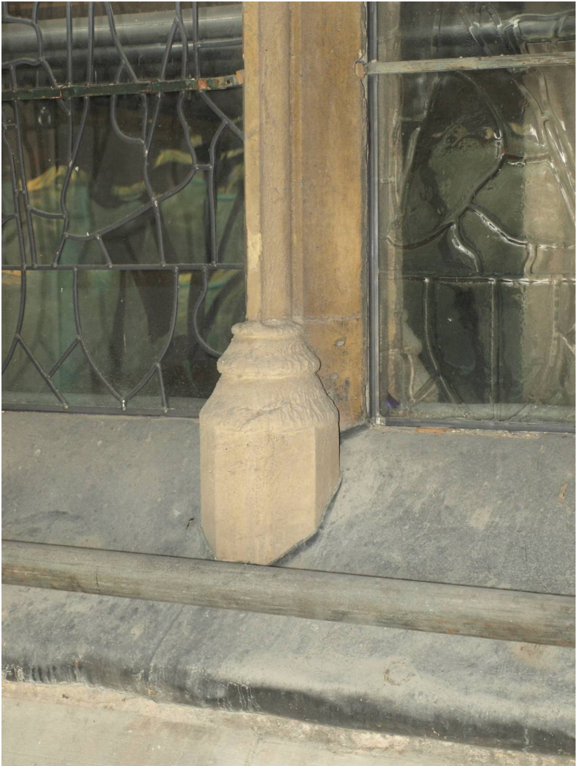
Figure 304: East Front, Great East Window exterior, sill, stooling and mullion detail
