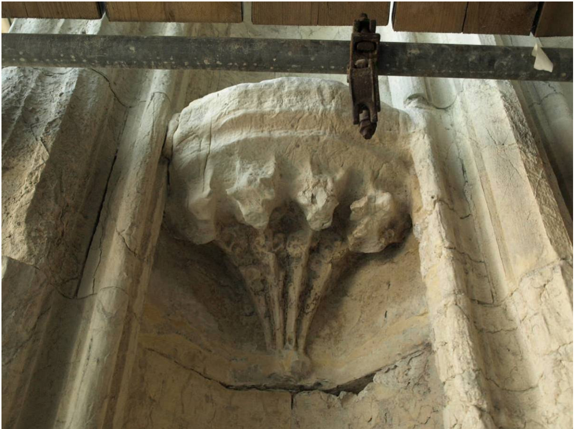
Figure 255: East Front, fourteenth-century niche-pedestal in south buttress, Level D
