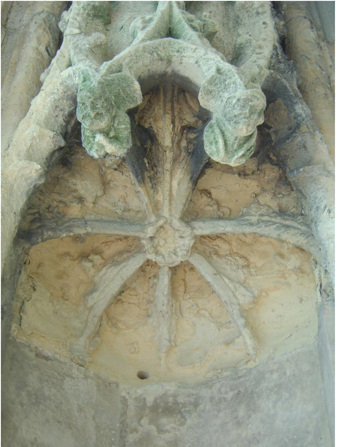
Figure 441: East Front, south-buttress canopy before conservation by Lee Godfrey
