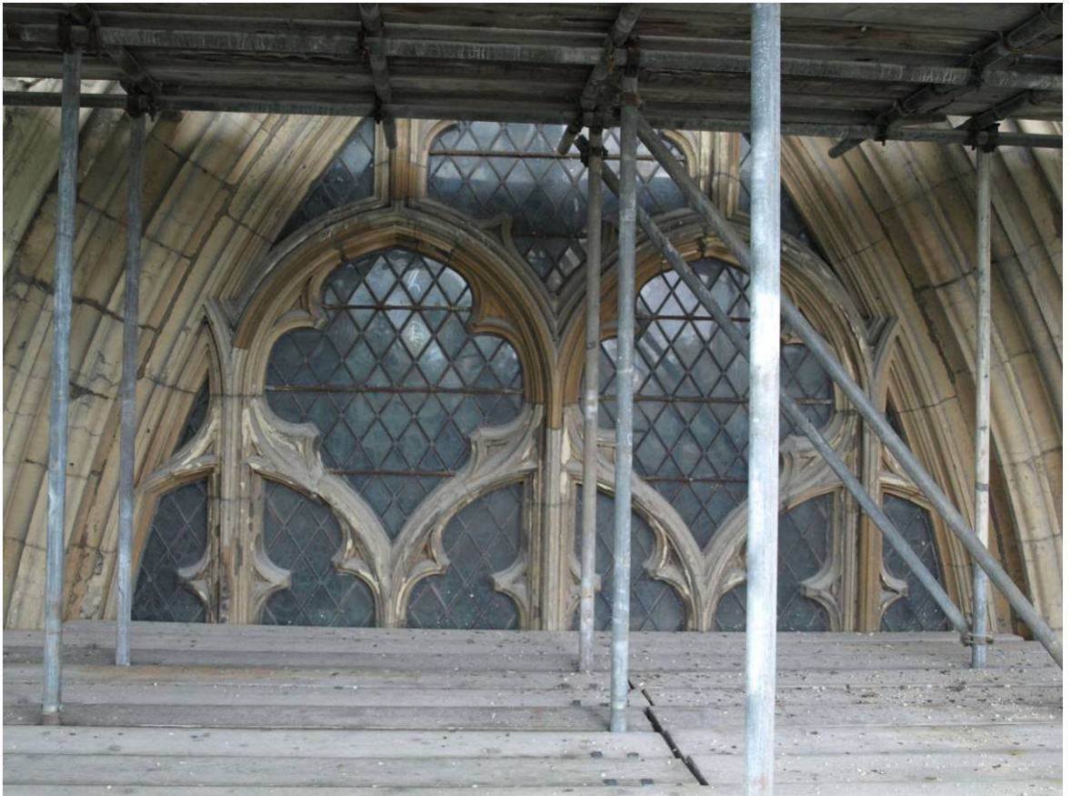
Figure 168: East Front, east window of south aisle, tracery, Level B
