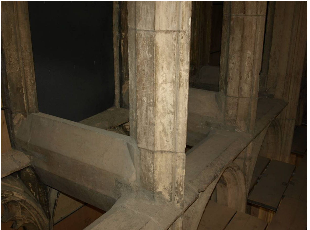
Figure 316: Great East Window interior, inner screenwork showing through-stones to outer masonry
