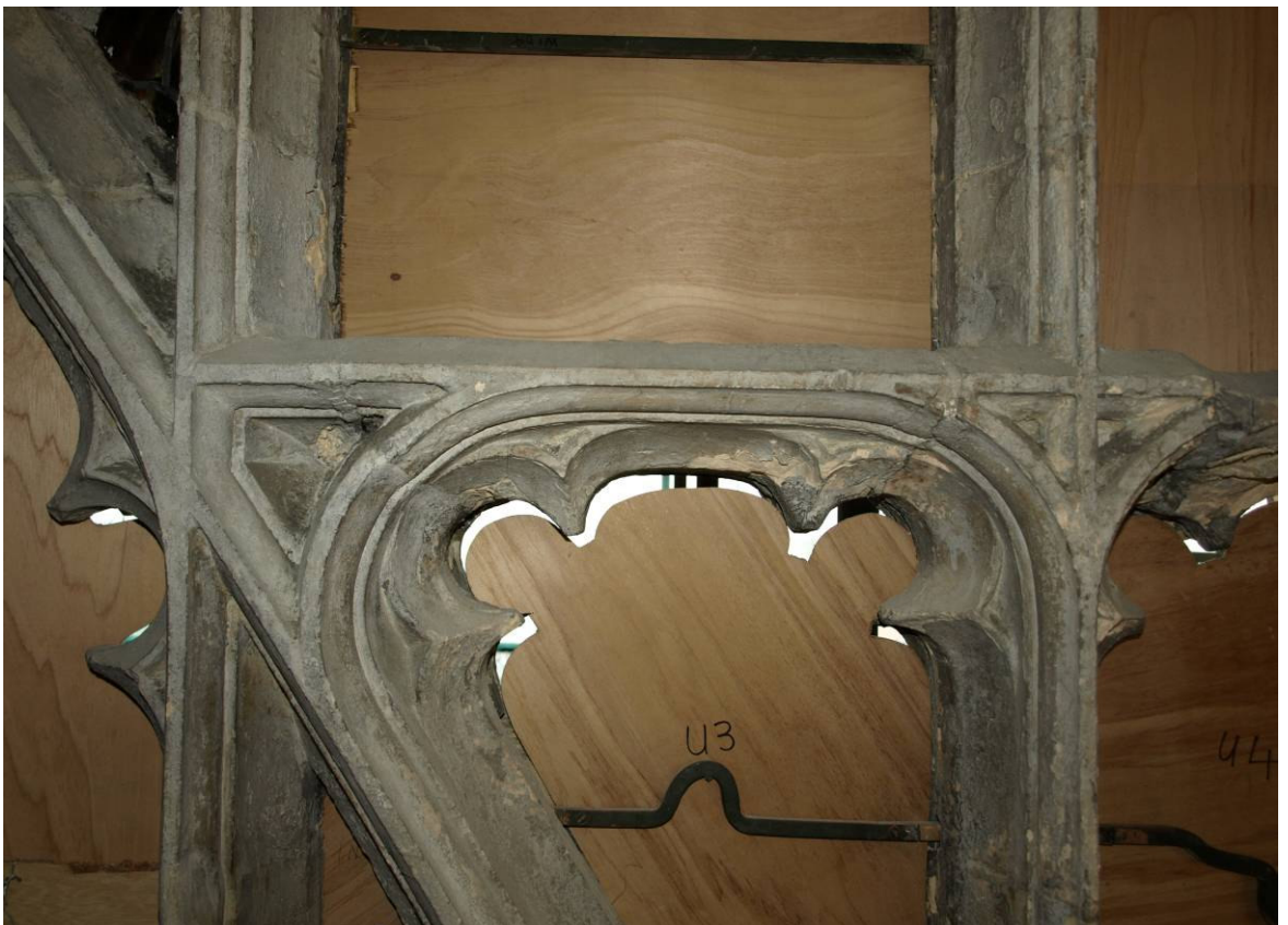
Figure 312: Great East Window interior, detail showing removal of medieval foliage during 1820s, plus 1970s limewash
