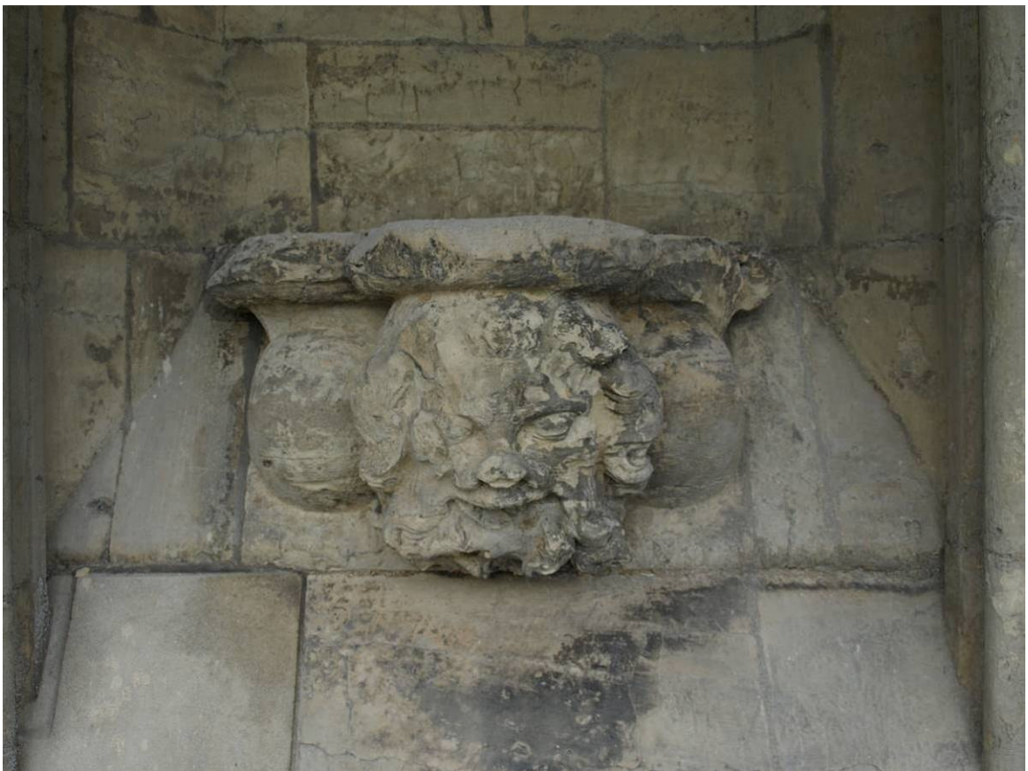
Figure 187: East Front, base of niche in south buttress, Level A
