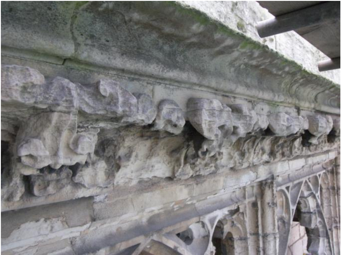
Figure 462: North-clerestory cornice bay 2 before renewal
