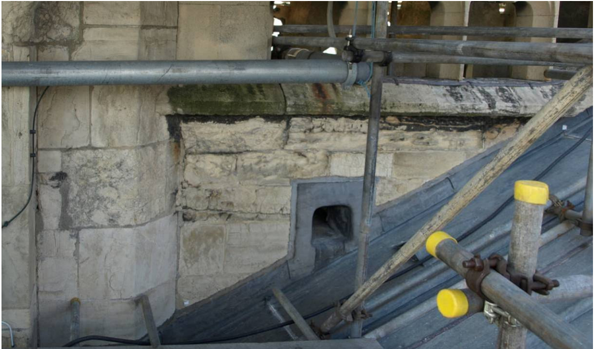
Figure 276: East Front, west face at main parapet level, north side
