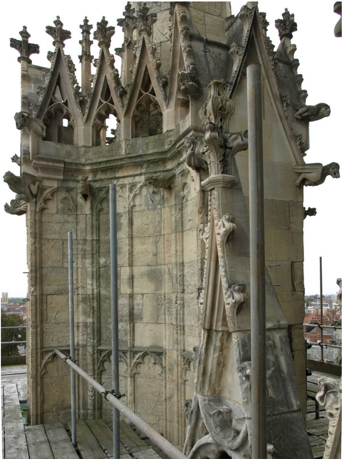
Figure 240: East Front, south-east turret, upper masonry, Level D
