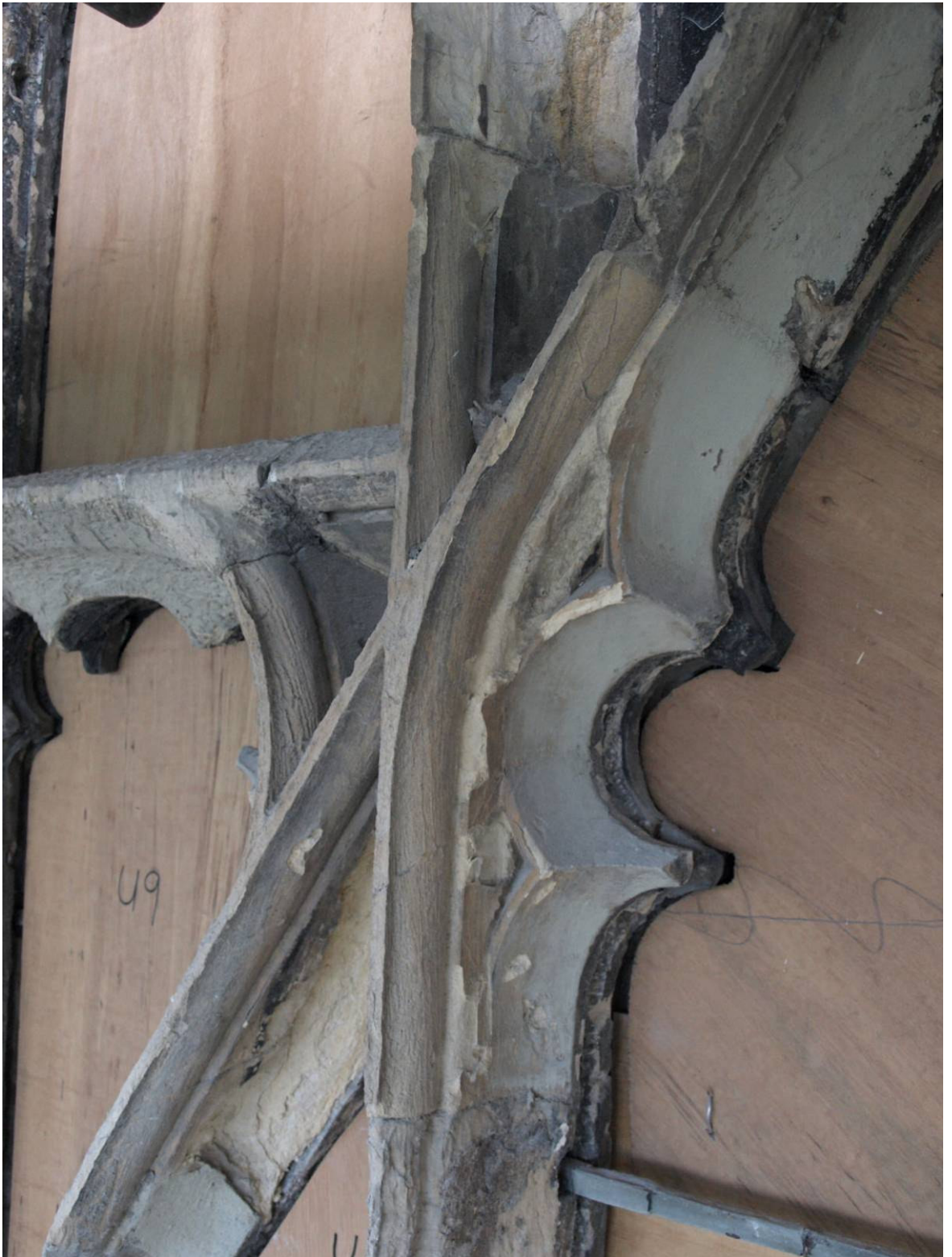
Figure 310: Great East Window exterior, tracery detail showing 1820s insert
