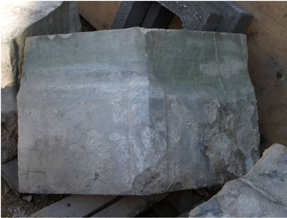
Figure 290: Removed broach-stone from below spirelet, south buttress, showing concealed and damaged moulding
