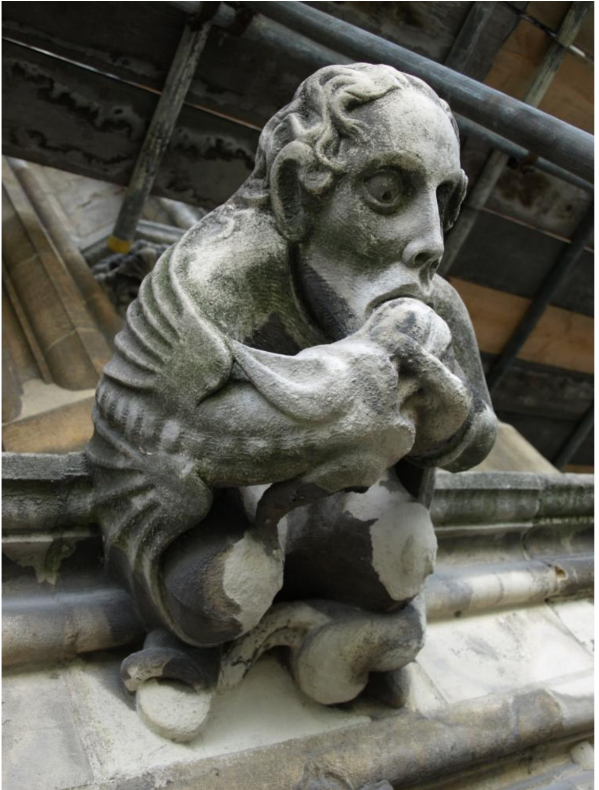
Figure 459: East Front, Huddleston-stone grotesque on north buttress, c.1970
