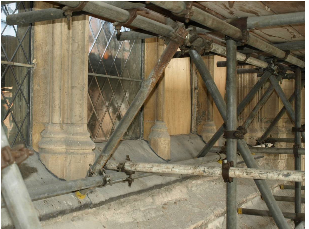
Figure 303: East Front, Great East Window exterior, sill, stoolings and mullions
