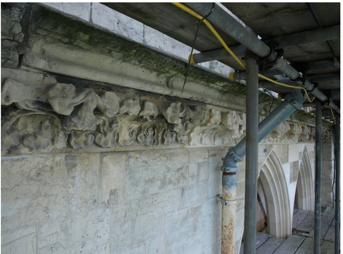
Figure 273: Thoresby's east end, north-clerestory cornice, 1830s with recent replacements (2006)
