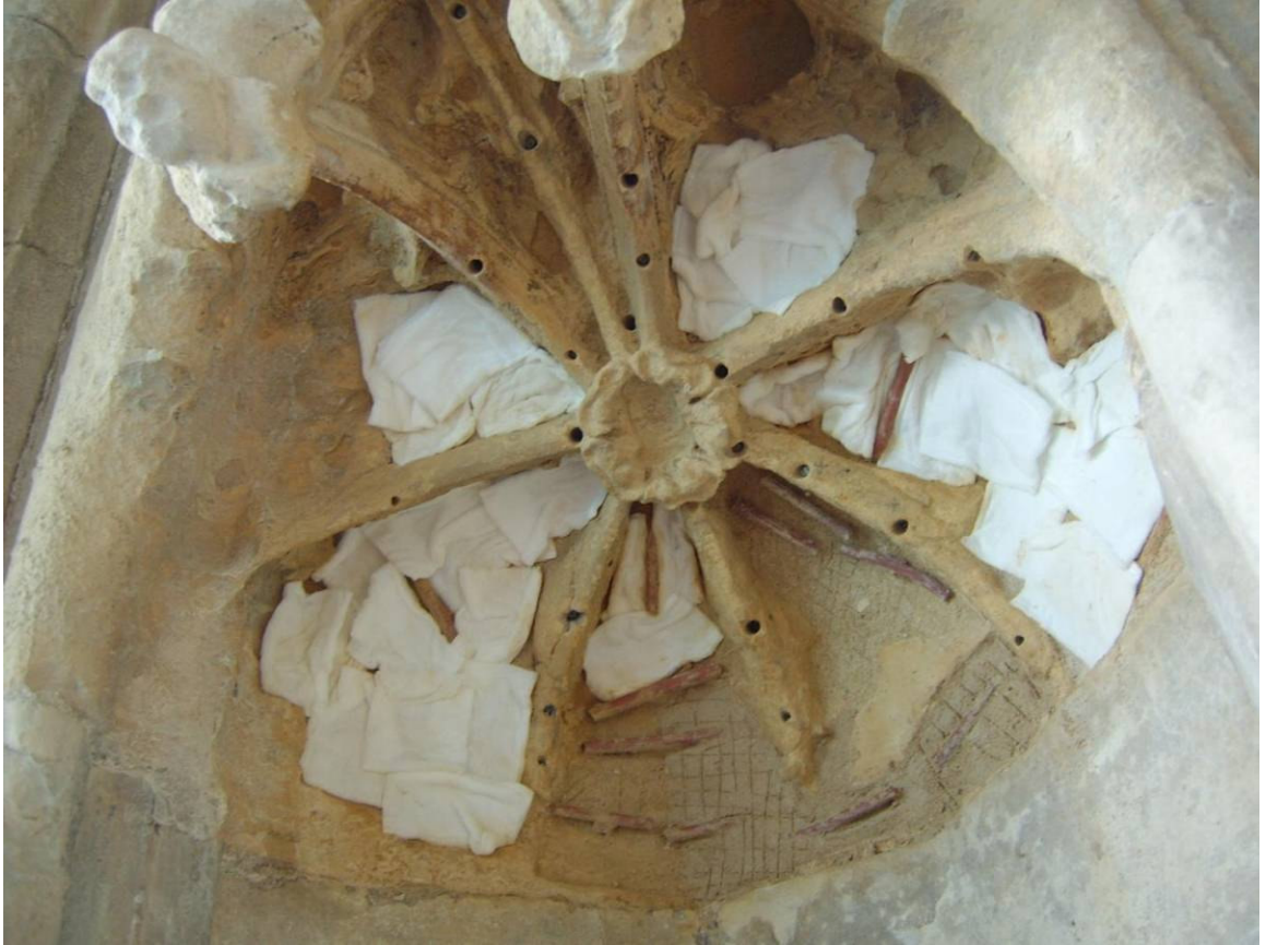
Figure 443: East Front, south-buttress canopy during mortar repair
