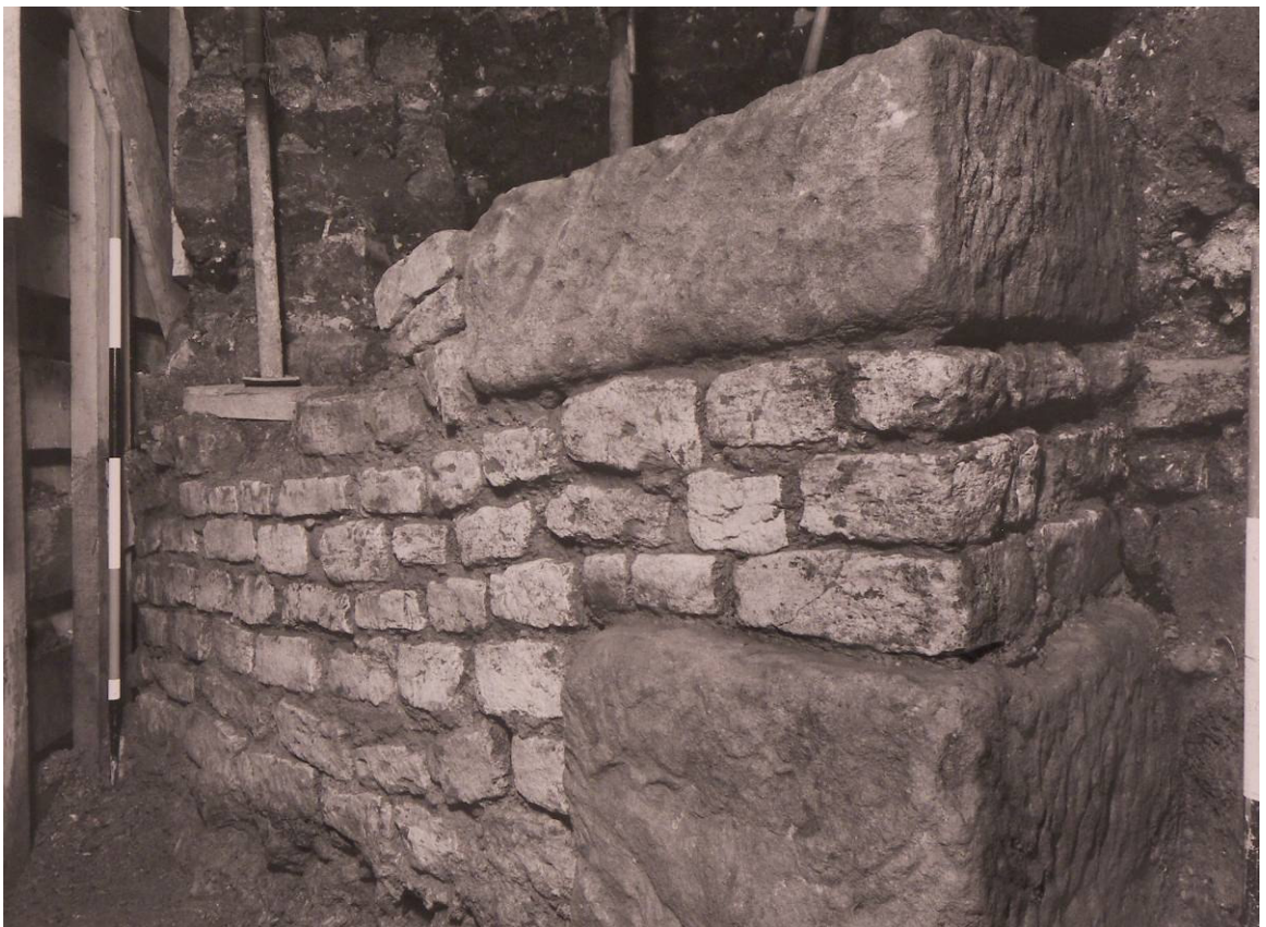
Figure 157: In situ Roman masonry beneath north-aisle wall west of north-east turret of East Front, 1969 (YML/YMEX/6492)
