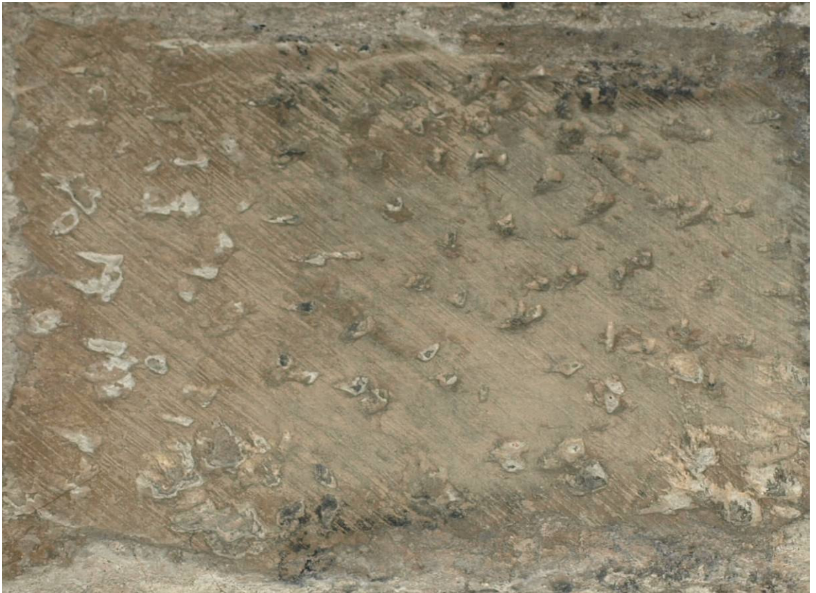
Figure 130: Punched tooling, late medieval on re-used twelfth-century ashlar
