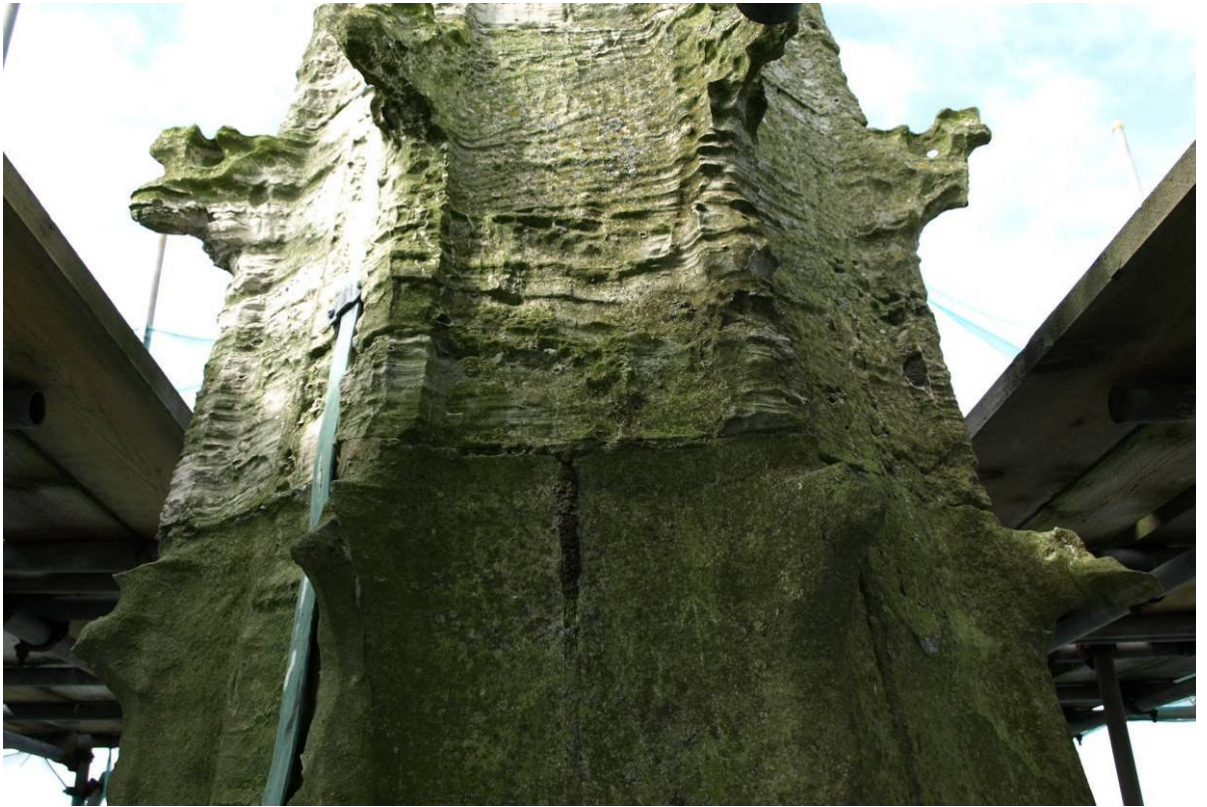
Figure 281: East Front, south-buttress spirelet, Level I, showing differentiation between nineteenth and eighteenth-century stone types and stages in crocket weathering
