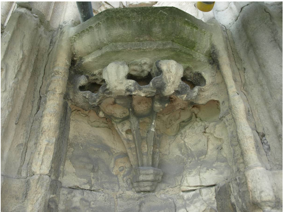
Figure 259: East Front, nineteenth-century niche-pedestal in north buttress, Level D
