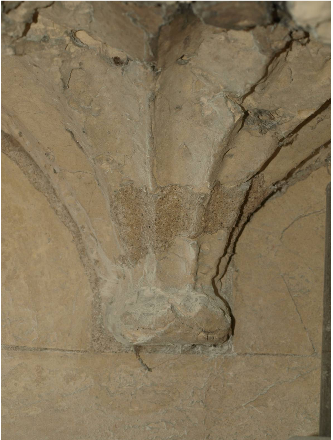
Figure 446: East Front, central vessel, historic lime-mortar repair
