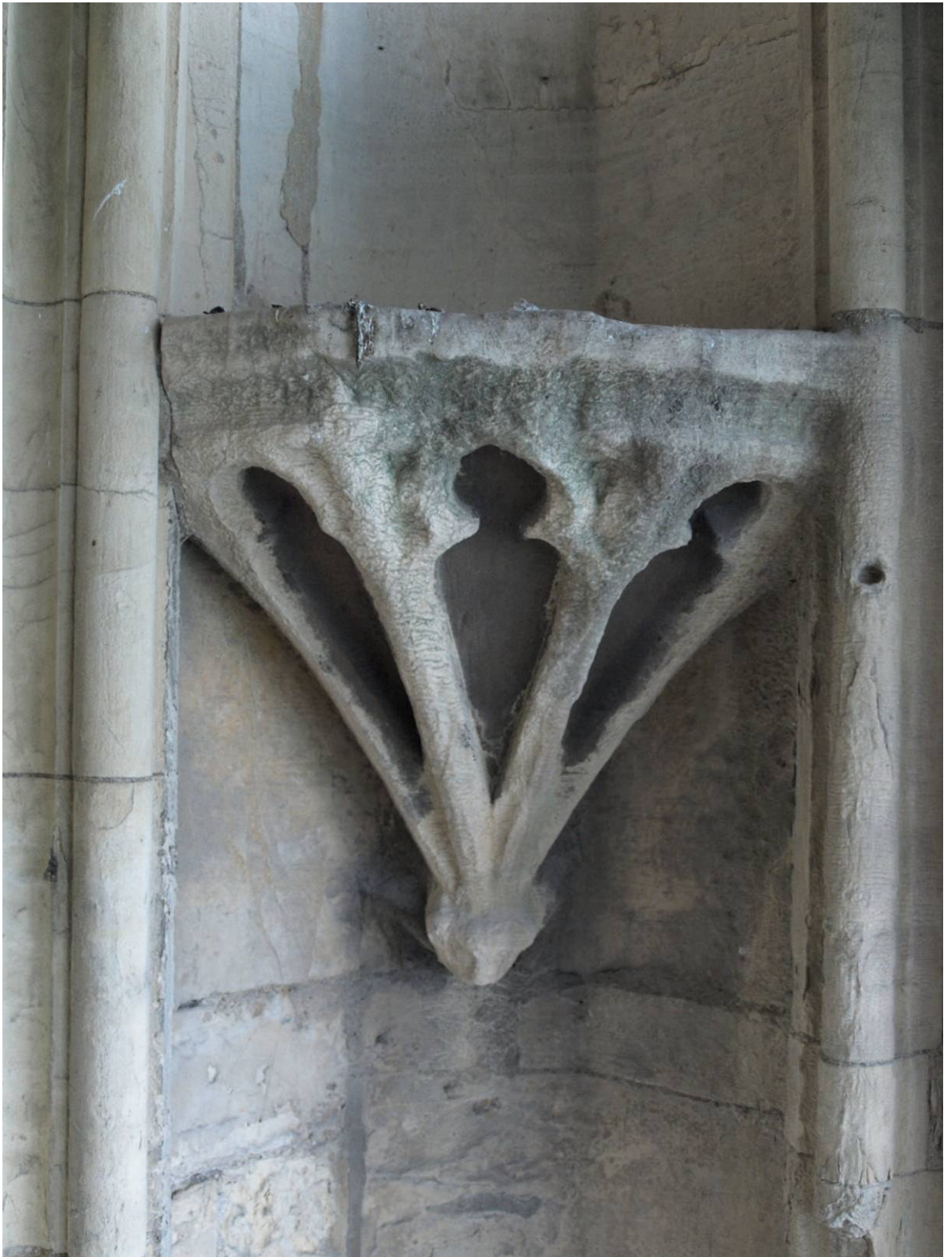
Figure 227: East Front, south-buttness fourteenth-century console detail, Level C
