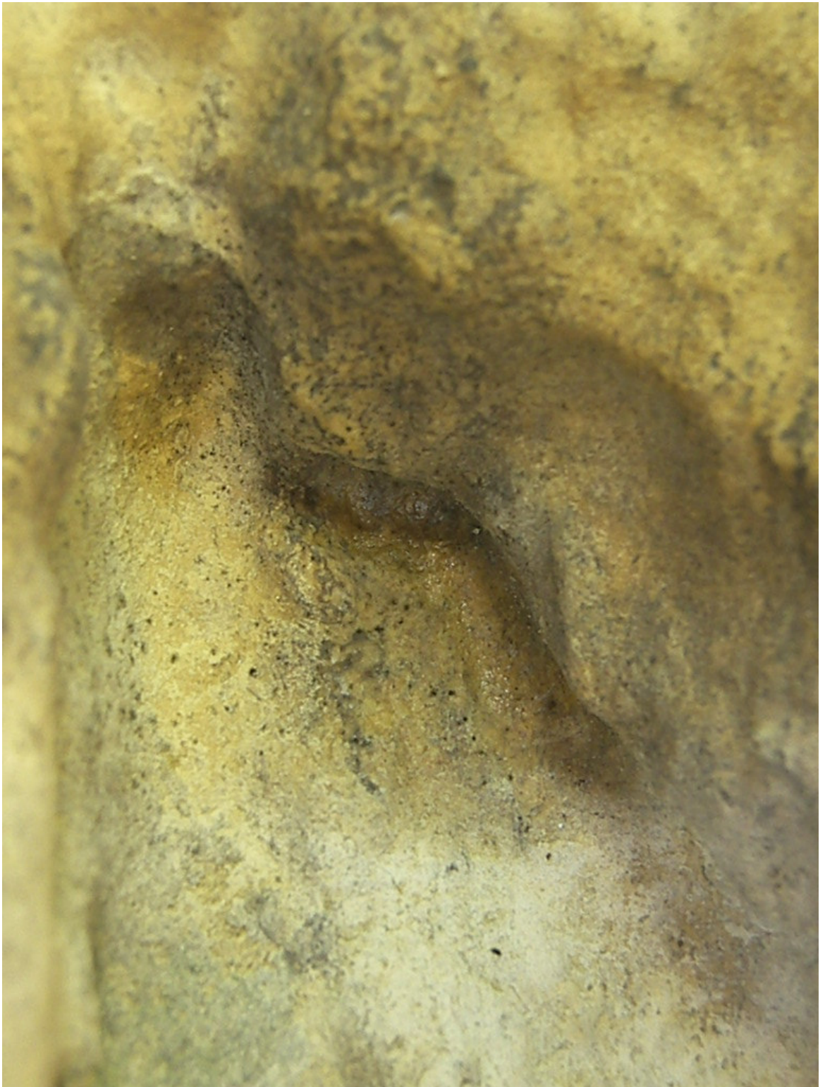
Figure 458: Example of effect of linseed oil, south-aisle parapet trial area, January 2008
