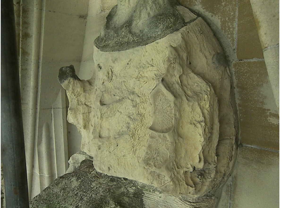
Figure 375: Seated figure, detail of torso section from north-east. Note face-bedding of stone
