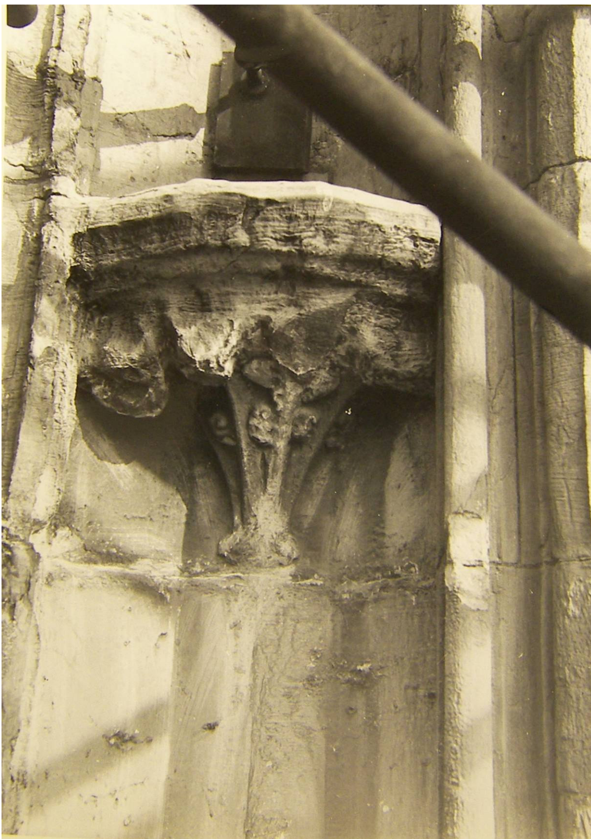
Figure 76: East Front, buttress-console detail, 1955 (YML/APYM/A57iv/C1+)
