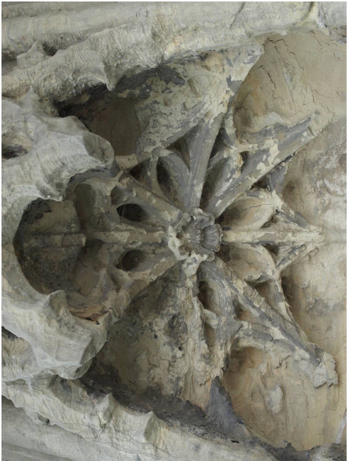
Figure 6: Example of sheltered decay at York Minster, nineteenth-century niche-head of south buttress, East Front (landscape)
