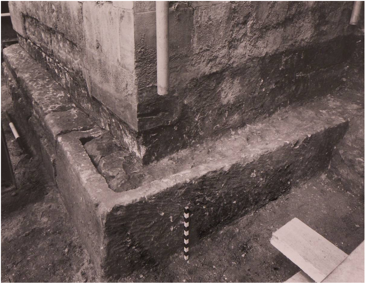
Figure 160: Foundations of first buttress west of south-east turret, 1969 (YML/YMEX/6481)
