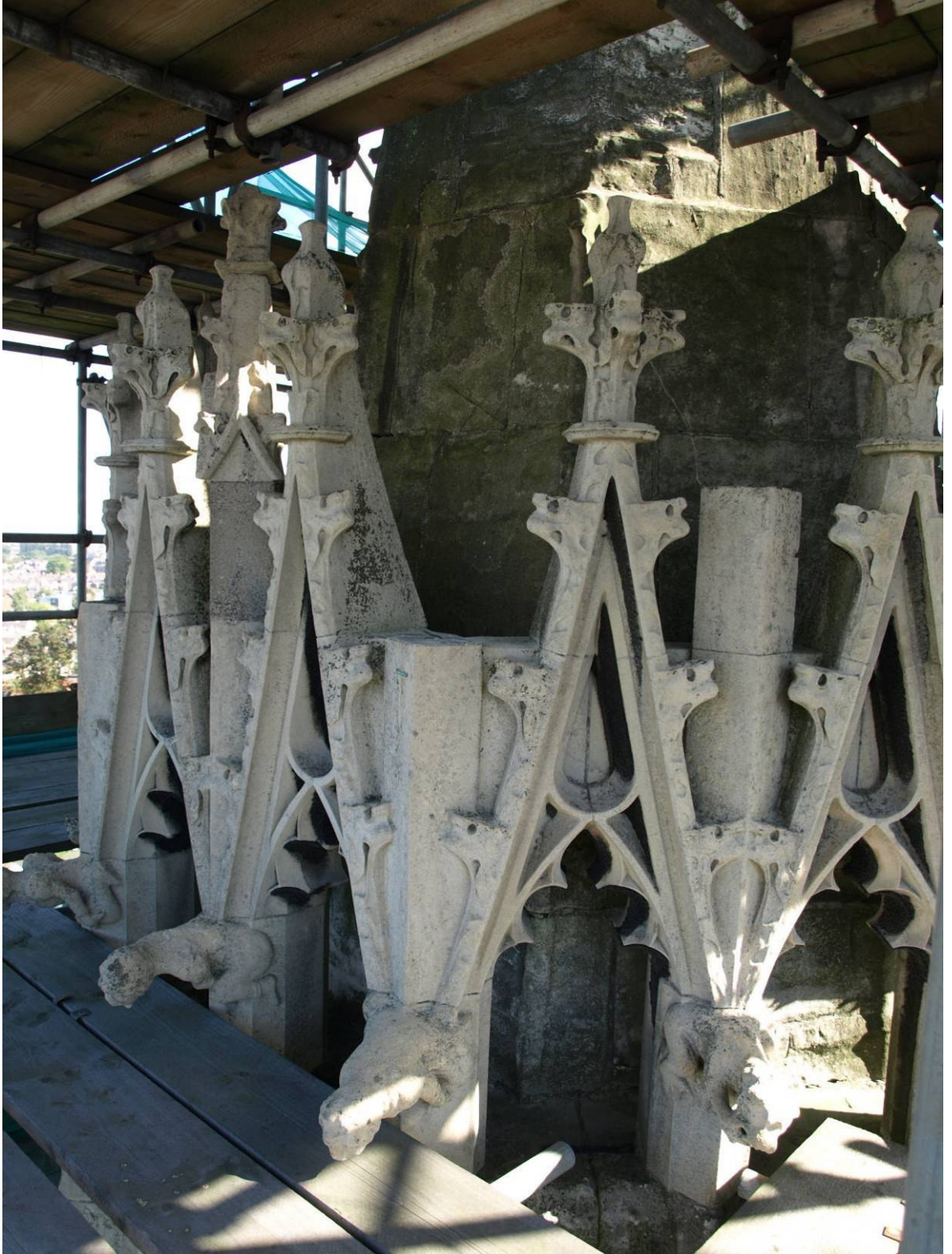
Figure 279: East Front, north-butress corona, Level H
