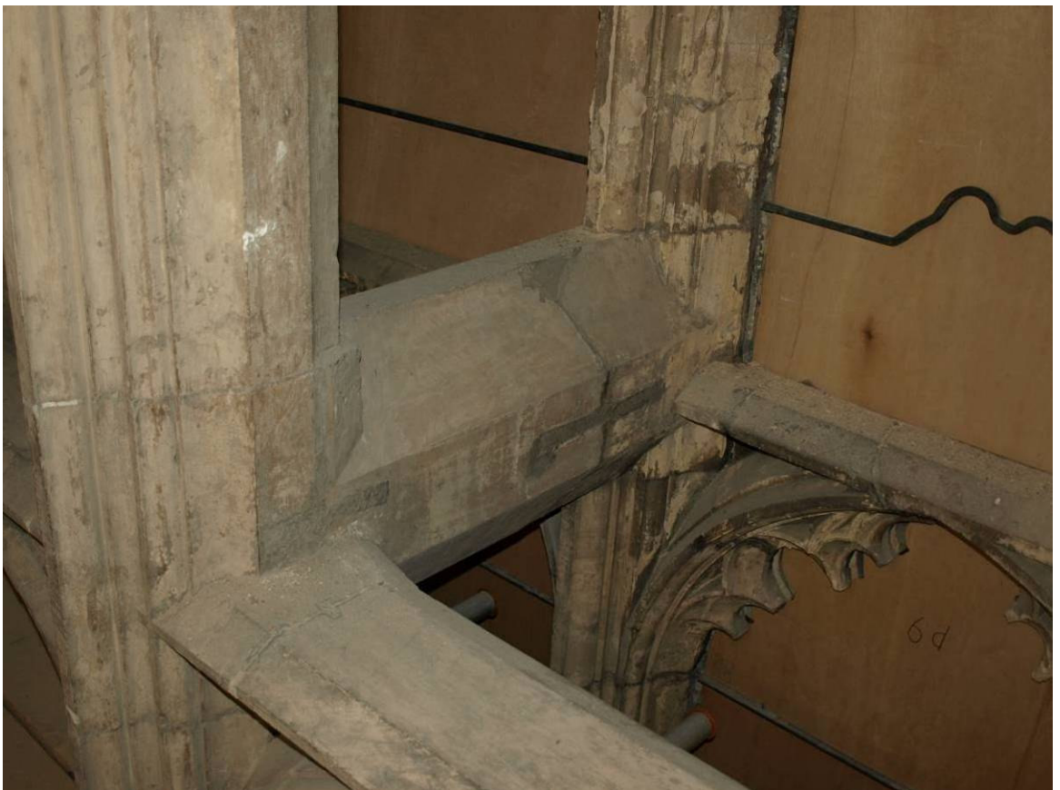
Figure 319: Great East Window interior, detail showing cramping of 1820s through-stone
