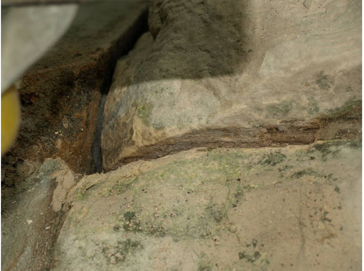
Figure 382: Seated figure, base stone, bottom bed, claw tooling
