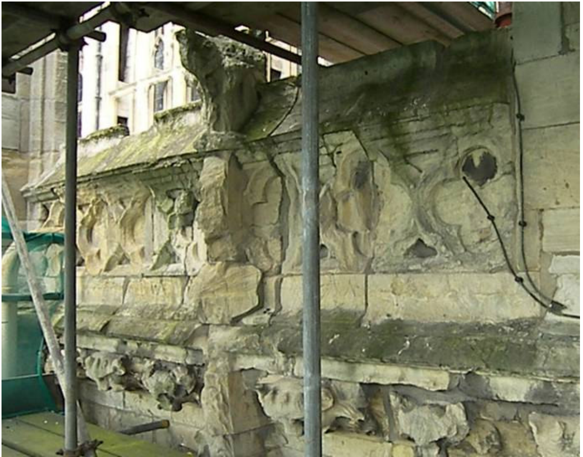
Figure 453: York Minster, aisle parapet, easternmost bay before surface treatment trials, July 2007
