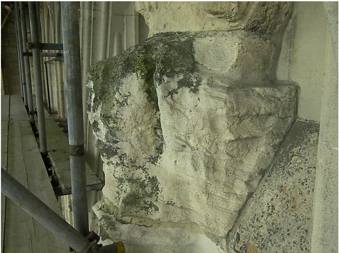
Figure 373: Seated figure, detail of base stone from north-east (note natural bedding of stone)
