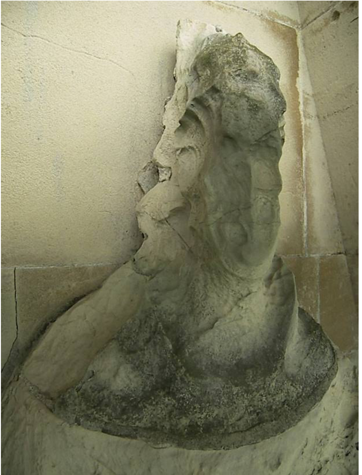
Figure 377: Seated figure, head section from south-east. Note face-bedding of stone
