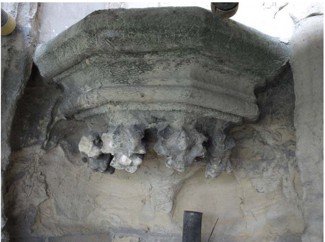
Figure 271: East Front, nineteenth-century niche-pedestal, north side of Great East Window, Level D
