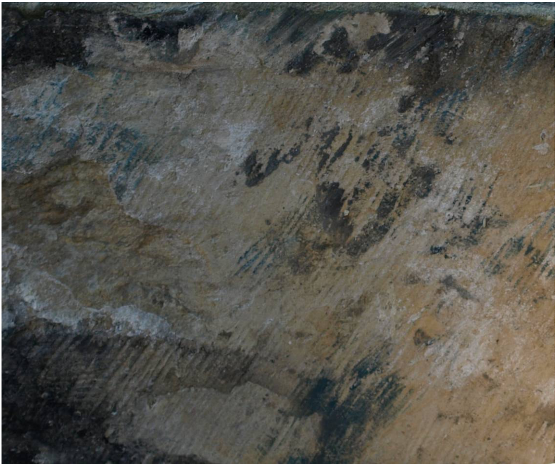
Figure 133: Plain bolster or boaster tooling, nineteenth century
