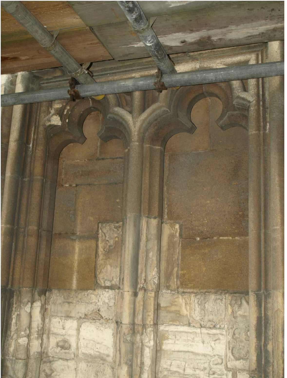
Figure 212: East Front, recesses in north-east turret, Level B
