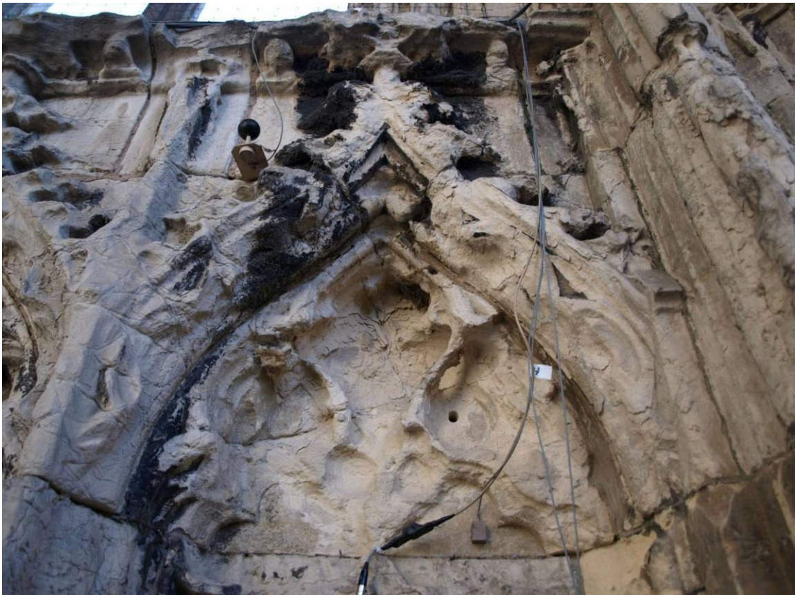
Figure 448: Howden Minster Chapter House, arcade panel before conservation trials
