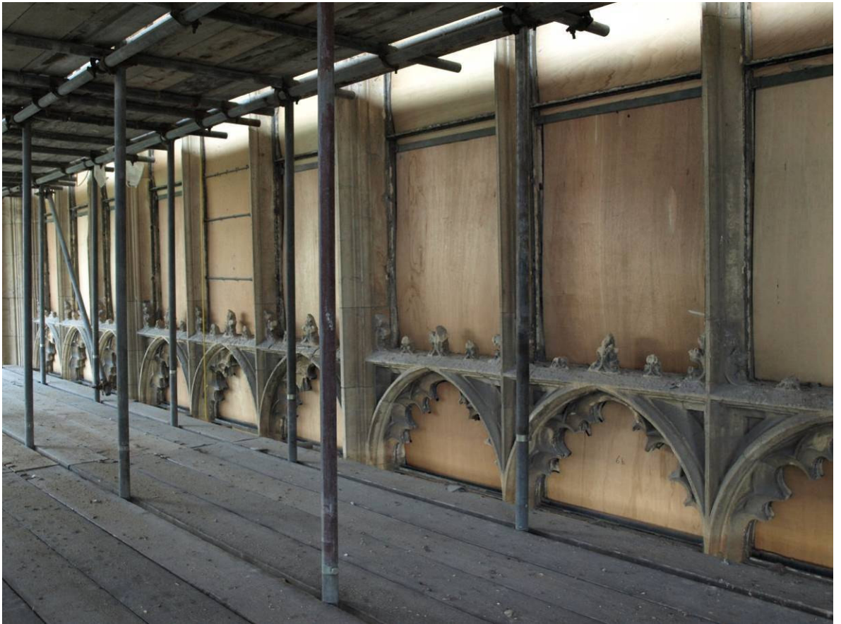
Figure 305: East Front, Great East Window exterior, lower transom and mullions
