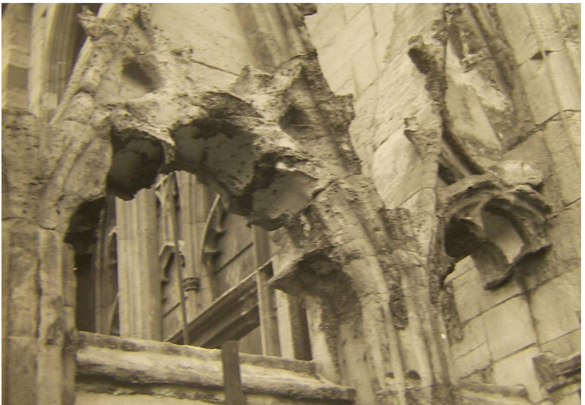
Figure 75: East Front, south parapet detail, 1954 (YML/APYM/A57iv/S15)
