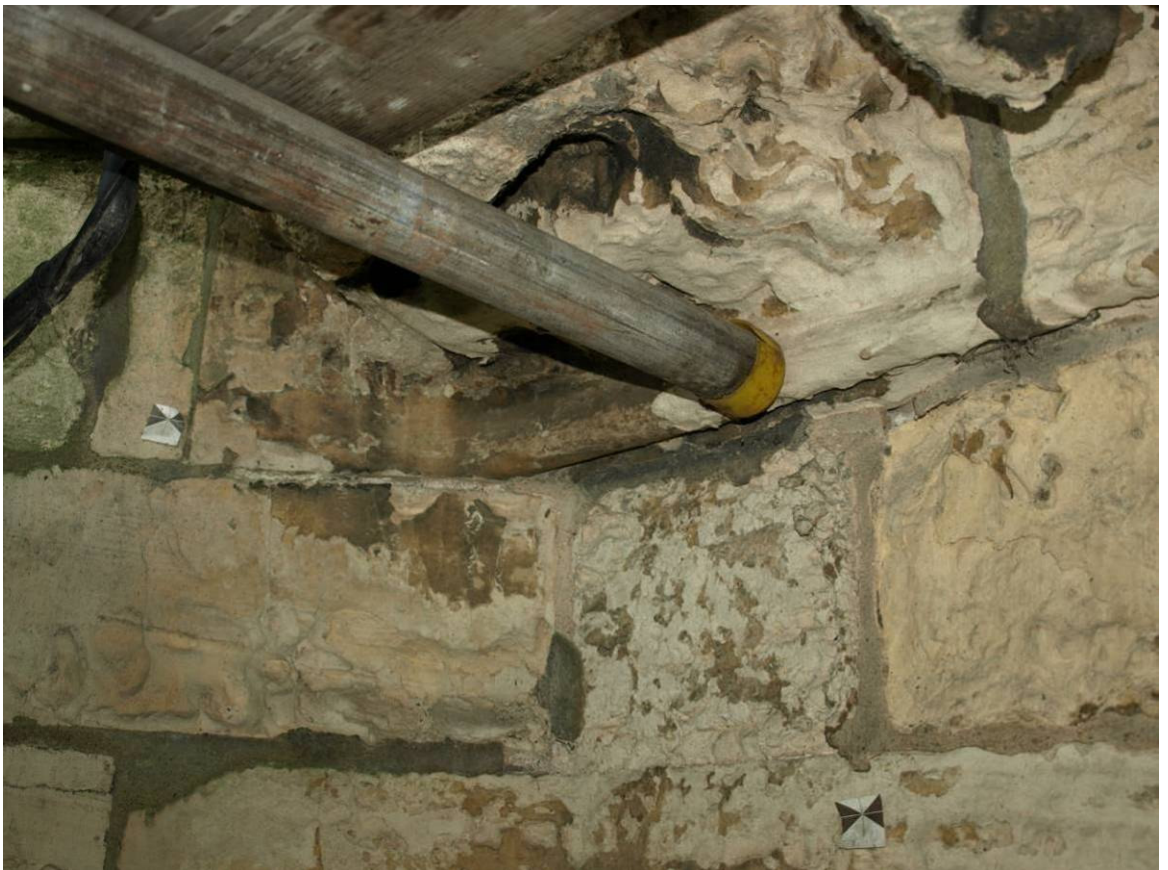
Figure 208: Junction between north-aisle cornice and north-east turret, Level B
