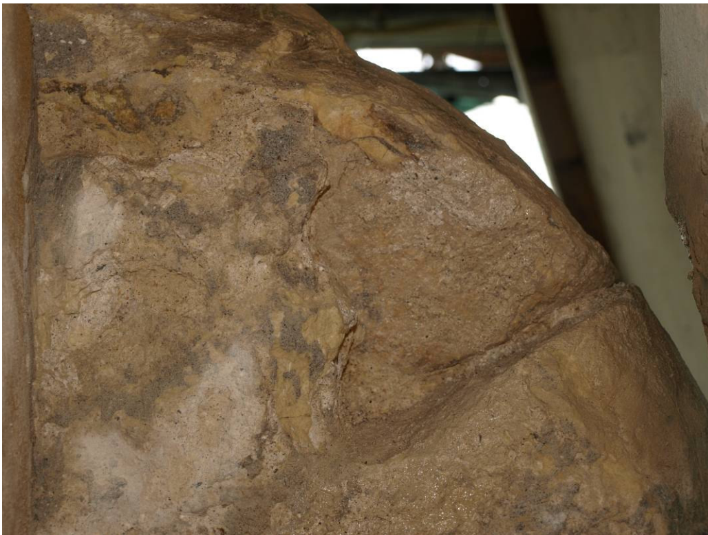
Figure 389: Seated figure, view through rear face of parapet to right-hand shoulder of statue with detached fragment removed to reveal calcite fault. Note white repointing mortar over re-fixing mortar
