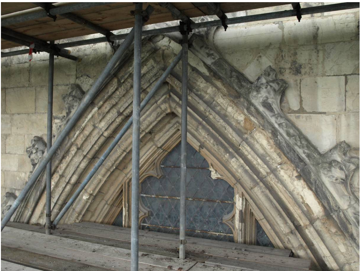
Figure 173: East Front, east window of north aisle, Level B
