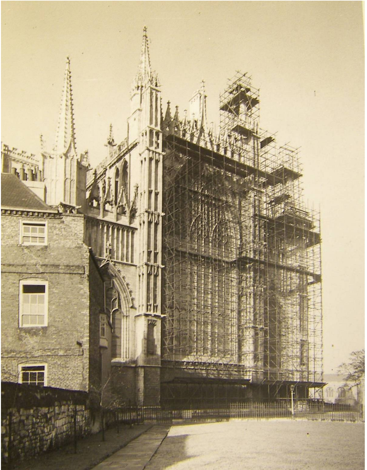
Figure 64: The East Front during the 1950s repairs (YML/APYM/A55)
