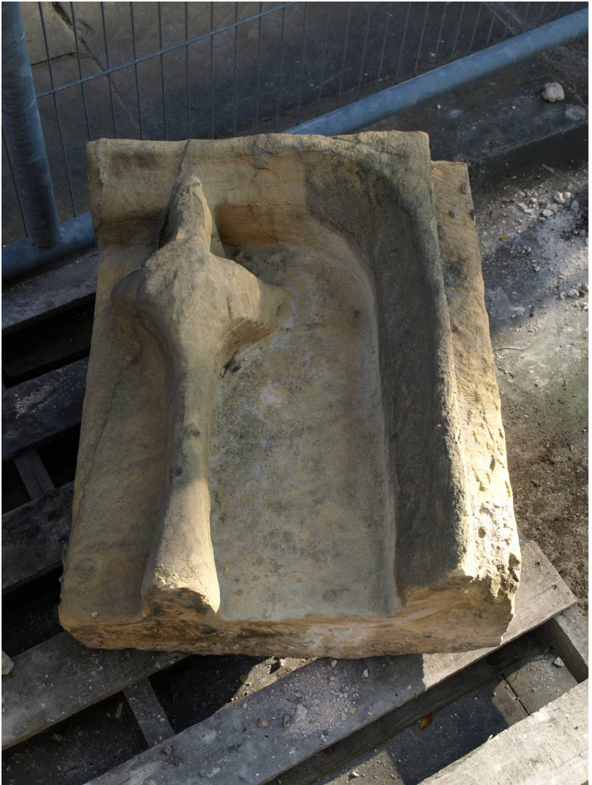
Figure 295: Removed nineteenth-century indent from south buttress, Level F, illustrating shallow depth of replacement stone
