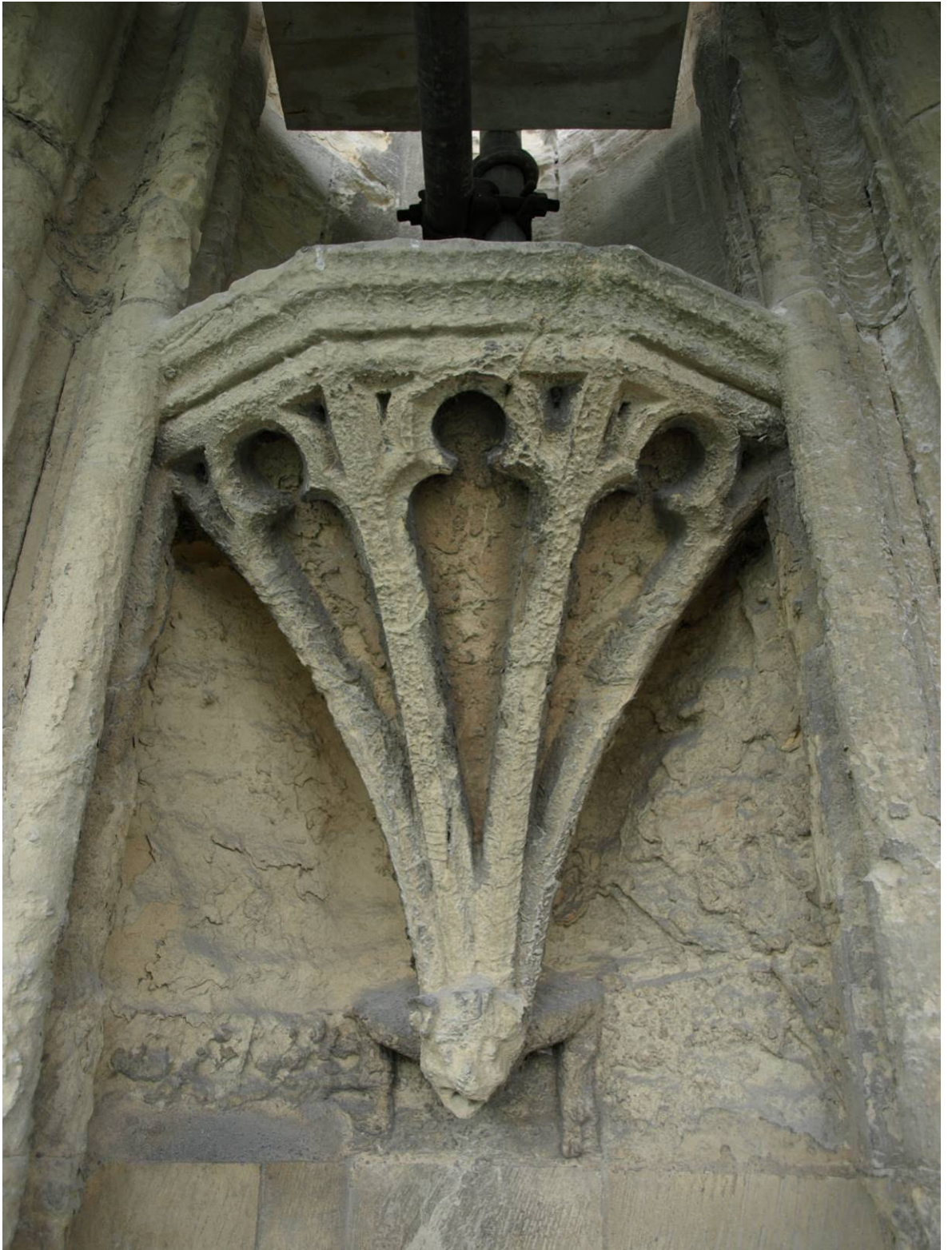
Figure 226: East Front, south-buttress nineteenth-century console detail, Level C
