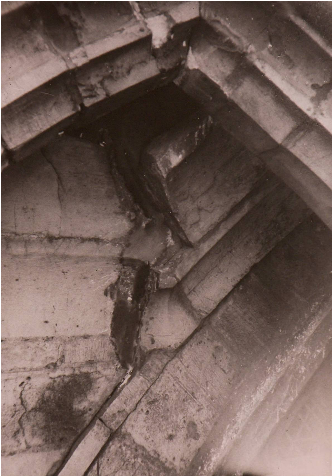
Figure 79: East end, bay 1 of the north clerestory, 1954 (YML/APYM/A71)
