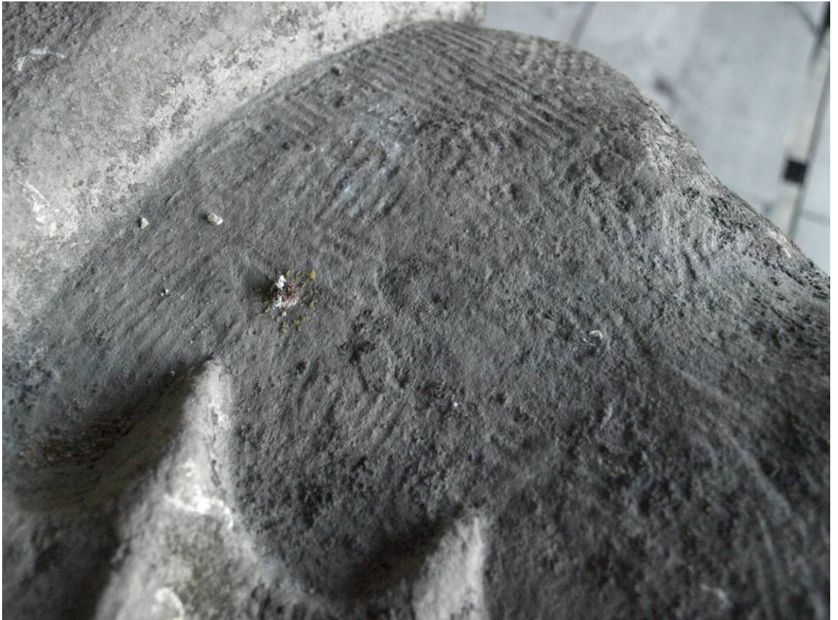
Figure 134: Twentieth-century claw tooling, 1970s
