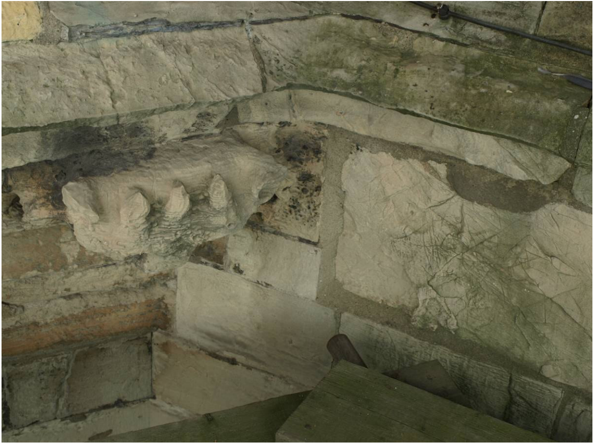
Figure 207: Junction between south-aisle cornice and south-east turret, Level B
