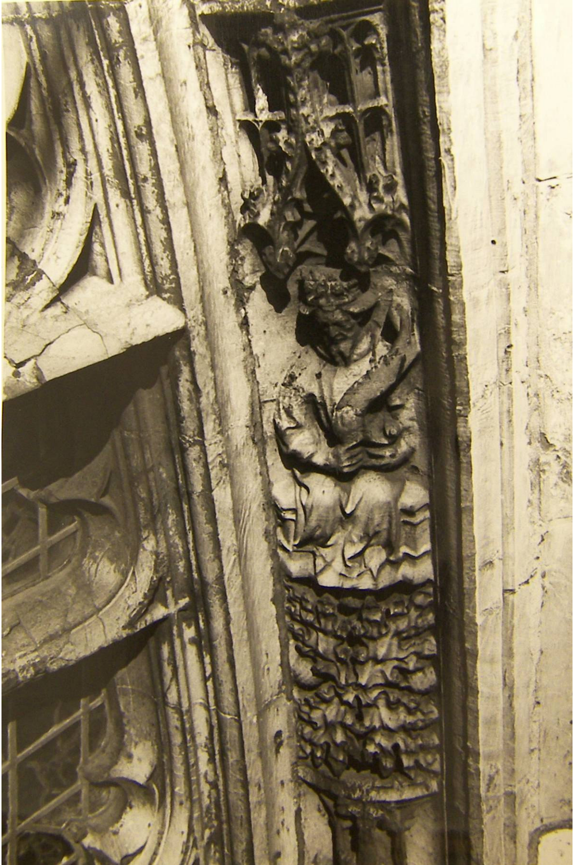
Figure 68: Great East Window exterior voussoirs, north side 1955 (YML/APYM/A57ii/14)
