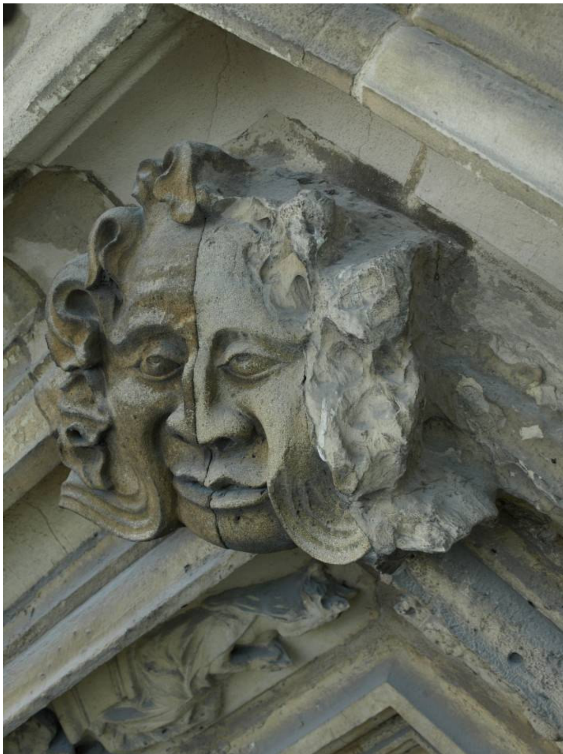
Figure 354: East Front, 'Green Man' keystone (b59) at apex of arch of Great East Window
