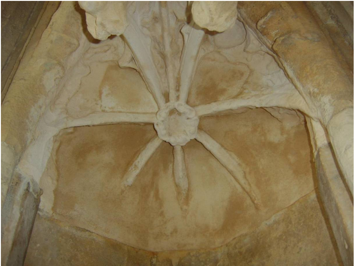
Figure 444: East Front, south-buttress canopy after conservation
