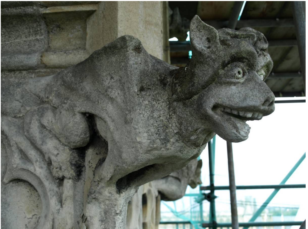
Figure 245: East Front, north-east turret nineteenth-century grotesque detail, Level D
