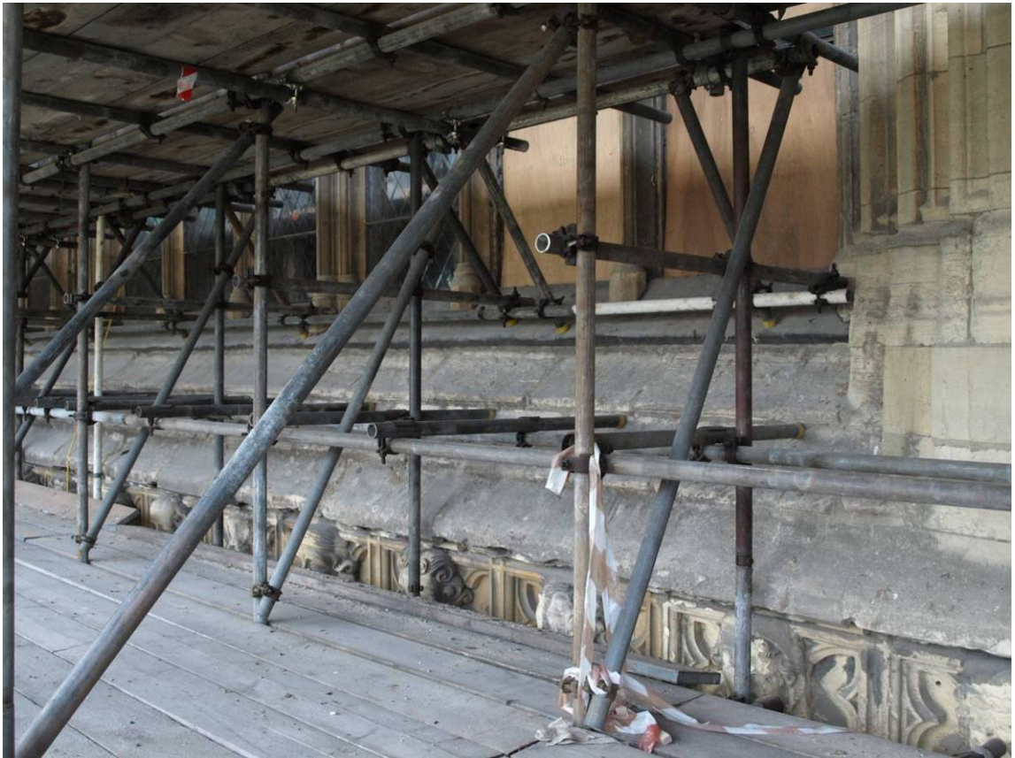
Figure 203: Great East Window sill, with carved heads beneath, Level A
