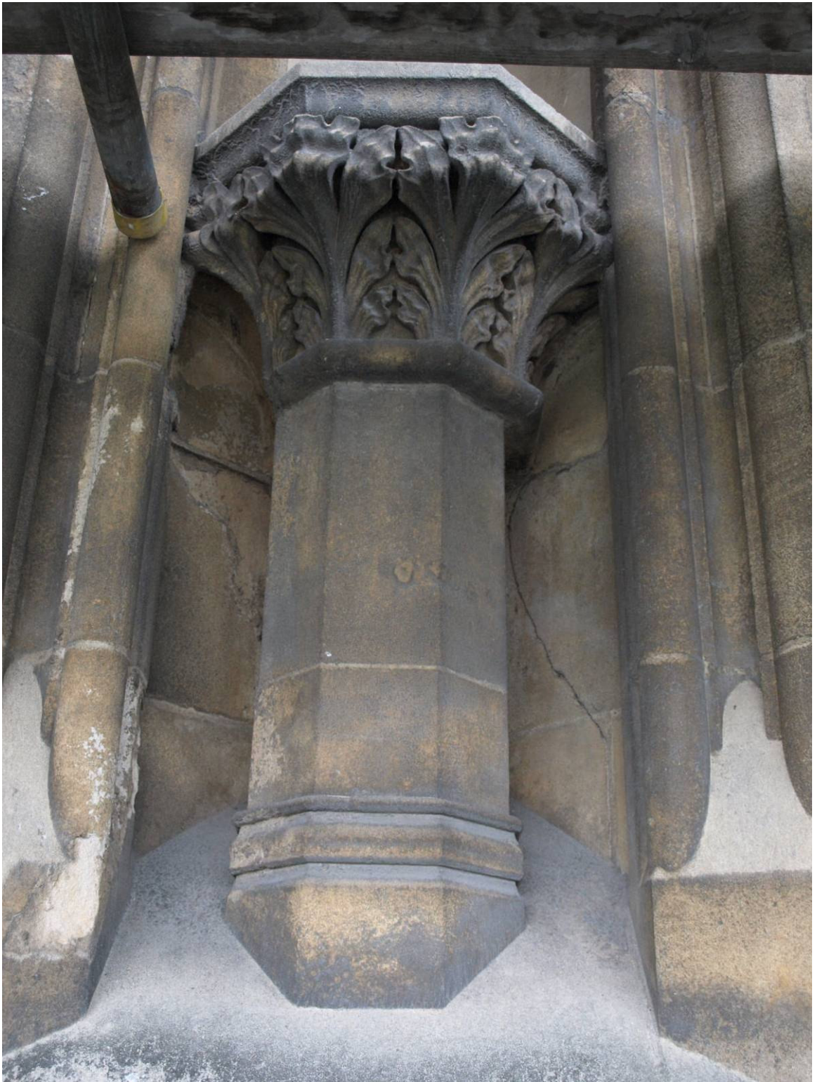
Figure 218: East Front, north buttress, New Ketton column detail, Level B
