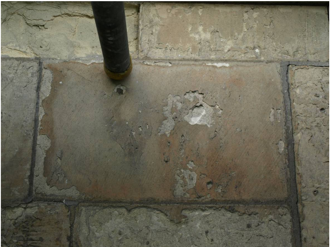
Figure 151: Masonry treated with limewash above south aisle window, easternmost bay of eastern arm
