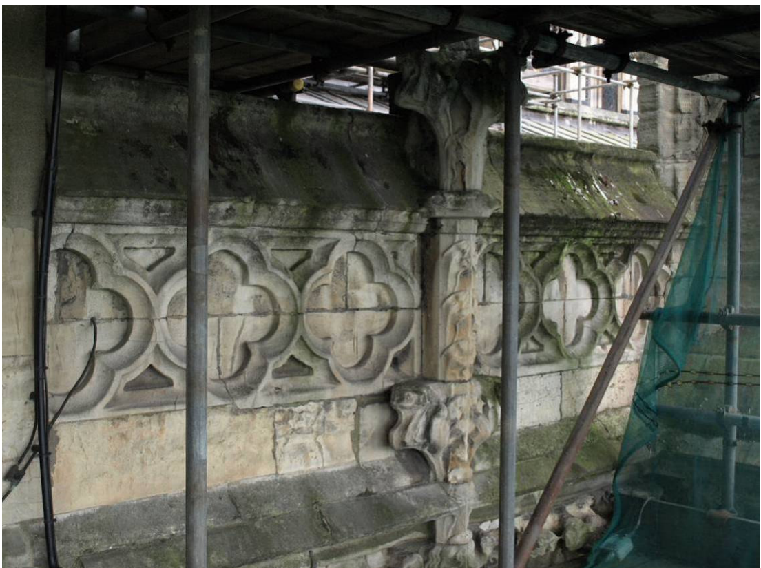
Figure 210: Easternmost bay, north-aisle parapet, Level B
