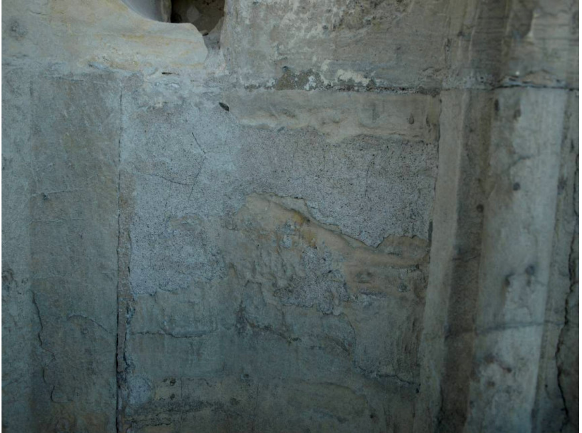
Figure 447: East Front, south buttress, historic lime-mortar repair
