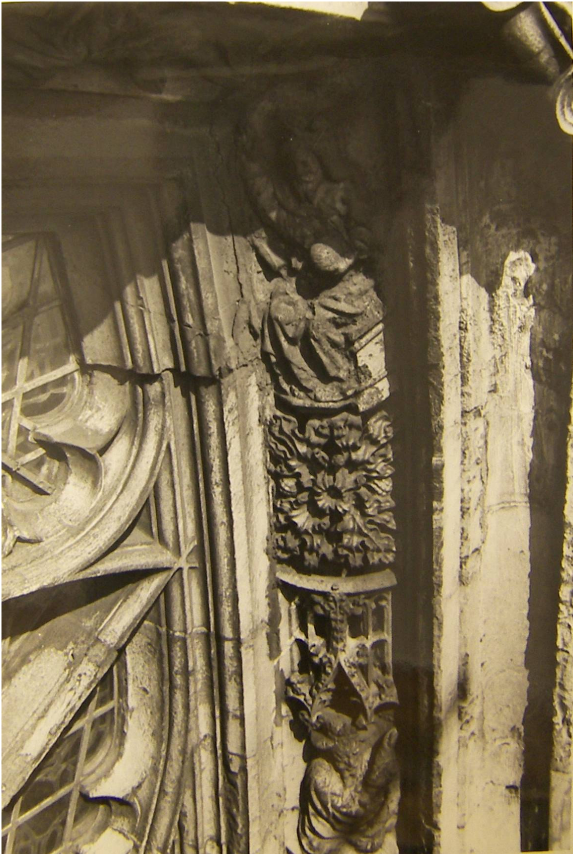
Figure 66: Great East Window exterior voussoirs, north side 1955 (YML/APYM/A57ii/14)
