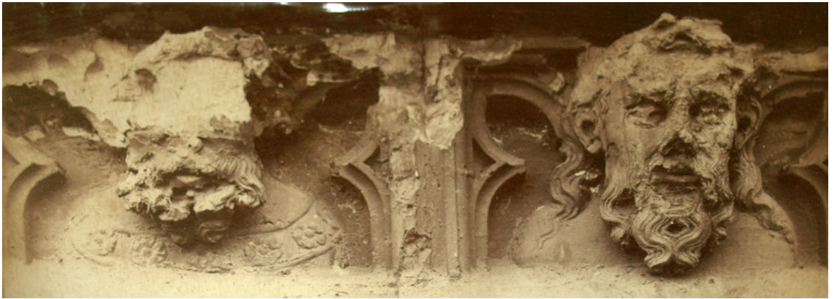
Figure 60: Sill carvings beneath Great East Window before renewals, Nos. 13-14 (YM Stoneyard)
