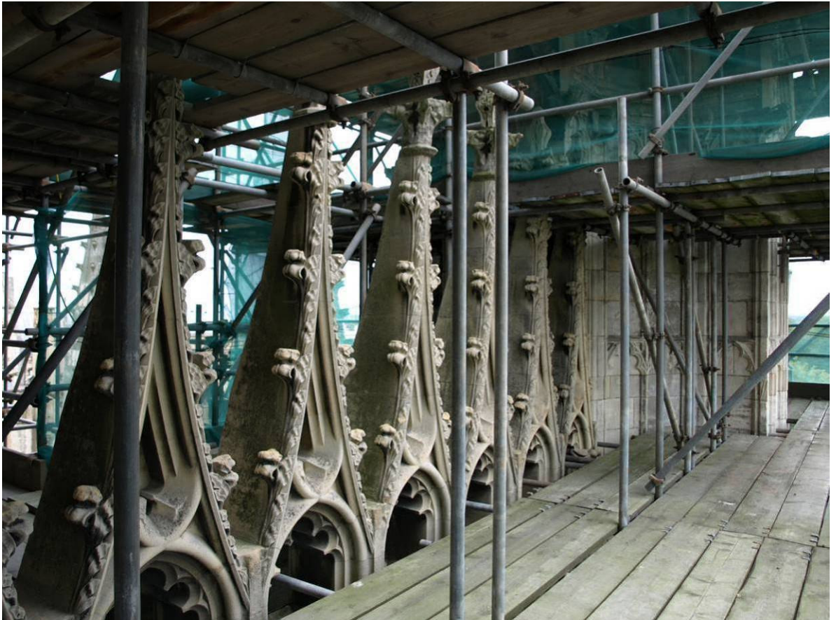
Figure 246: East Front, parapet gablets above north aisle, Level D
