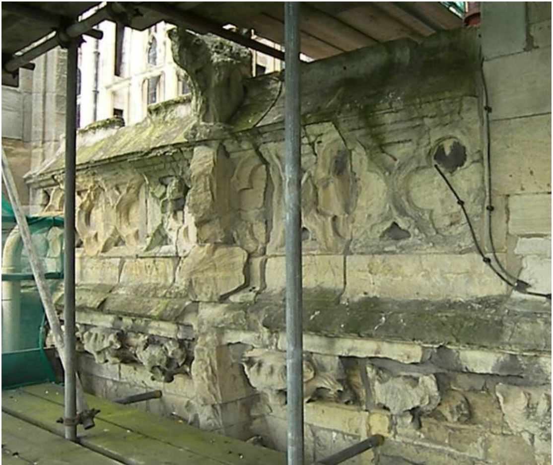
Figure 209: Easternmost bay, south-aisle parapet, Level B
