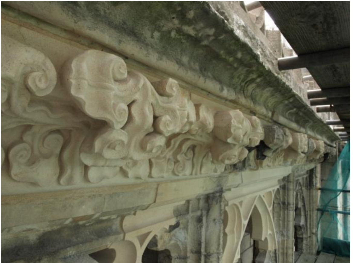
Figure 464: North-clerestory cornice bay 2 after renewal, 2008
