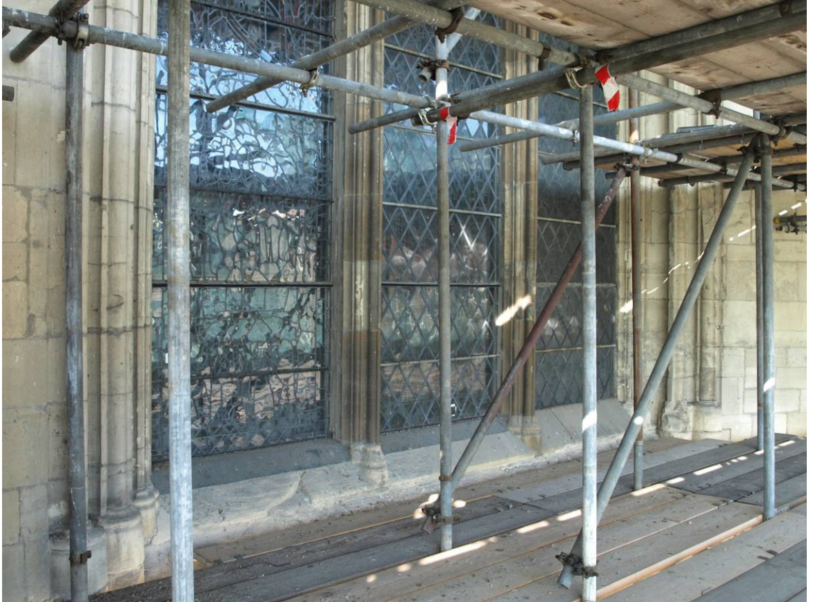
Figure 178: East Front, east window in north aisle, sill level, Level A
