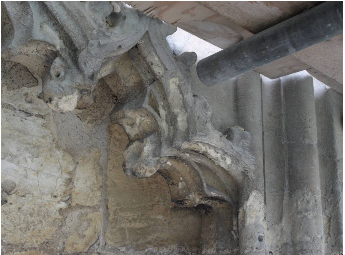
Figure 186: East Front, detail of canopy in south buttress showing previous surface repair and decaying carvings, Level A
