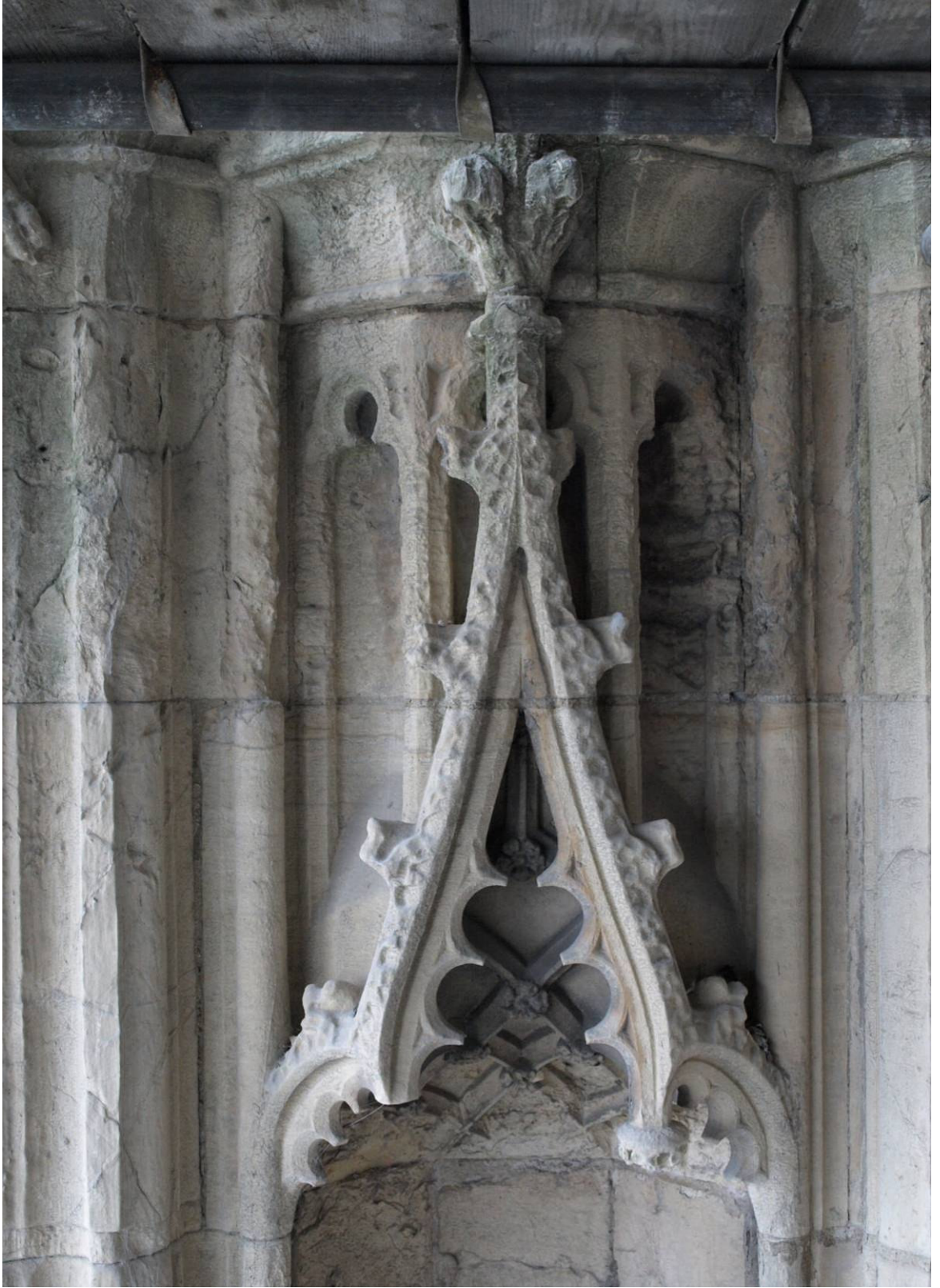
Figure 216: East Front, canopy in south buttress, Level B
