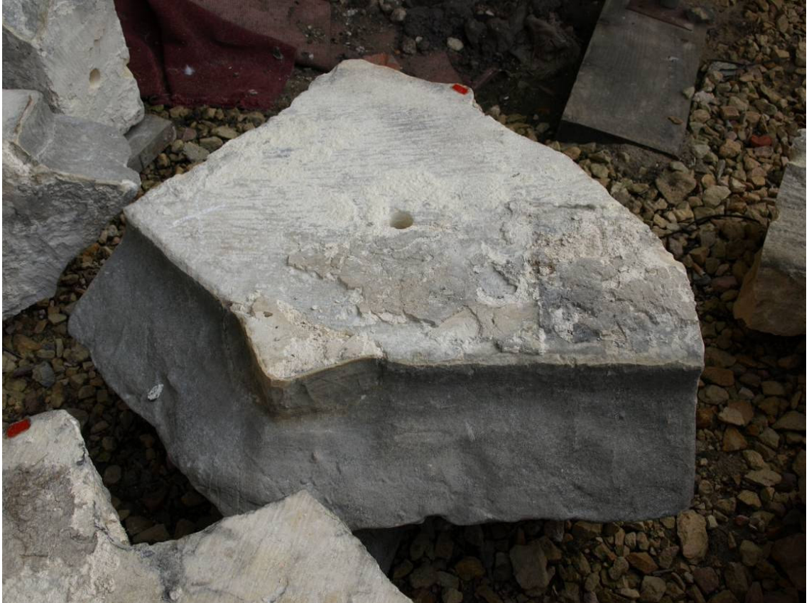
Figure 287: Removed stringcourse stone from beneath south-buttress corona, showing indented stooling
