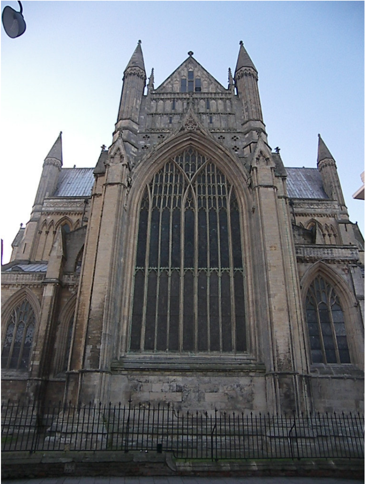
Figure 105: Beverley Minster, east end remodelled c.1416
