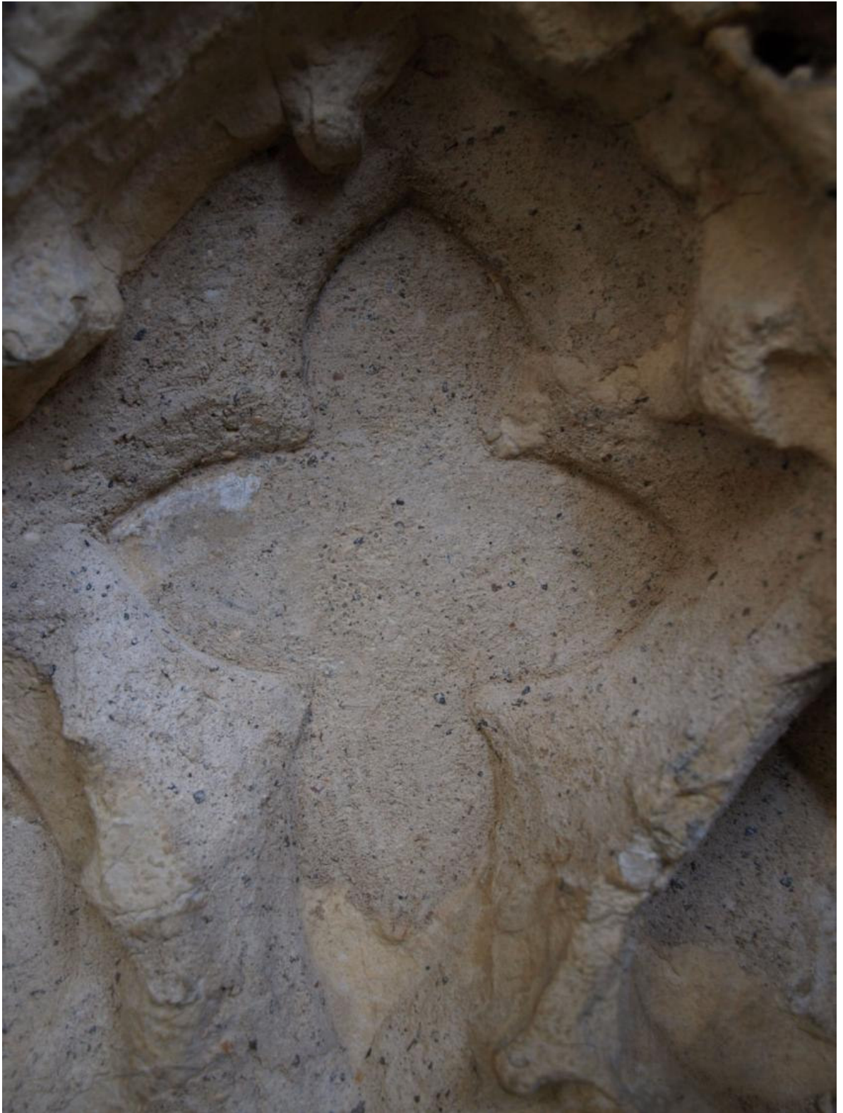
Figure 450: Howden Minster Chapter House, detail of trial conservation with coarse lime mortar
