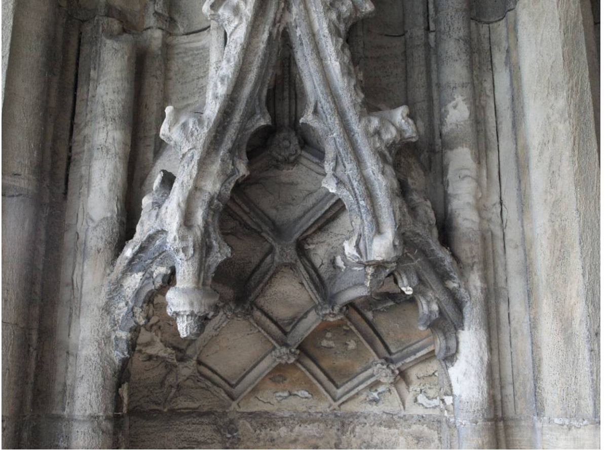
Figure 221: East Front, detail of canopy in north buttress, Level B
