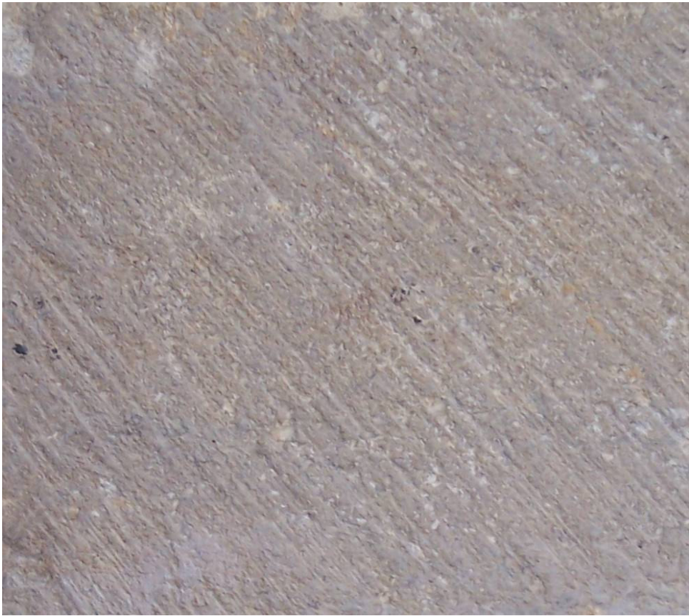
Figure 128: Diagonal plain axe on re-used twelfth-century ashlar in east end
