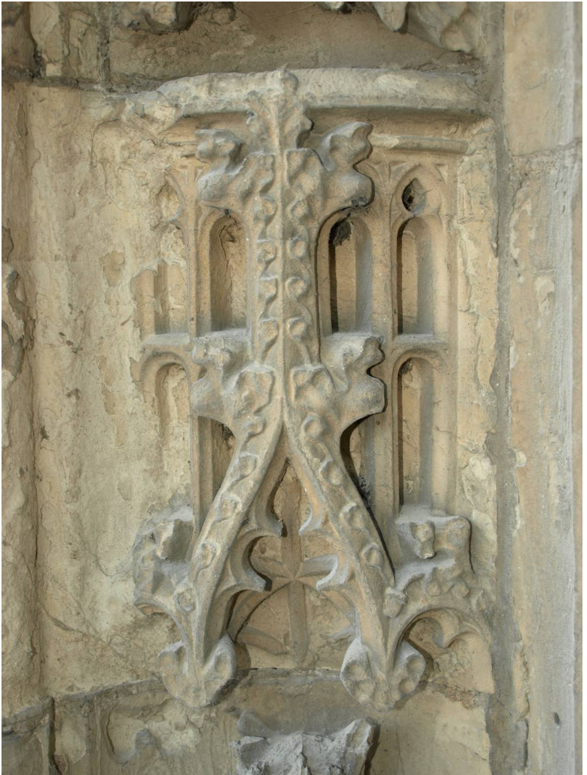
Figure 365: Voussoir b29, nineteenth-century replacement canopy
