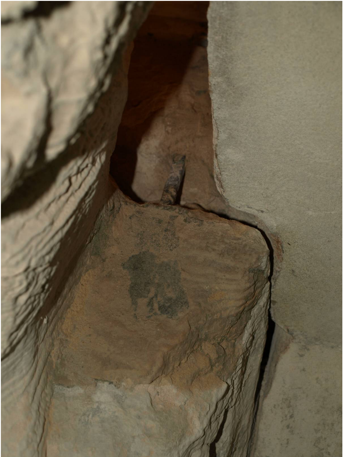
Figure 381: Seated figure, right-hand side of base showing exposed armature linking base with parapet
