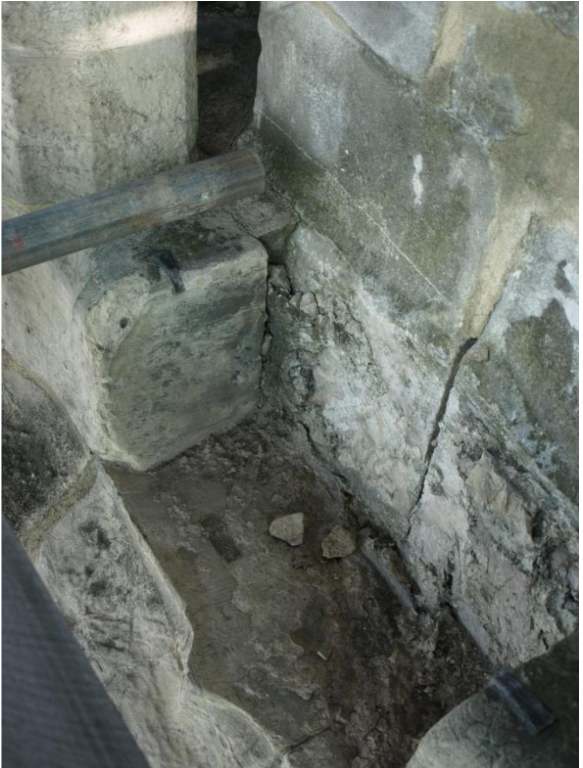
Figure 289: East Front, south buttress Level G/H, straight-joint between corona and broach
