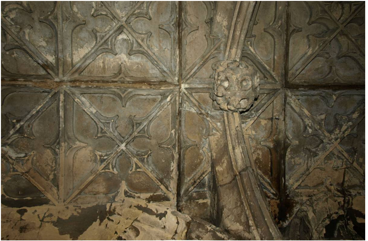
Figure 318: Great East Window interior, detail of underside of walkway (1820s)
