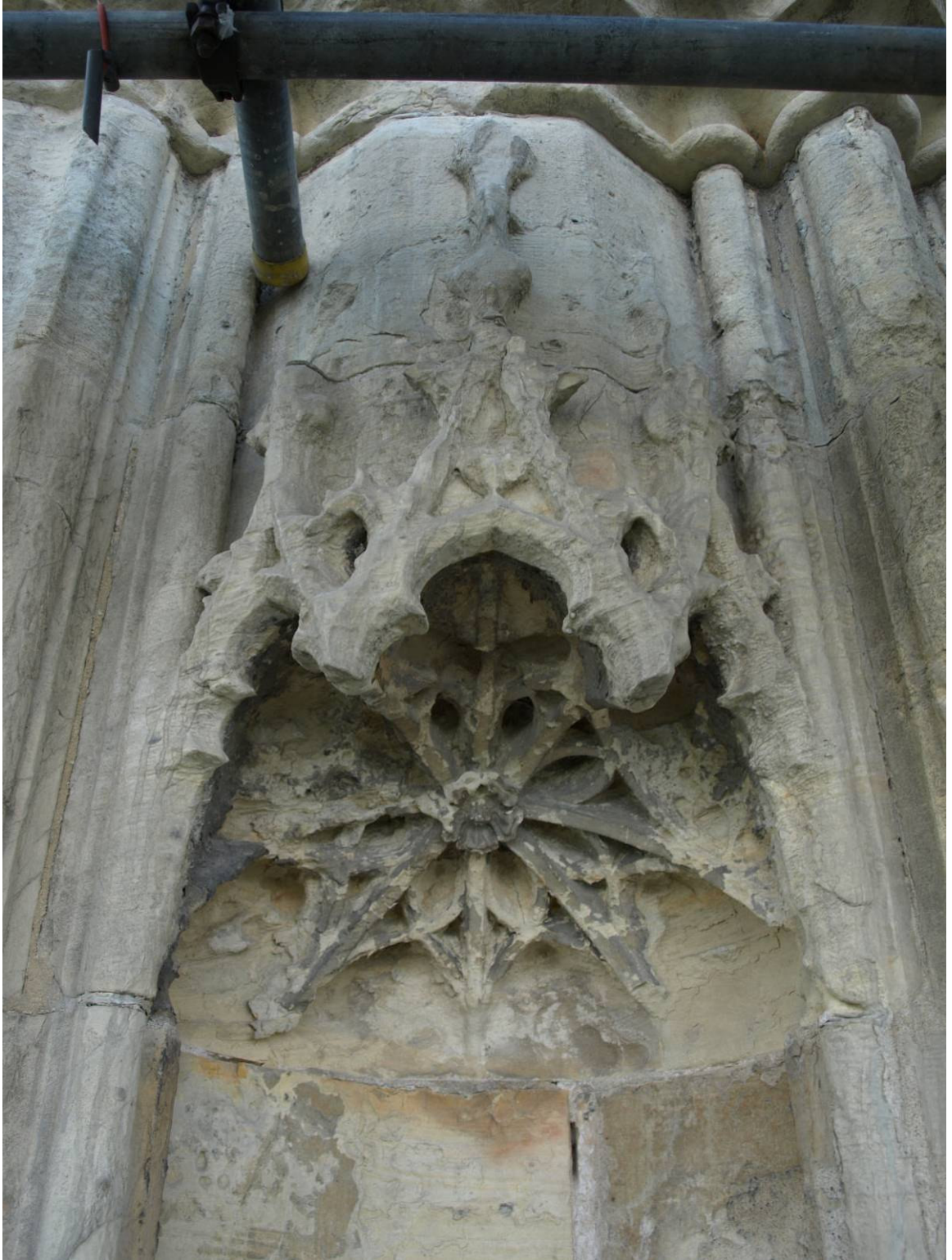
Figure 261: East Front, nineteenth-century canopy in south buttress, Level D
