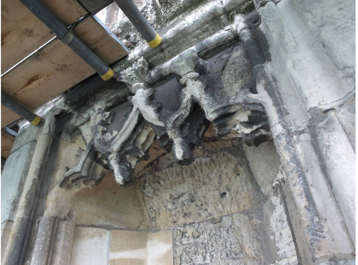
Figure 190: East Front, canopy in north-east turret, Level A
