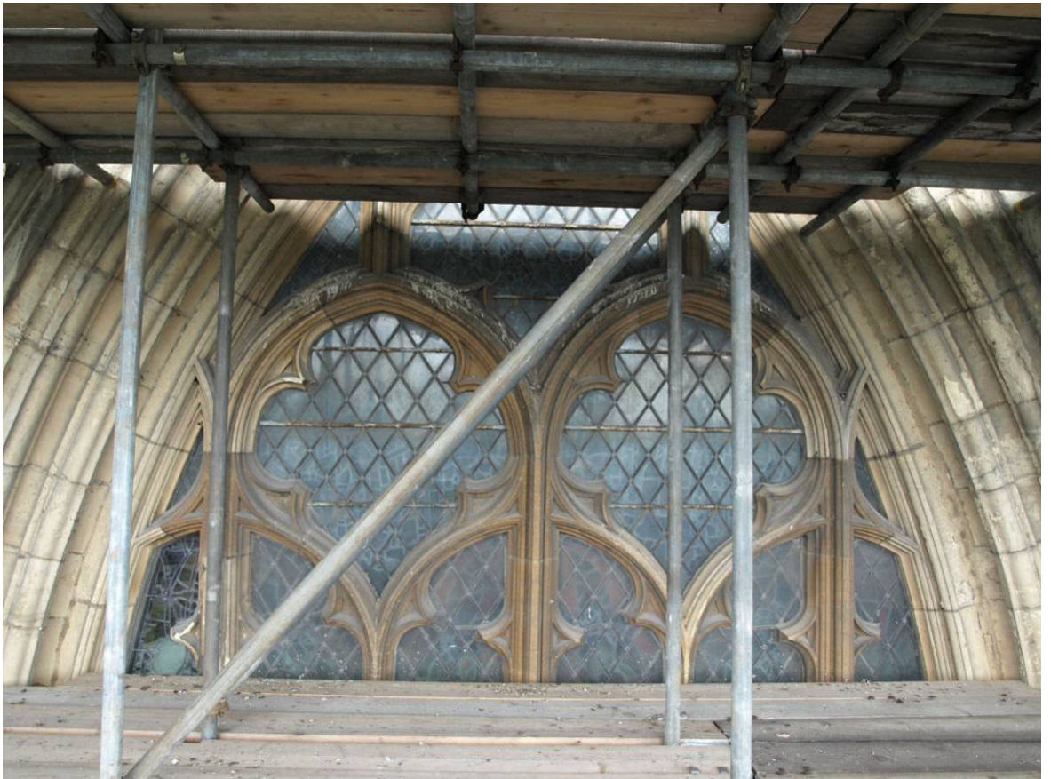
Figure 174: East Front, east window of north aisle, tracery, Level B
