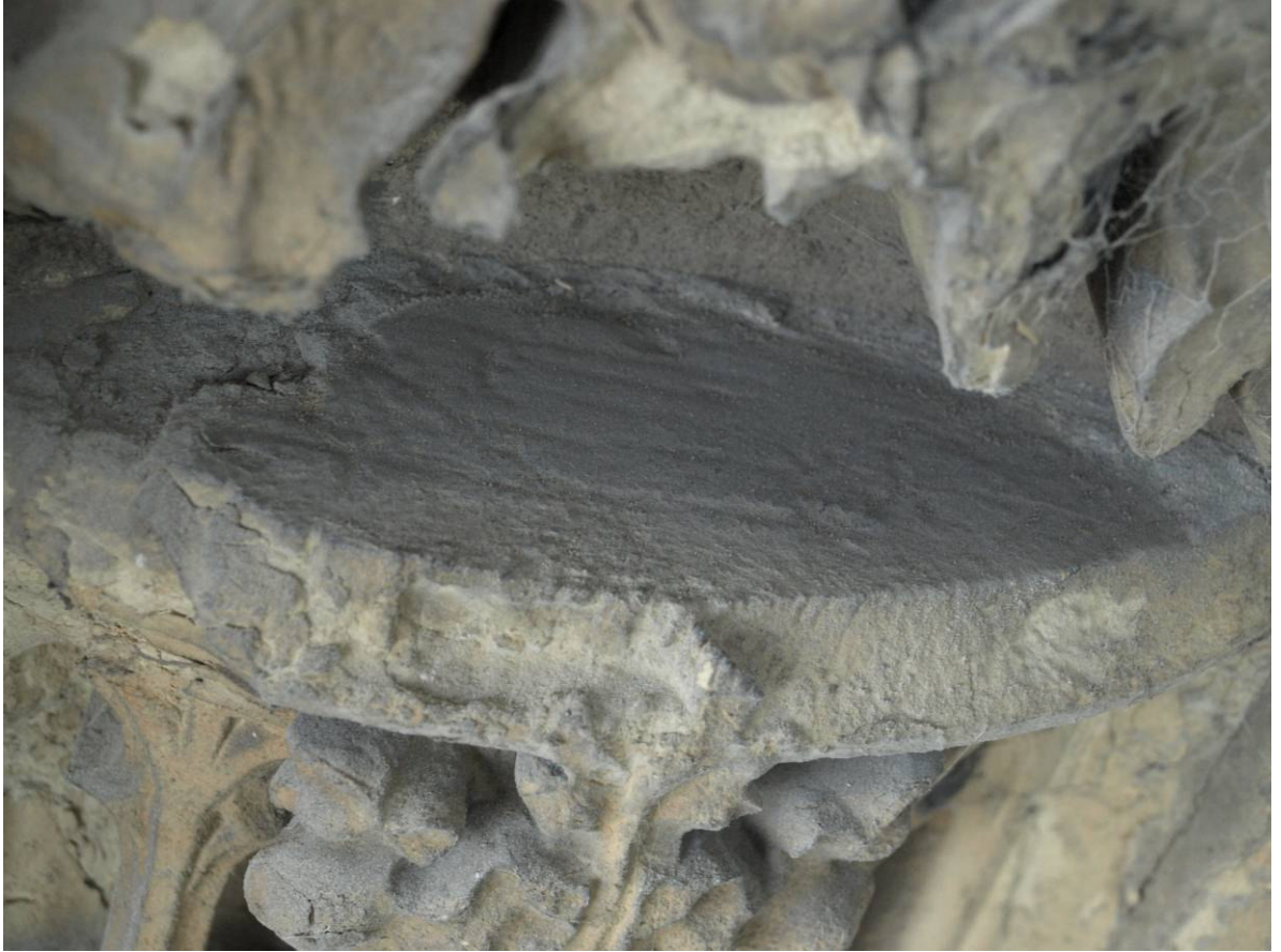
Figure 366: Example of replacement canopy showing lack of piercing and nineteenth-century tooling
