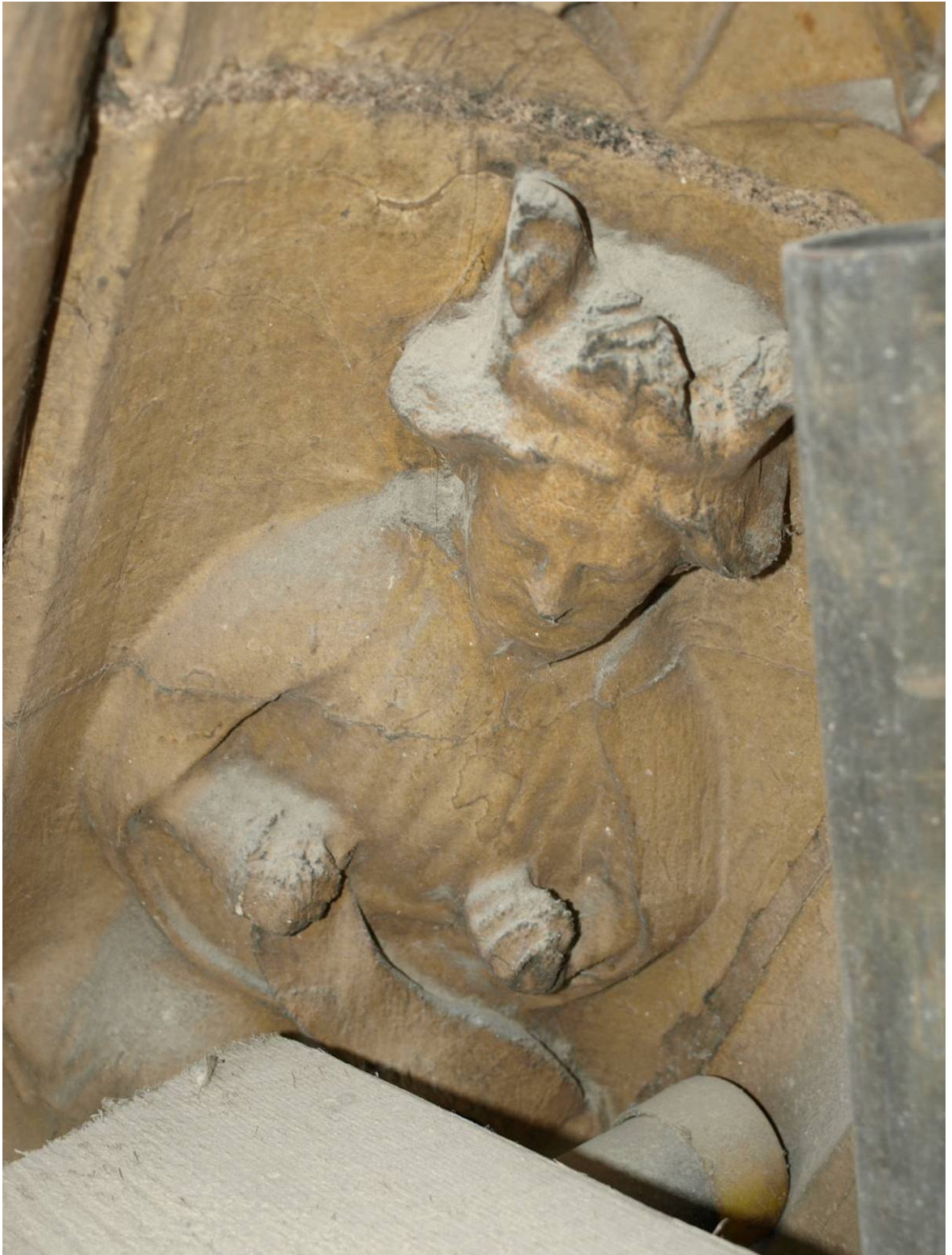
Figure 367: Voussoir b39, showing typical brown staining indicative of previous treatments with linseed oil
