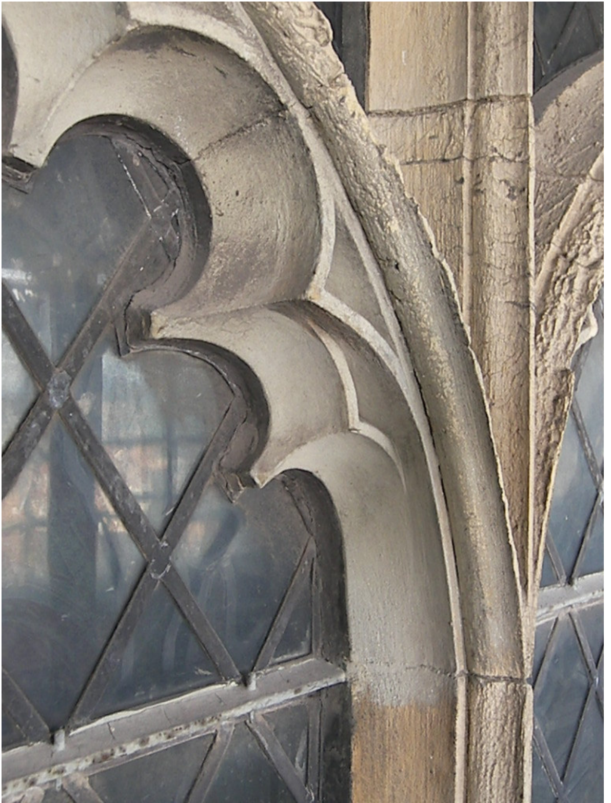
Figure 436: Great East Window exterior, mullions and transom masonry before cleaning trials
