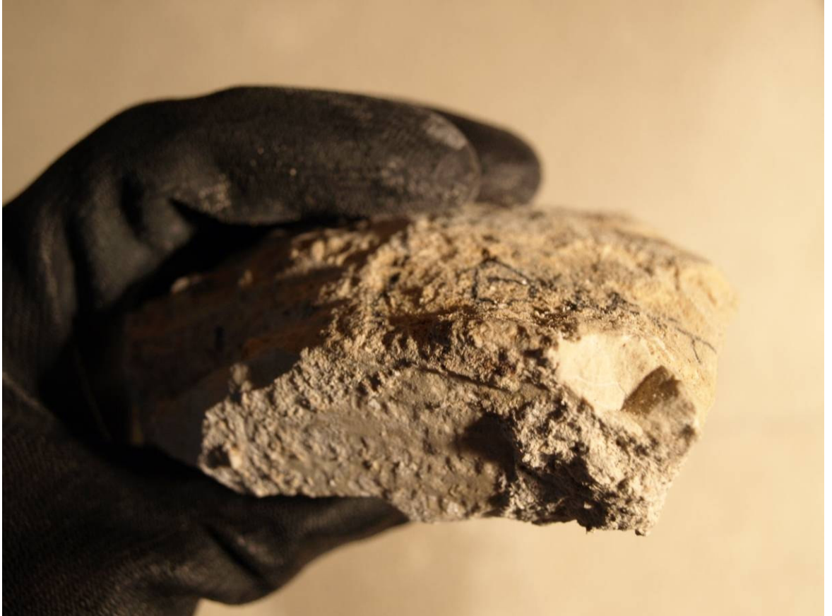
Figure 390: Fragment from rear of upper section showing claw tooling on bottom bed
