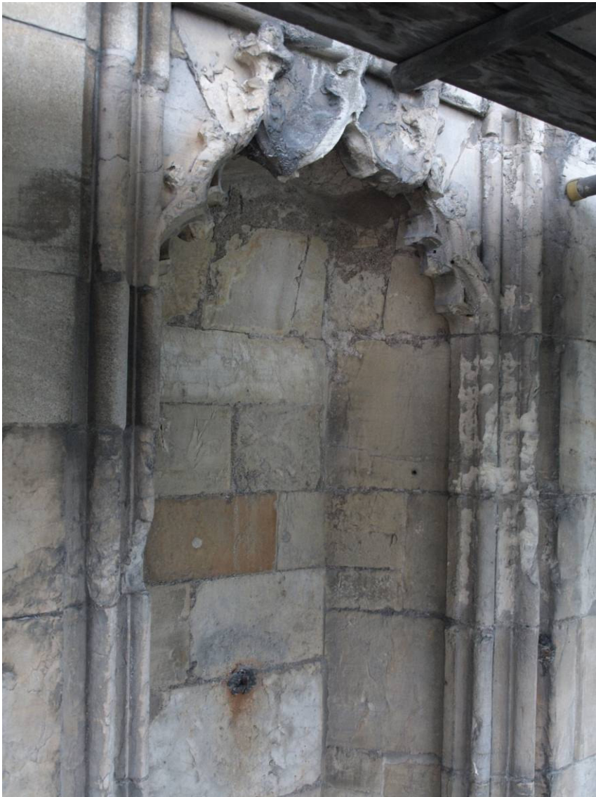
Figure 183: East Front, south turret niche, Level A
