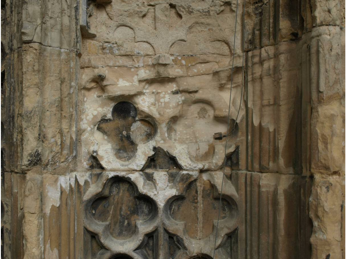
Figure 451: Howden Minster Chapter House, enhanced salt development adjacent to magnesium-lime pointing, June 2010
