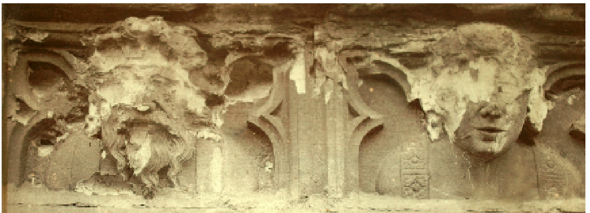
Figure 56: Sill carvings beneath Great East Window before renewals, Nos. 5-6 (YM Stoneyard)
