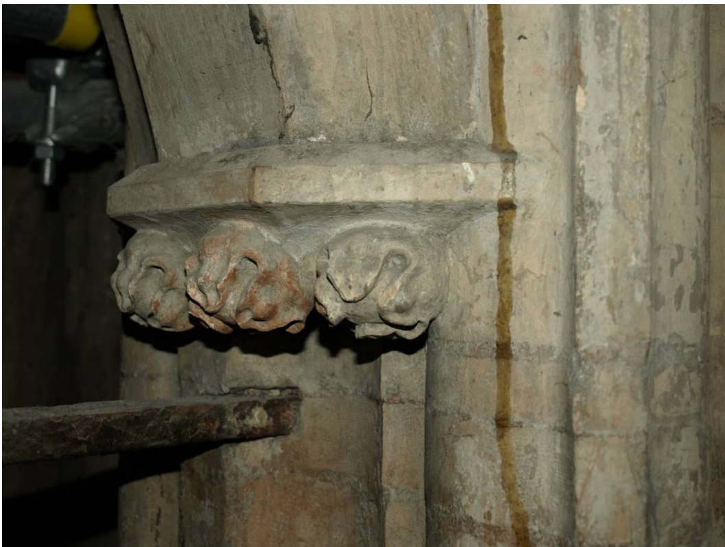
Figure 332: Great East Window interior, detail showing relationship between inner screenwork and iron reinforcement and window aperture, upper transom/walkway south side (screenwork masonry is 1820s work)
