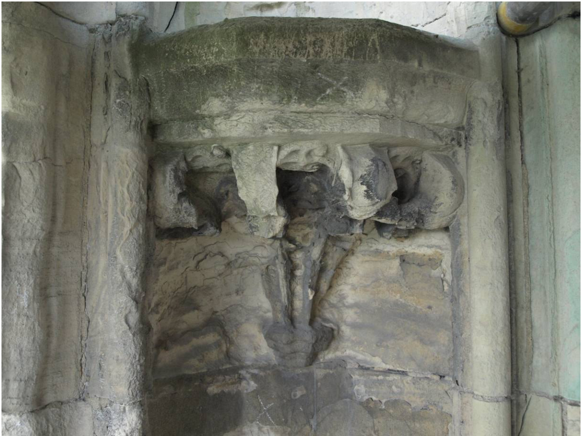
Figure 258: East Front, nineteenth-century niche-pedestal in north buttress, Level D
