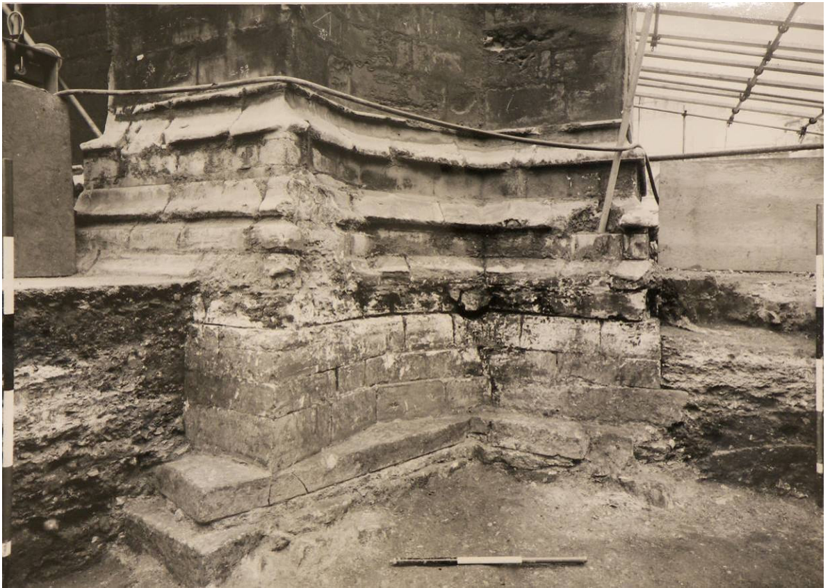
Figure 158: Foundations of north-east turret, East Front, 1968 (YML/YMEX1968/YM889)
