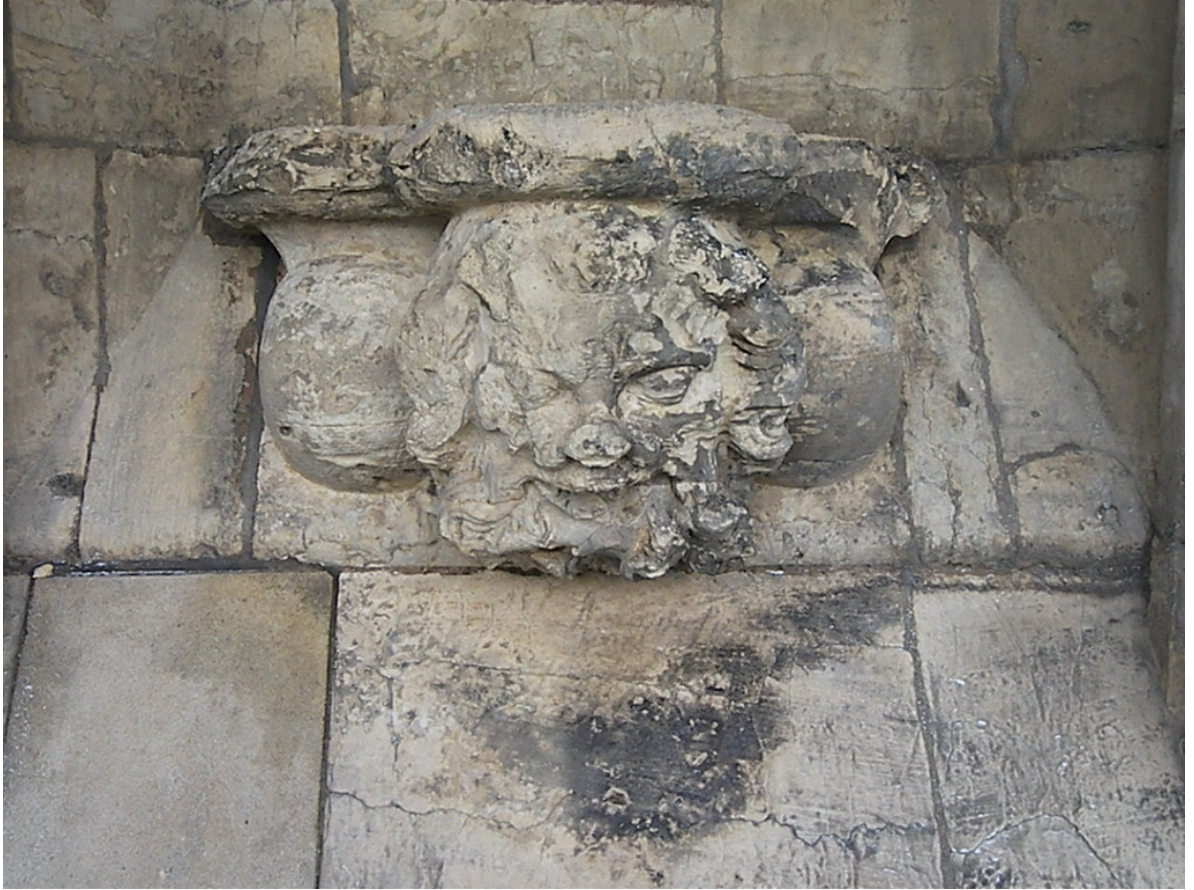
Figure 435: East Front, niche-base after cleaning trials (right-hand side left untreated)
