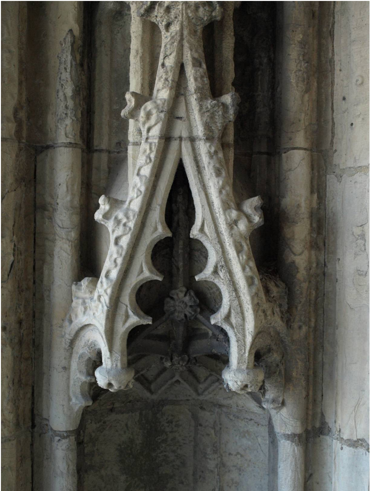
Figure 229: East Front, niche-canopy detail in south buttress, Level C
