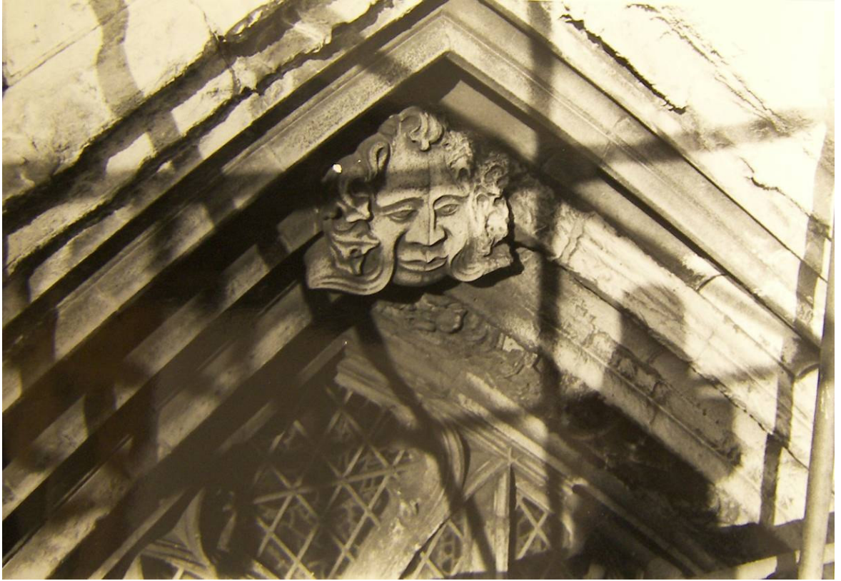
Figure 70: Great East Window exterior voussoirs, apex 1955 (YML/APYM/A57ii/14)
