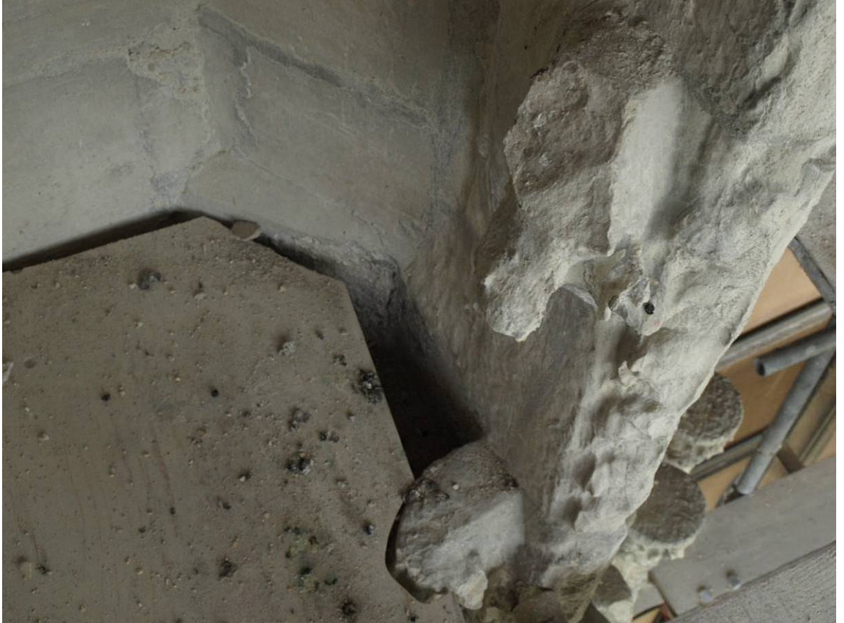
Figure 339: East Front, Great East Window exterior, off-set punched masonry, south side of arch
