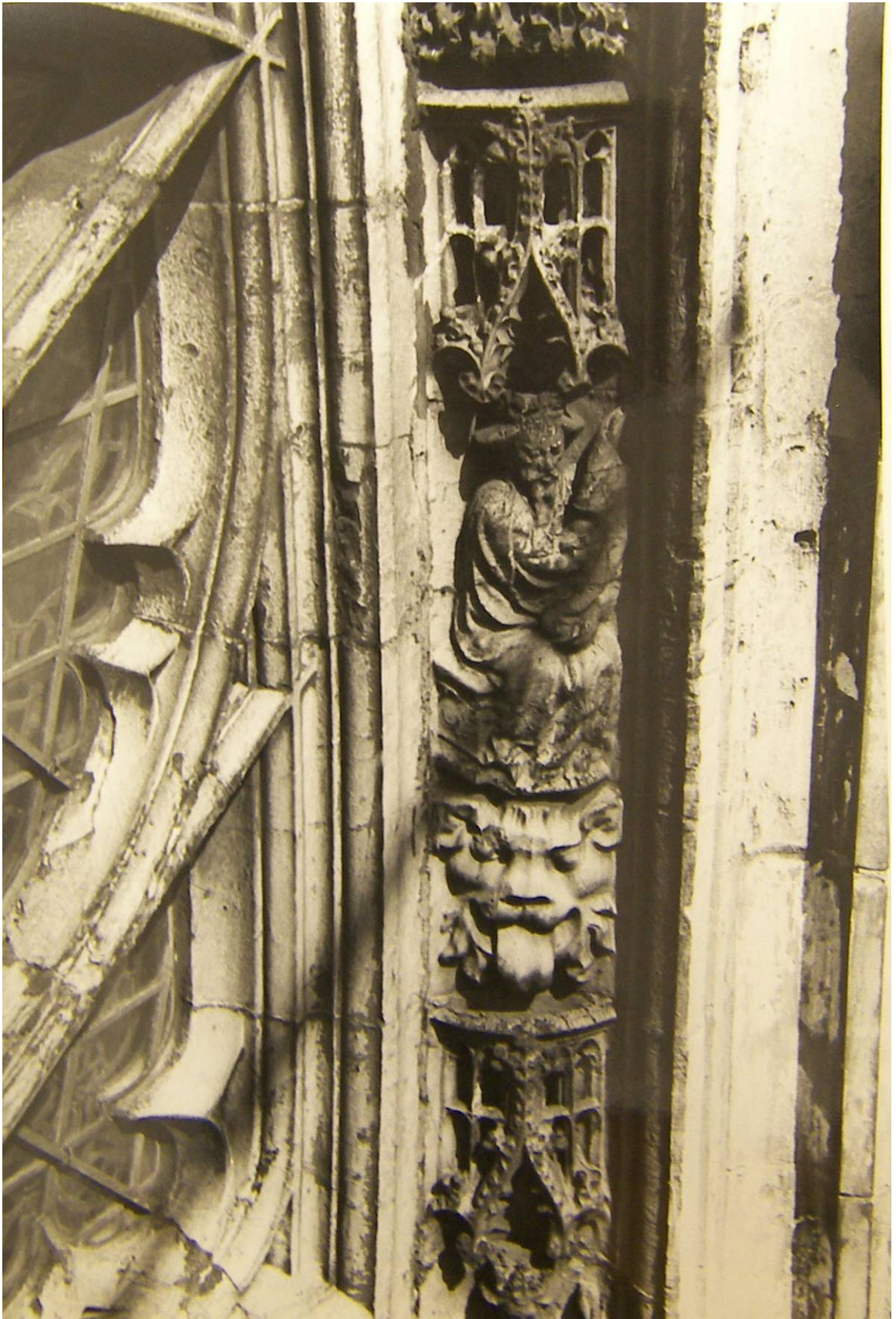
Figure 65: Great East Window exterior voussoirs, north side 1955 (YML/APYM/A57ii/14)
