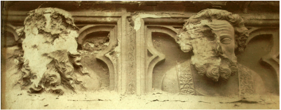
Figure 57: Sill carvings beneath Great East Window before renewals, Nos. 7-8 (YM Stoneyard)
