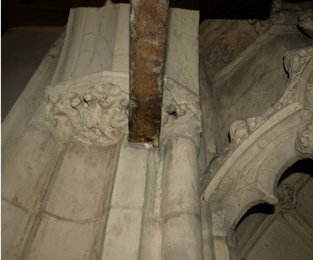
Figure 329: Great East Window interior, detail showing relationship between inner screenwork and iron reinforcement and window aperture, lower transom north side
