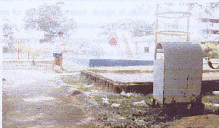
c. Lack of maintenance of rubbish bins in park.
