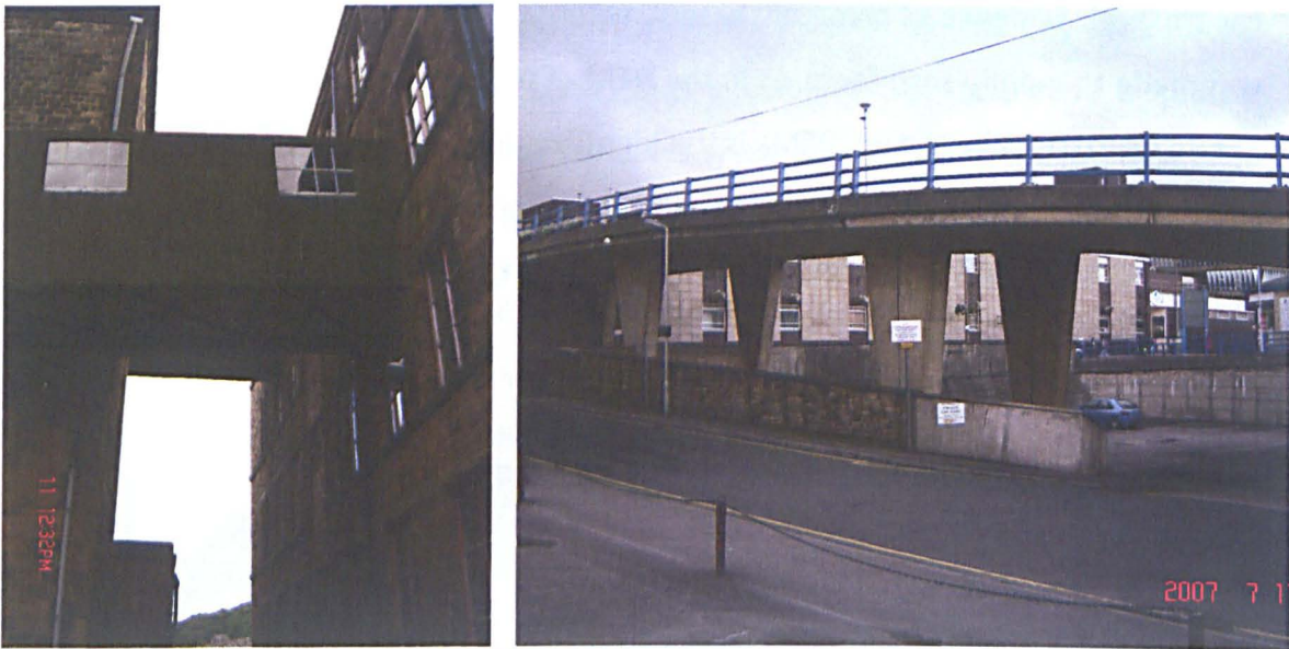
Figure 2.5: Elevated structures that in LiDAR DEMs are represented as barriers to water movement downstream.
