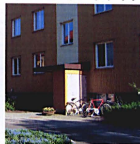
H) Shared facilities for storage of outdoor furniture and play equipment.
