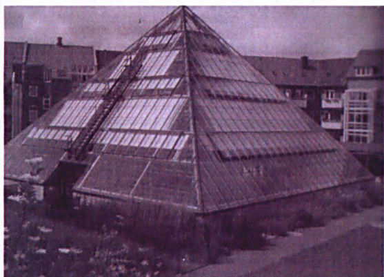
Figure 1.4 Sewage has been entirely treated through an effective but complicated series of basins, plants, and reed beds in this pyramid as part of the regeneration for the Hollandervej Fredensgade block (image from Ian Bentley, Green Urbanism: Learning from European Cities , 2000, p. 250)
