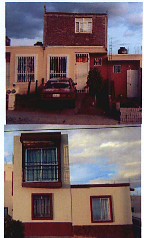
Fig. 1.9 Above: Low income housing of Villas de la Loma Morelia, Mex. extended on the top by traditional local techniques. Bottom: Comparative of two low- income housing modified in different ways giving little individuality to the owners. Villas de la Loma, Morelia, Mex.
