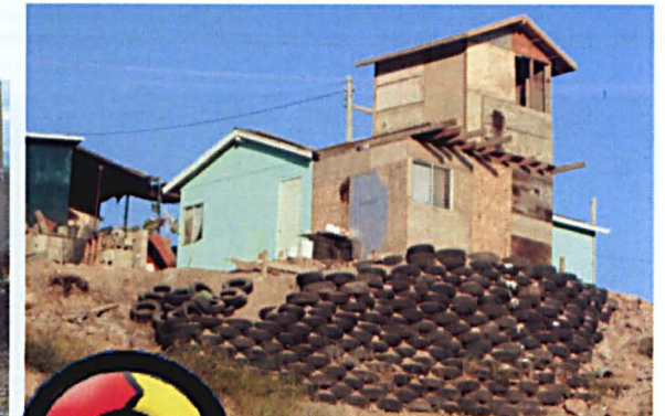
Tyres used as a container wall
