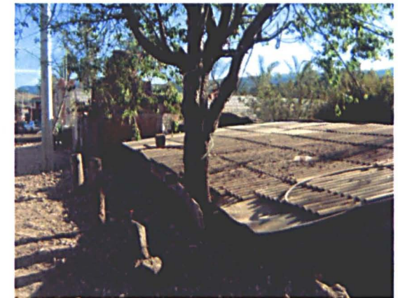
Fig. 3.2 Traditional housing literally considered as obstacle to the new road. As a result of the new levels of the paving street which does not acknowledge natural topographic level, it was almost covered. It is located in the vernacular town of Jesus Del Monte already a suburban area of Morelia Mex, next to the brand new development Bosques de Altozano.
