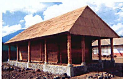
Wood Troje with stone foundations
