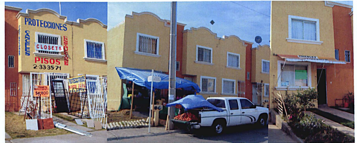
Front housing doors and windows protections workshop
