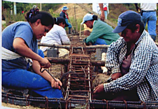
Family enabling the steel foundations
