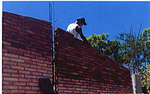
Member of the family developing a brick wall
