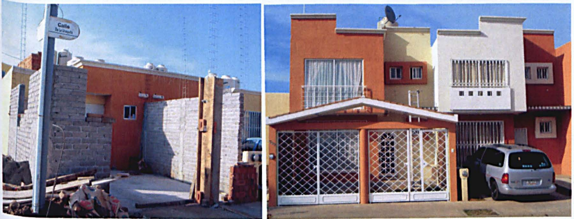
Basic Housing suffering an extension in the front
