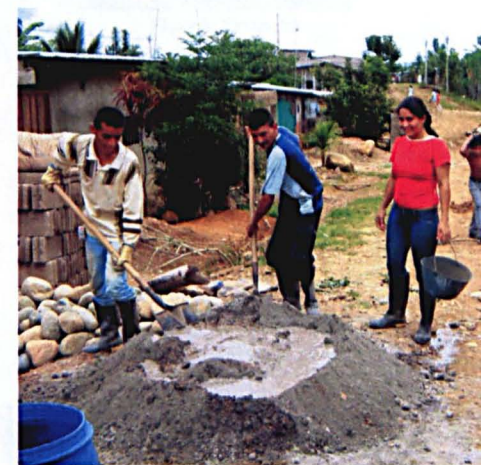
Members of the family preparing concrete for the roof.
