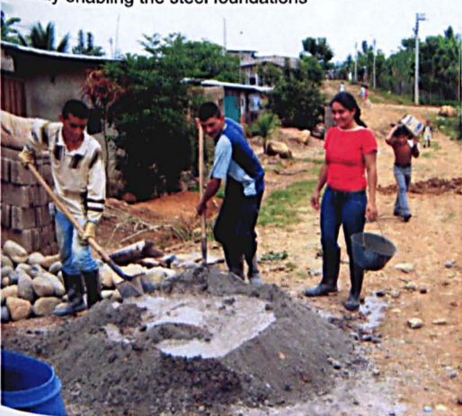
Members of the family preparing concrete for the roof.
