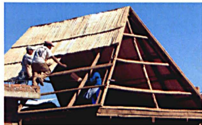
Construction of troje's roof
