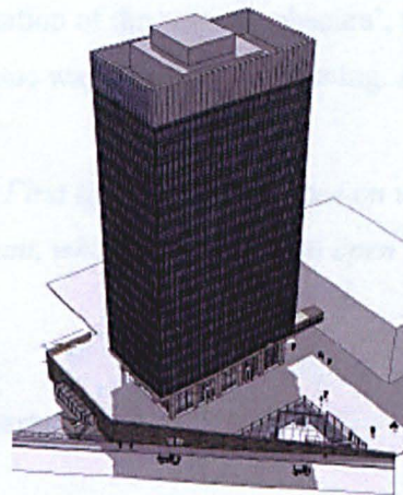
[Figure 6-4] Computer graphic image of the Arts Tower exterior.
