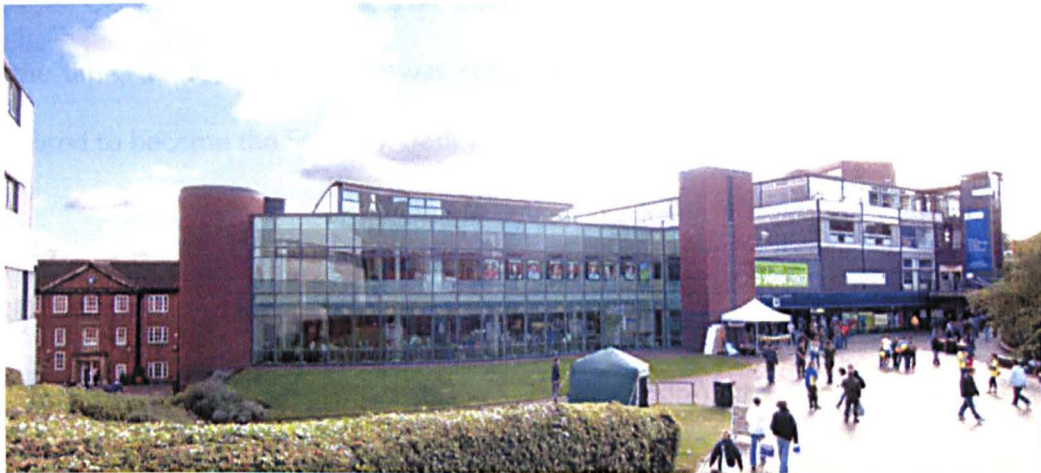
Figure 3.01 Main façade of the Student's Union. From left to right: white/grey building is part of Hicks Building (not part of the Students' Union); former Graves Building (3 storeys and pitched roof); new link (3 storeys, upper 2 storeys, both curtain glazed, visible) incorporating the atrium and related spaces; main entrance (1 storey visible); University House (4 storeys visible). Source: author's photograph
