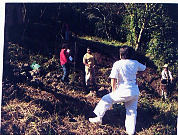
Photo 8.6: UCISV-Ver member supervising construction work on plot (Melanie Lombard)
