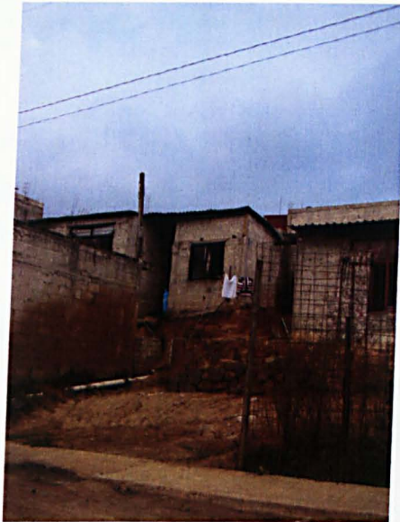
Photo 8.4: Construction shored up by earth and stones in Moctezuma (Melanie Lombard)
