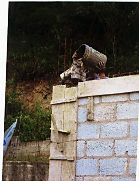
Photo 8.3: UCISV-Ver contractor using basic construction techniques (Melanie Lombard)
