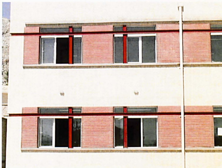
Fig 6.25. The main façade and classroom windows, Photo © F. Ai
