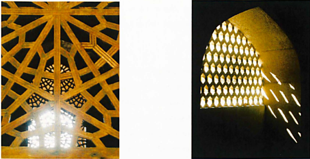
Fig 2.10. Examples of geometric latticed screens as filtering solutions of harsh sunlight, Khan School, Shiraz, Iran, (Photos © F. Ai)
