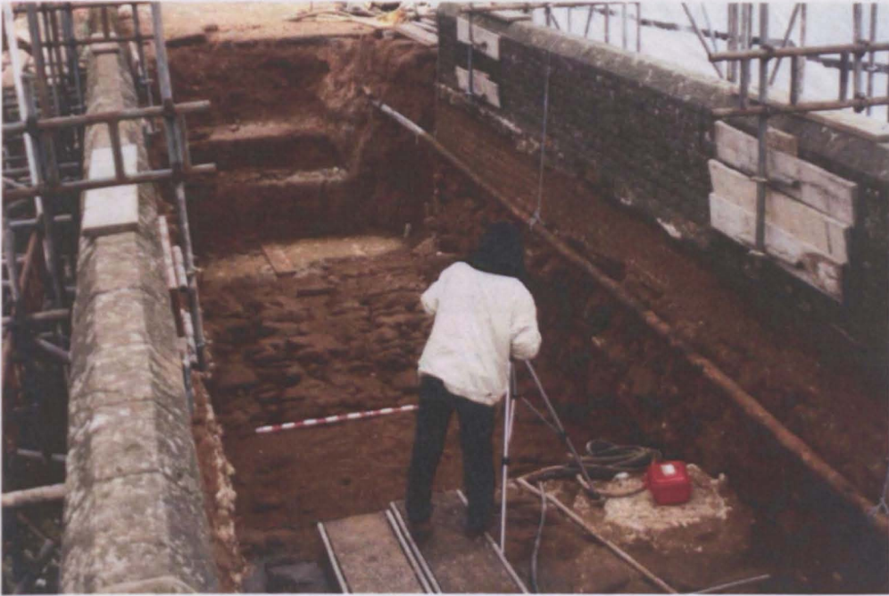
FIGURE 2.2: Strengthening Woolbeding Bridge (Mabon 2002)
