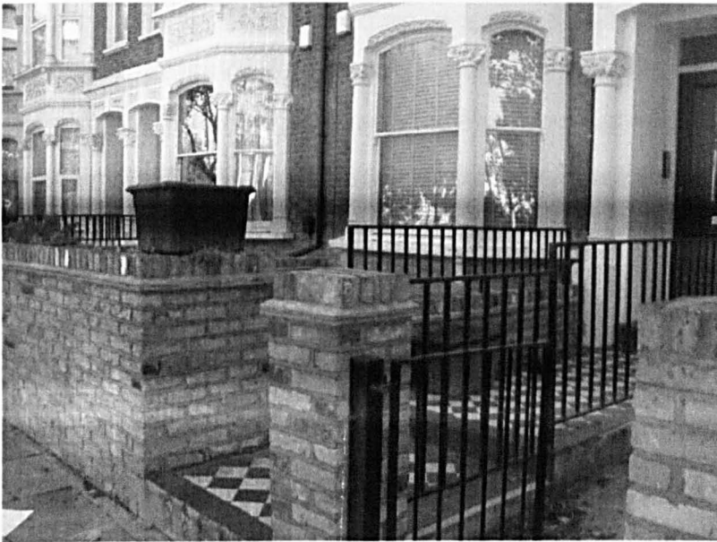
Image 20 – Front gardens give way to private new access to refurbished basement flats
