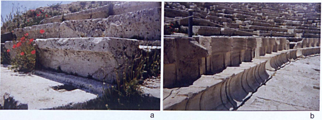
Figure 3.3.3. Detail of the seating system at the theatre of Dionysus. a) Archons' seats and b) Typical seats.
